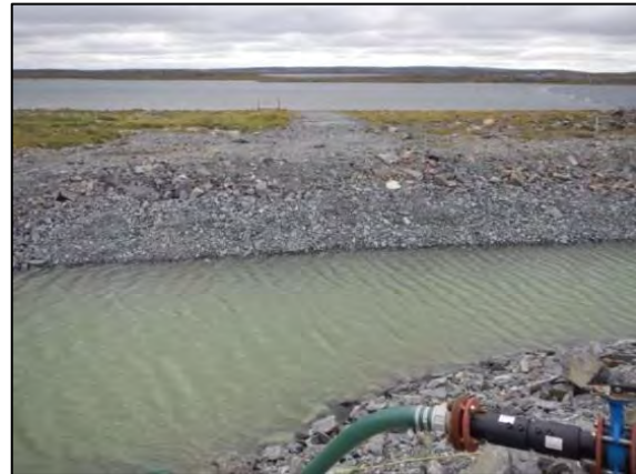
Photo 32: Trench below Assay Laboratory to prevent water from entering lake
