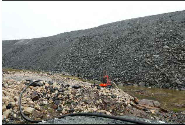
Photo 30: Ongoing monitoring of seepage from the Portage waste rock storage facility
