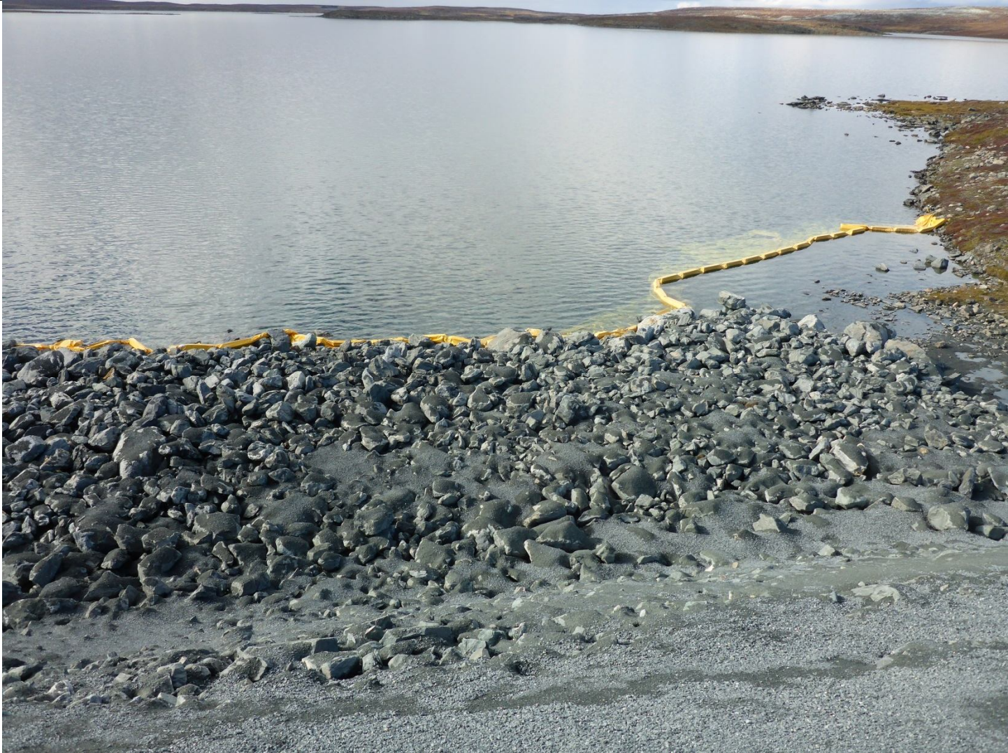
Description: Sediment booms installed at the Northwest end of the runway.
