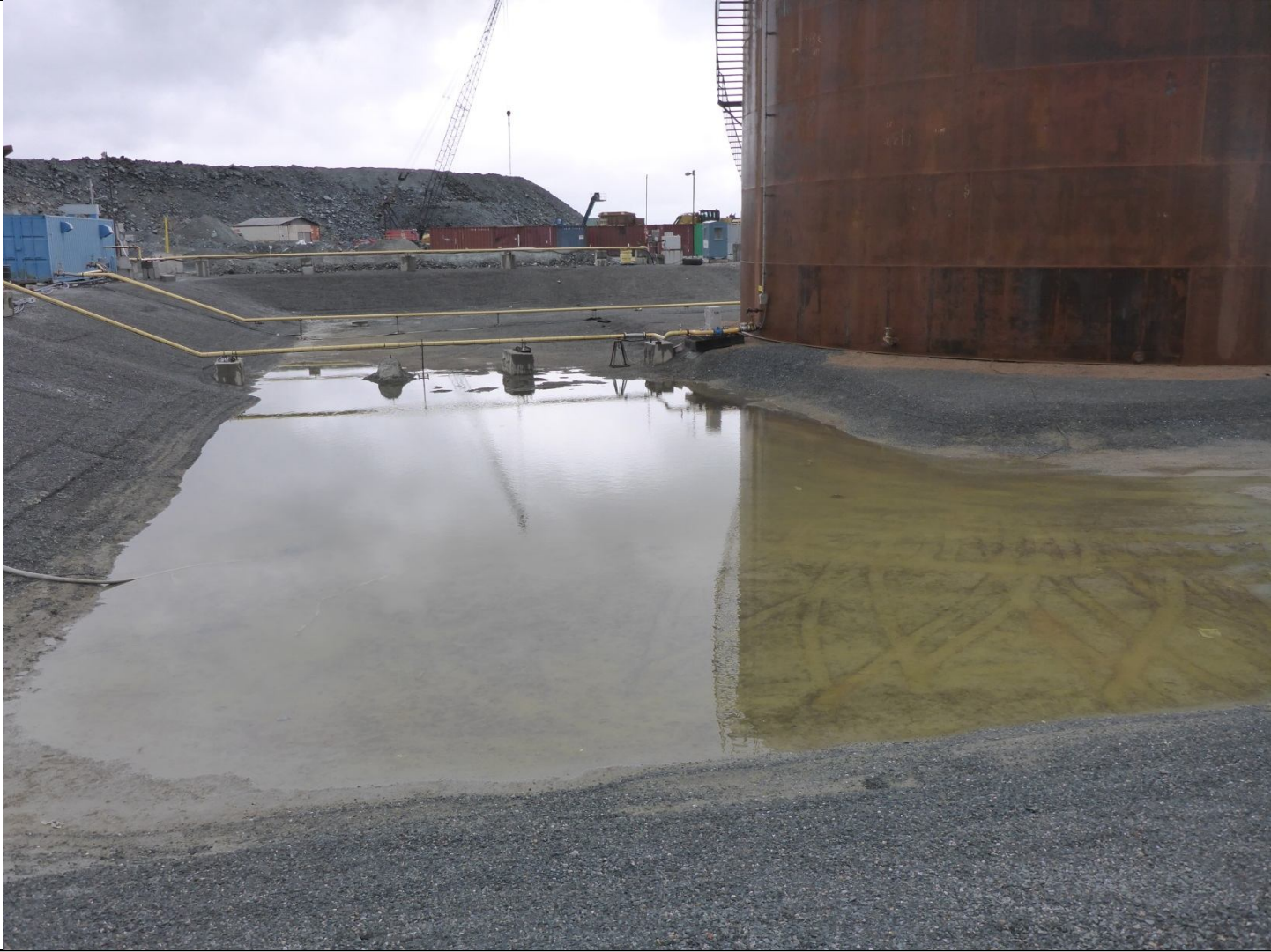
Description: Minimal water within the main tank farm berm.
