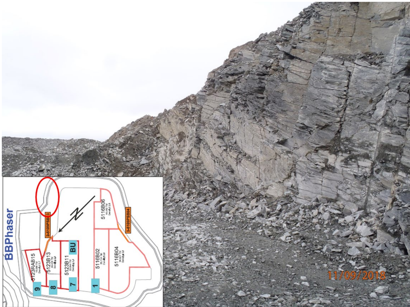
Photograph 8-21: BB Phaser Pit east to north end wall showing continuous orthogonal joint surfaces
