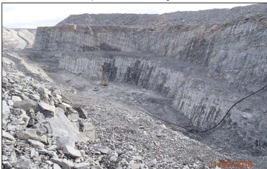
Photograph 8-14: Phaser Pit east-southeast highwall performance (2018)
