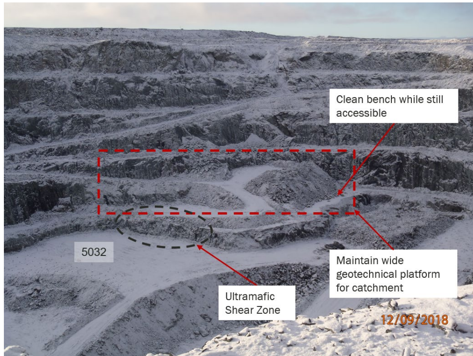
Photograph 6-9: Pit E5 5032 mRL platform and ultramafic shear zone
