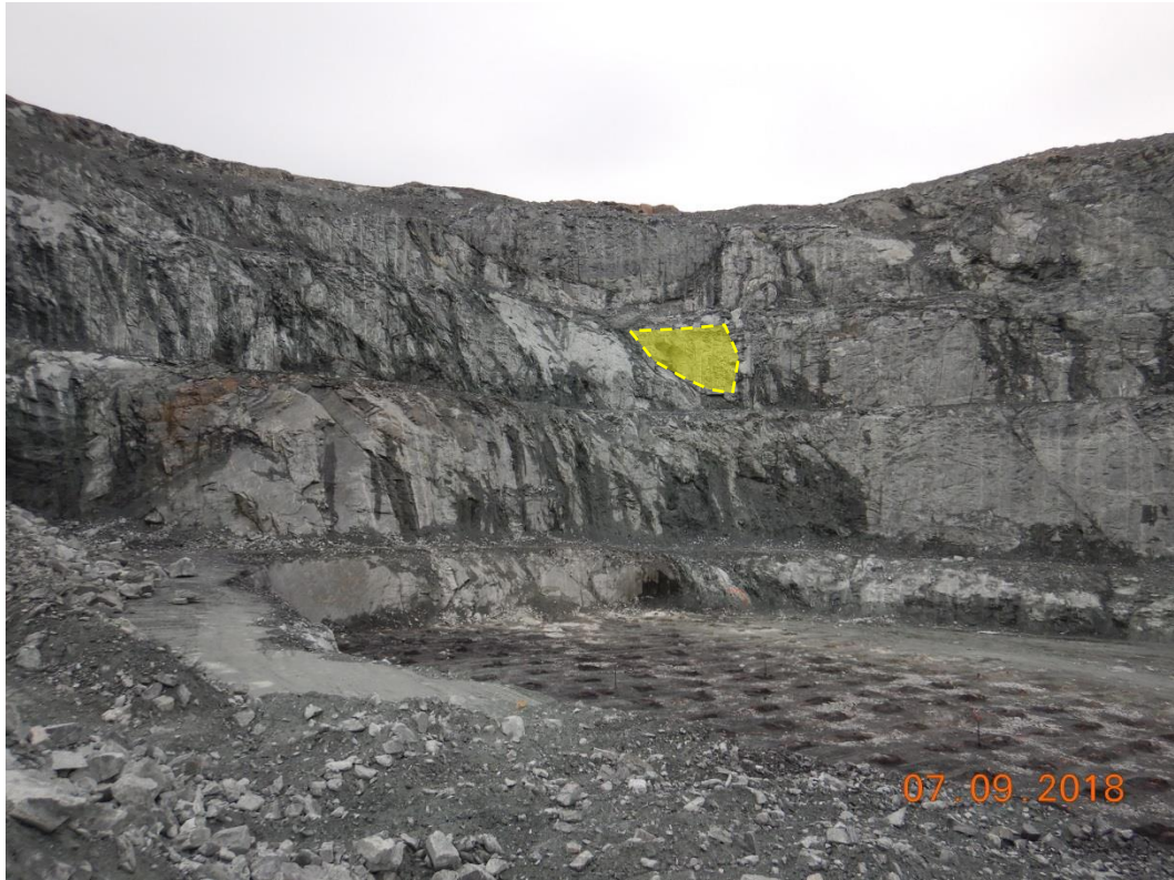
Zone E29: Pit E5, South Wall: Slab with linear progression to be monitored.
