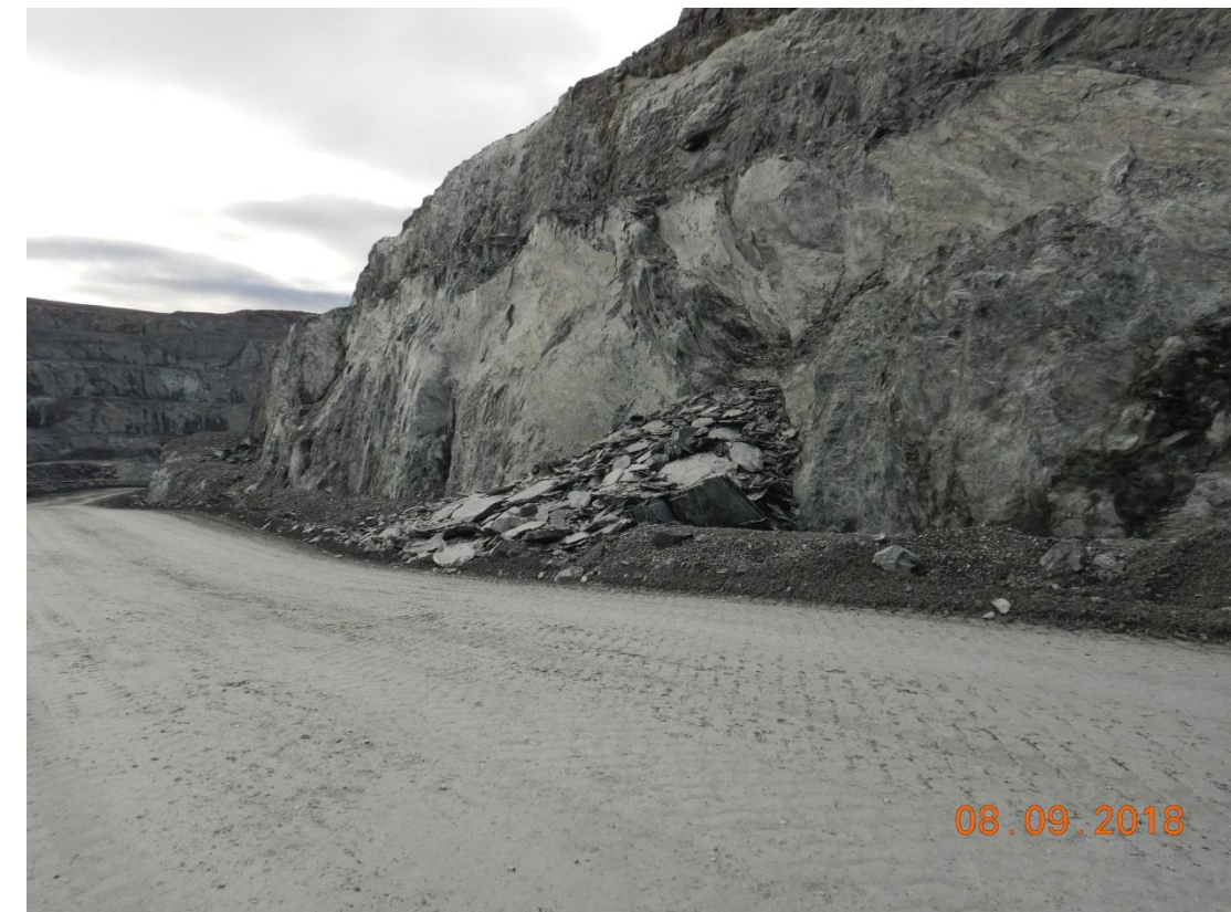
Zone E35: E3 Ramp, West Wall: Remove all loose material from previous rock fall.
