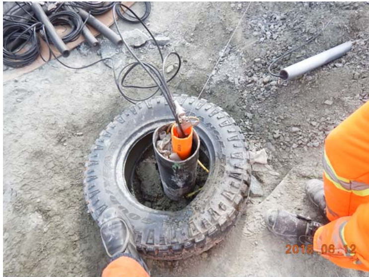
Photo 3.6: Connecting tube gently slid down the casing.
