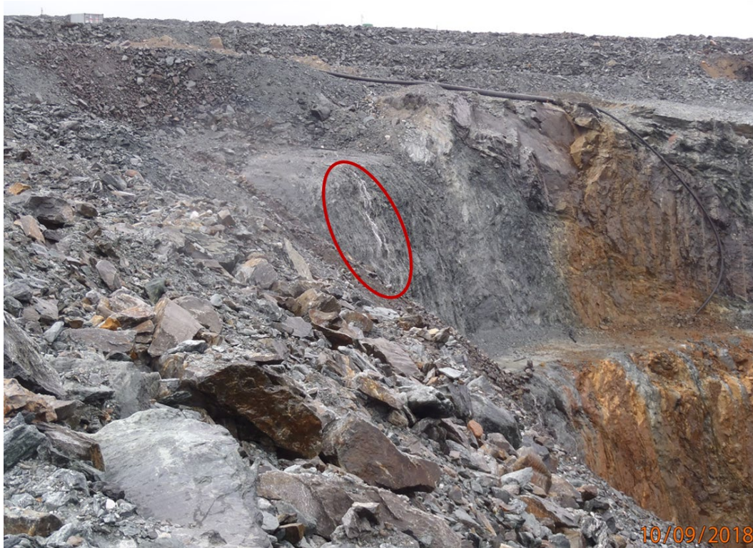
Photograph 7-11: Goose Pit uncontrolled water discharge on north pit wall
