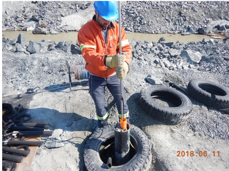
Photo 3.6: Connecting tube gently slid down the casing.
