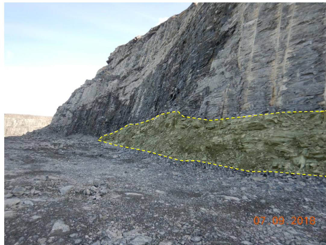
Zone P31: Phaser, East Wall: Scale the wall and hammer the toes when required.
