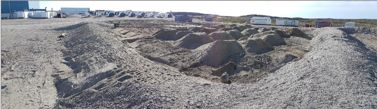
Photo 33: PHC Soil Placed into Phase 1 Cell Containment
