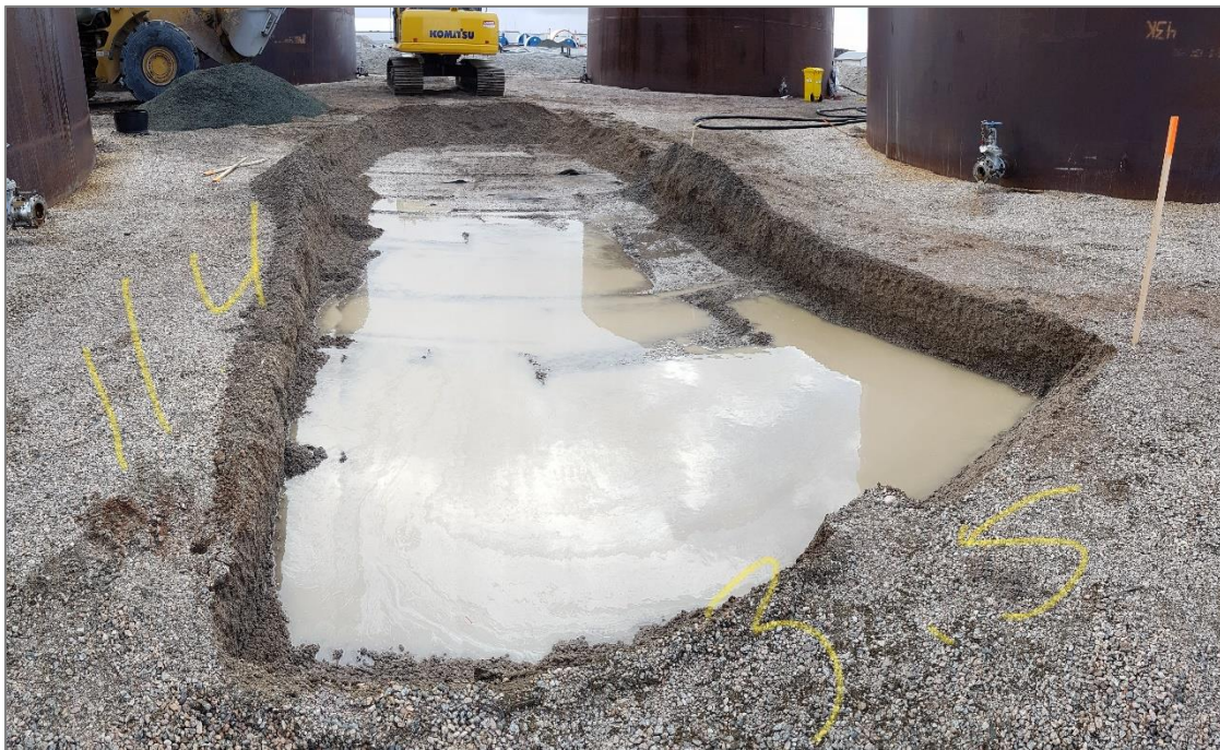
Photo 32: PHC Soil Excavation from Phase 2 Tank Farm Area.
