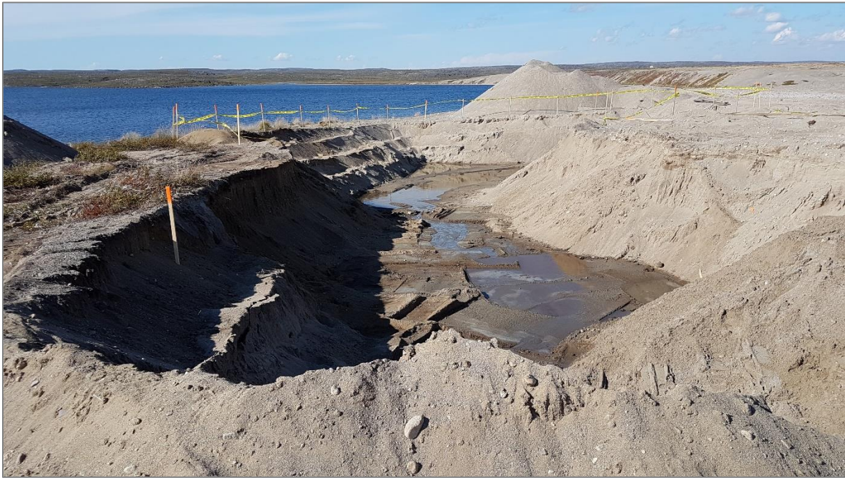
Photo 31: PHC Soil Excavation in Former Carat Lake Camp
