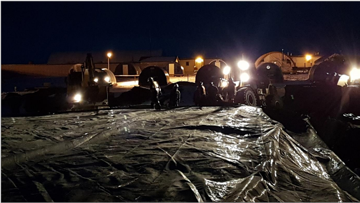
Photo 37: 2017 Installation of PHC Containment Cell Cover
