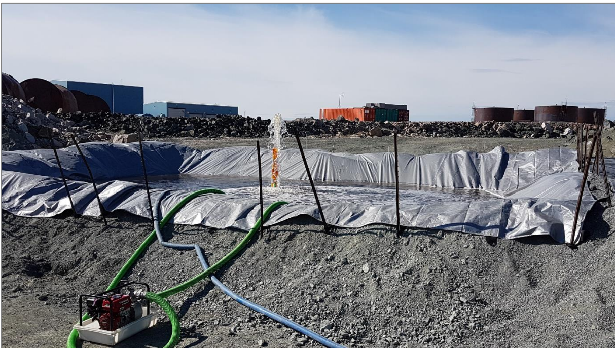
Photo 6: ROJV Aeration Treatment of Grey Water
