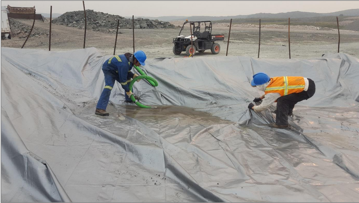
Photo 5: Repair of Grey Water Sump Liner
