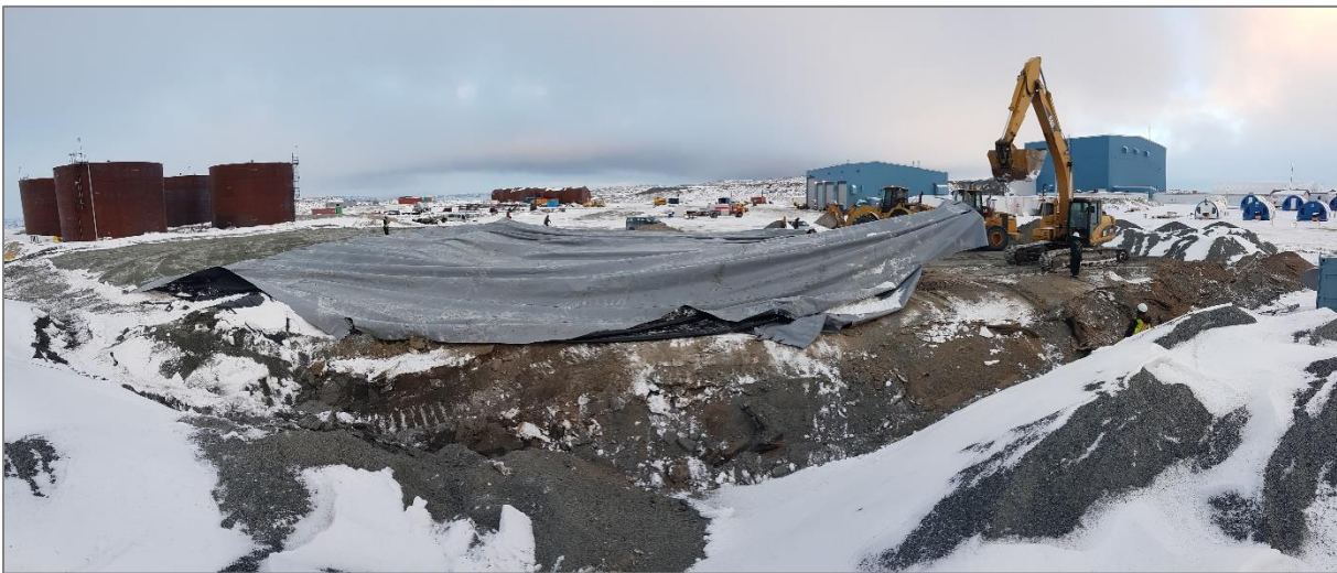
Photo 36: 2017 Installation of PHC Containment Cell Cover
