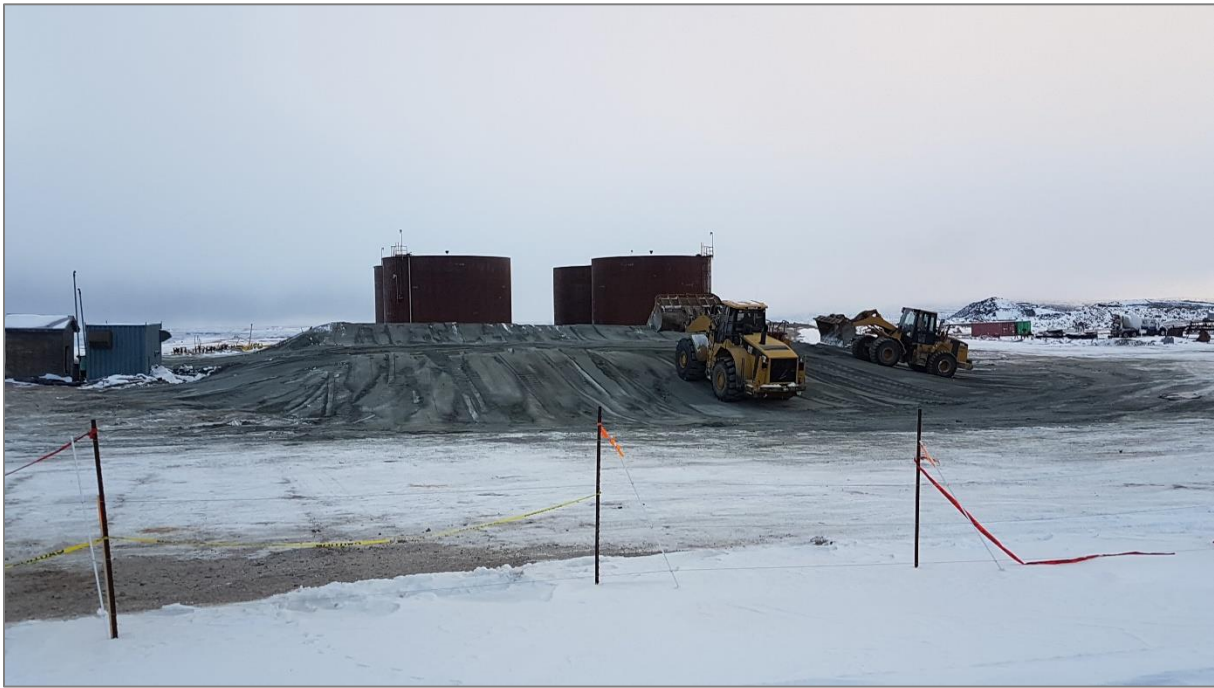
Photo 39: 2017 Construction of Containment Cell Protective Soil Cover.
