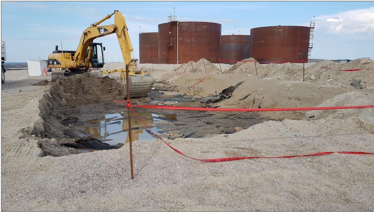
Photo 29: PHC Soil Excavation adjacent Phase 1 Cell
