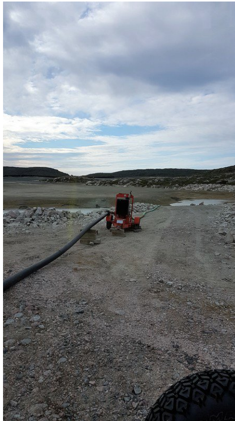
4in pump from PKCA to west dam
