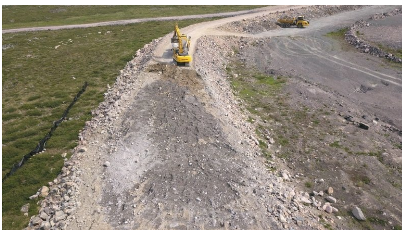
Excavation limit to frozen ground.
