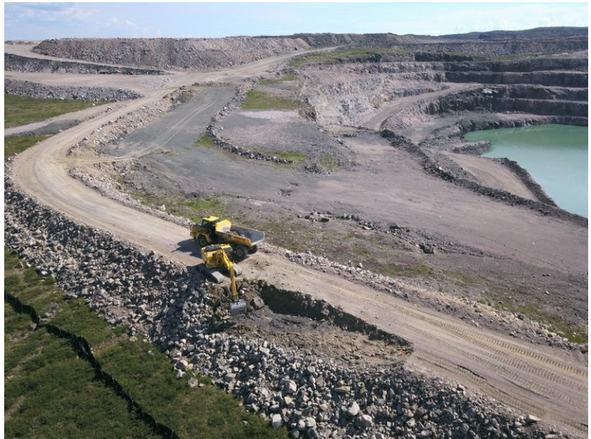
Excavation of outfall, hauled to adjacent area within pit.
