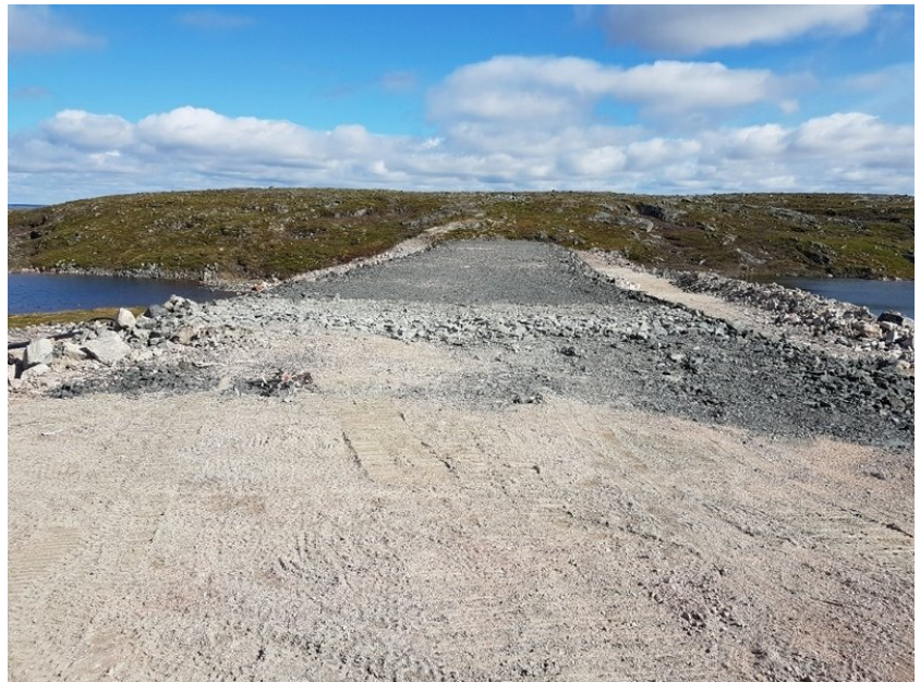
culvert refilled with backhoe
