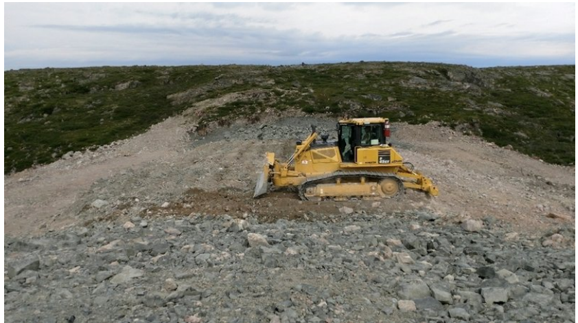
Looking north, dozer cross ripping.
