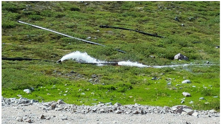
Discharge flow moved 2 feet no erosions
