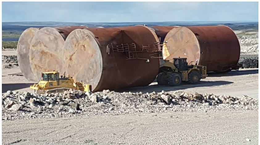
980G and D65 moved all tank form phase 1 to heli pad area
