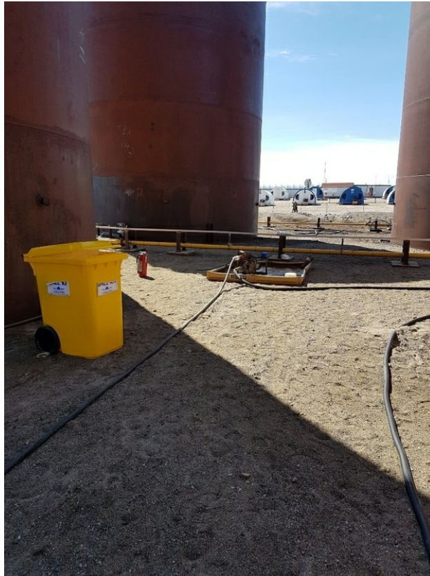
Fuel transferred from Tank 2 (11,433L), Tank 3 (12,520L) and Tank 4 (11,870L)
