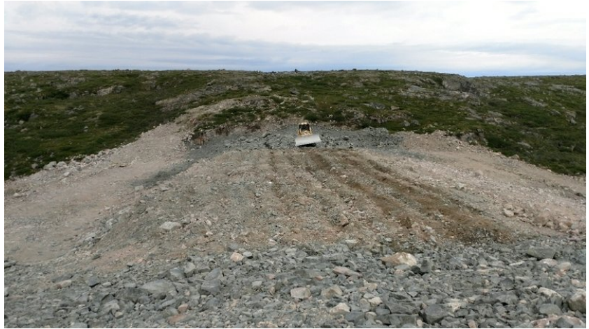
Looking north, dozer ripping frozen surface.
