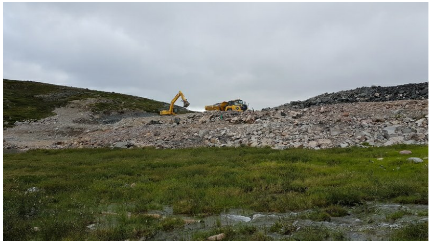
west dam breach 1 Excavator 2 rock trucks
