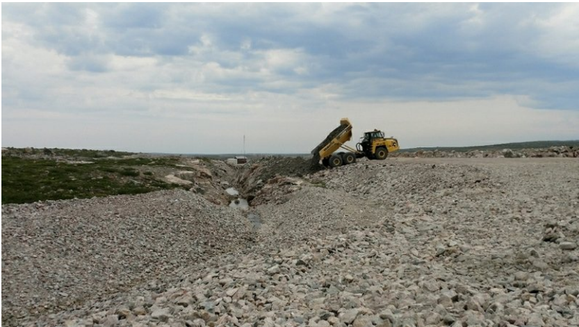
Dumping excavated material along edge of existing C1 Diversion channel.
