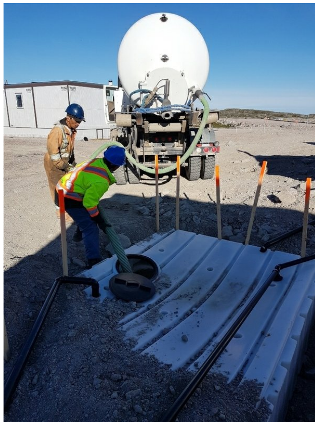
Gray water pumped out - 1200L taken to temporary berm (lined)
