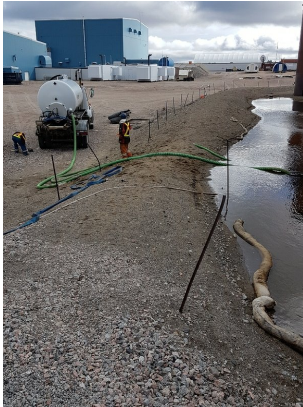
Dewatering berm water from Phase 1 Tank Farm Area
