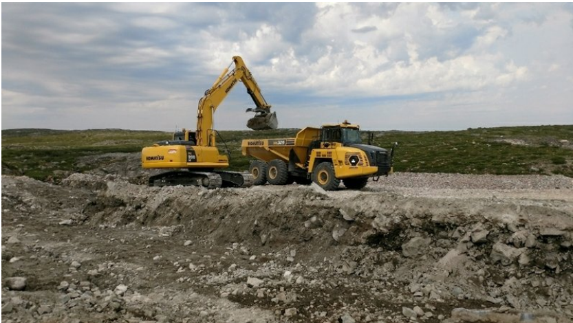
Looking northwest. Cut of unforzen material to 1.5m depth.
