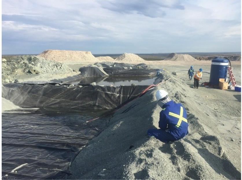
New greywater berm with water treated through granular activated carbon (GAC)
