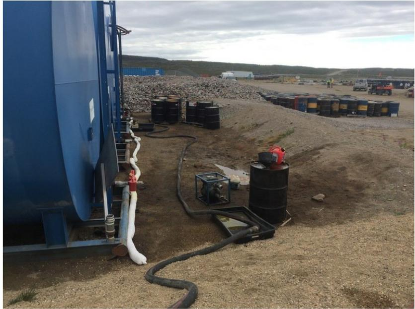
ROJV set up booms and trays in Fuel Berm of HWTA. Showing signs of spillage from transfer activities and use.
