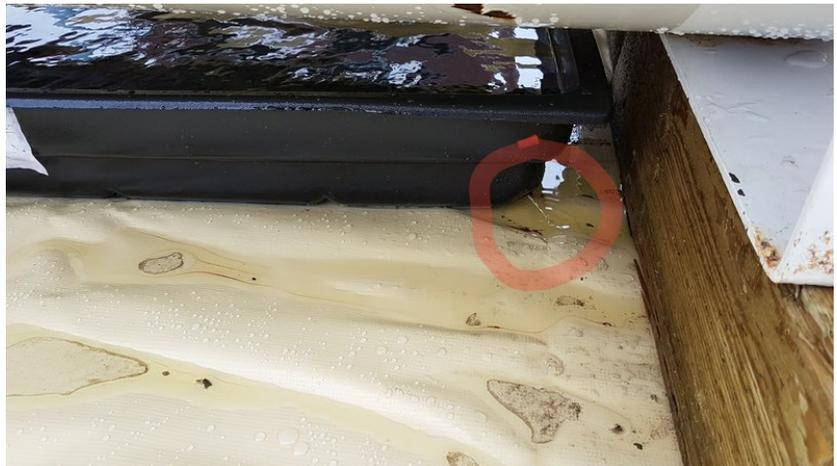
first tank that was setup had a leak under the tank also the spill tray they used had a hole in the corner as seen here in the picture
