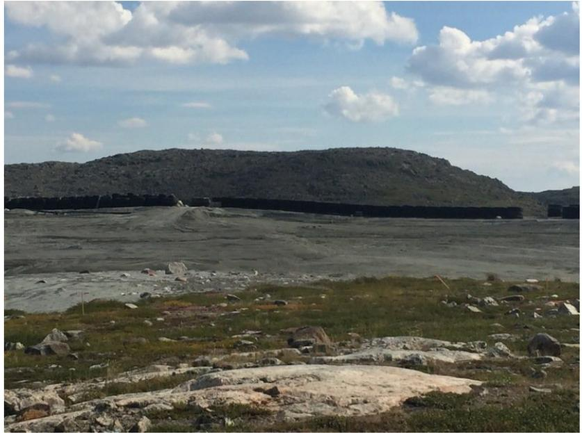
East side of PKCA. Covered on left and pre-graded only on right.
