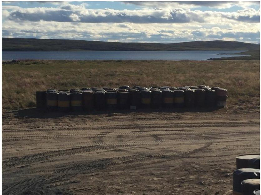
Additional empty drums opposite HWTA (from PHC contaminated soil). Upside down due to bulged out bottoms. ROJV asked to spot cleanup soils if residue found on ground surface (ROJV does not anticipate significant residue).
