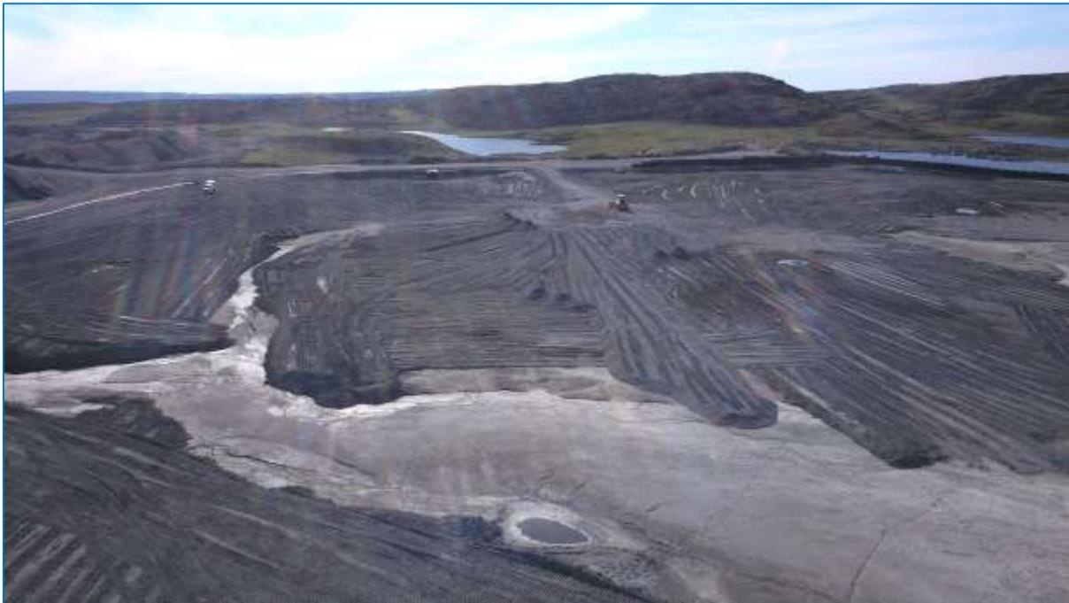
*PKCA - pre-grading perspective + constructed coarse PK central access road 0.5 to 1.0 m thick.*
