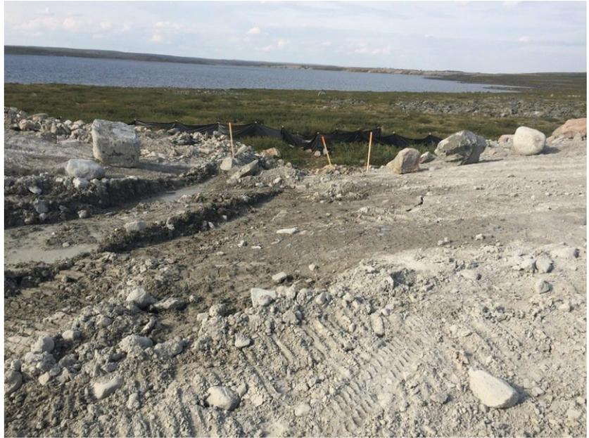
Downstream end of Open Pit Outfall. Additional excavation anticipated. Note downstream silt fencing.
