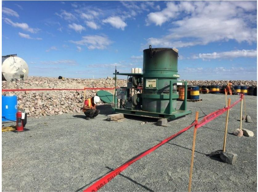
Weekly service shutdown (15 hours to cool and service). Preventative maintenance including removing soot.
