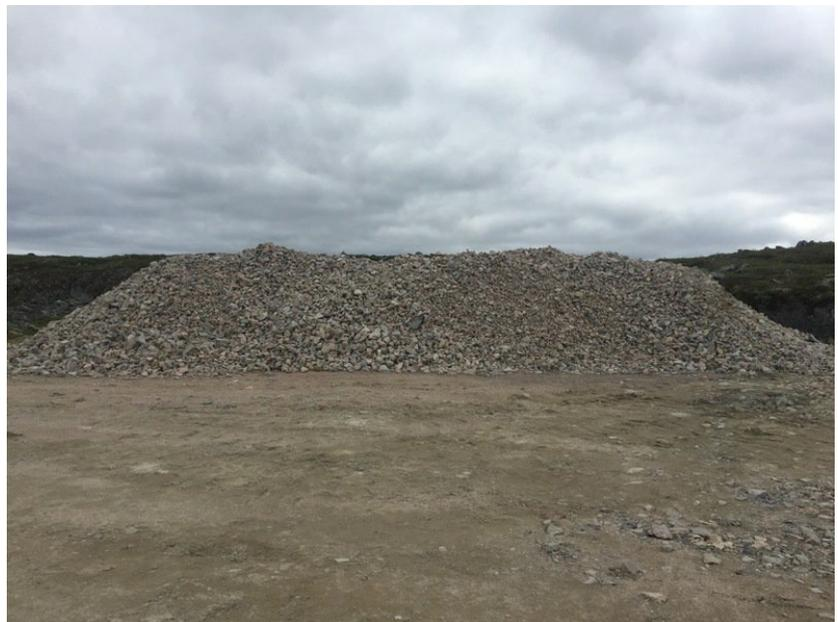
Post-screening riprap pile. Rough visual estimate of 300-500m3 (to be confirmed)
