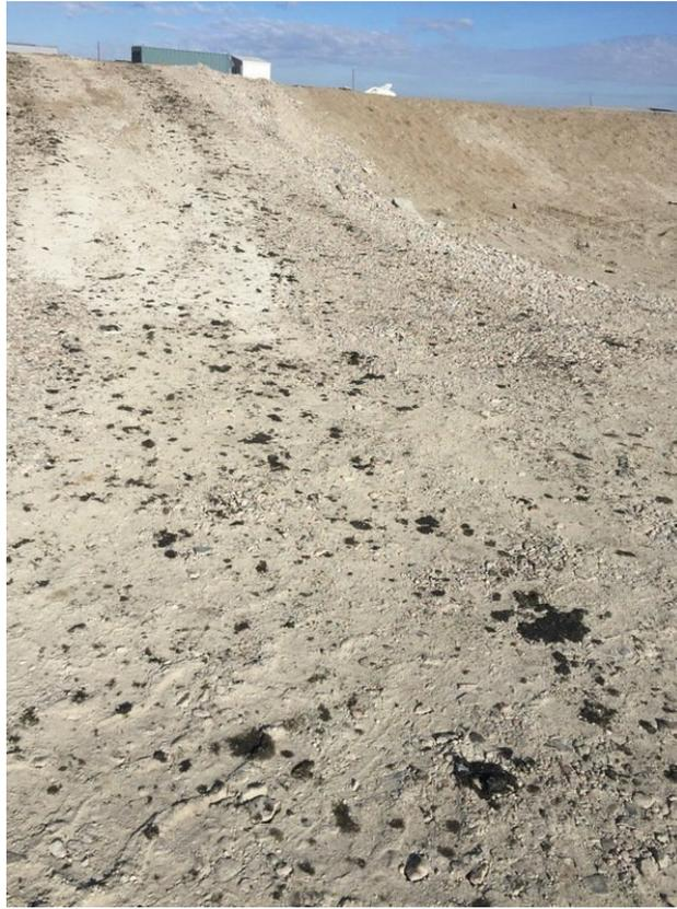
PHC contaminated soil from wheels of loader on ramp coming out of Phase 1. Small volume but work has just started.
