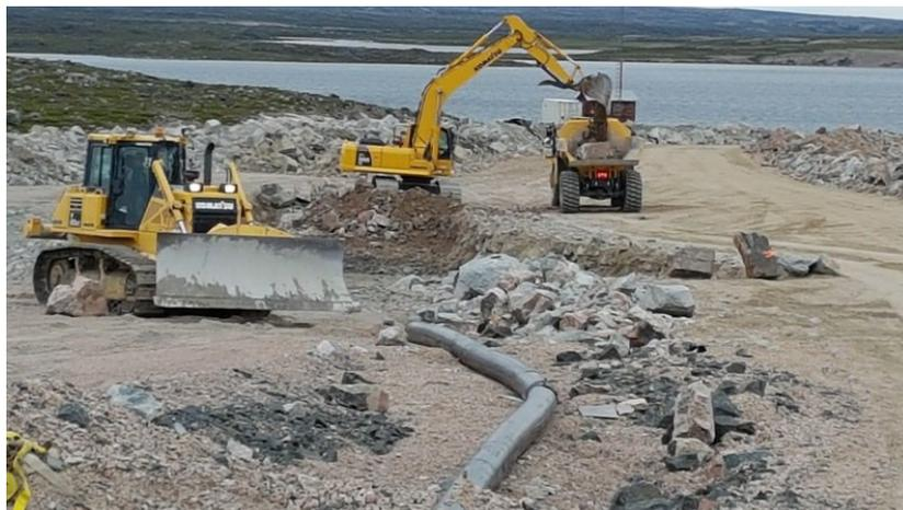
D-65 ripping at C-1 diversion Few bolder ripper having a hard time ripping
