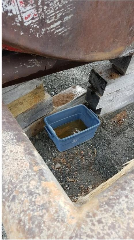
leak on red tank at phase 4 inside berm area was noticed and clean as soon as possible
