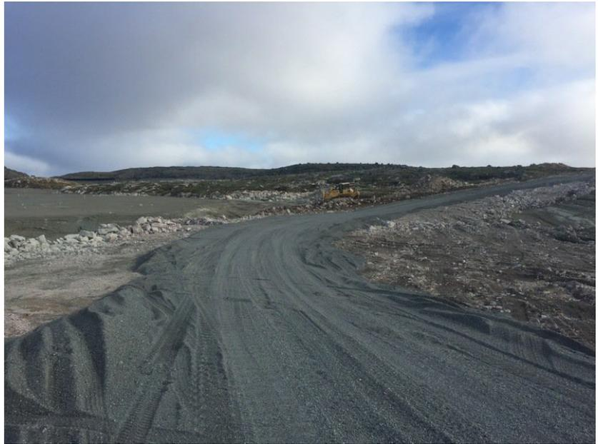
Dozer grading out piles of material on south end of Dyke A to fill low spot in PKCA
