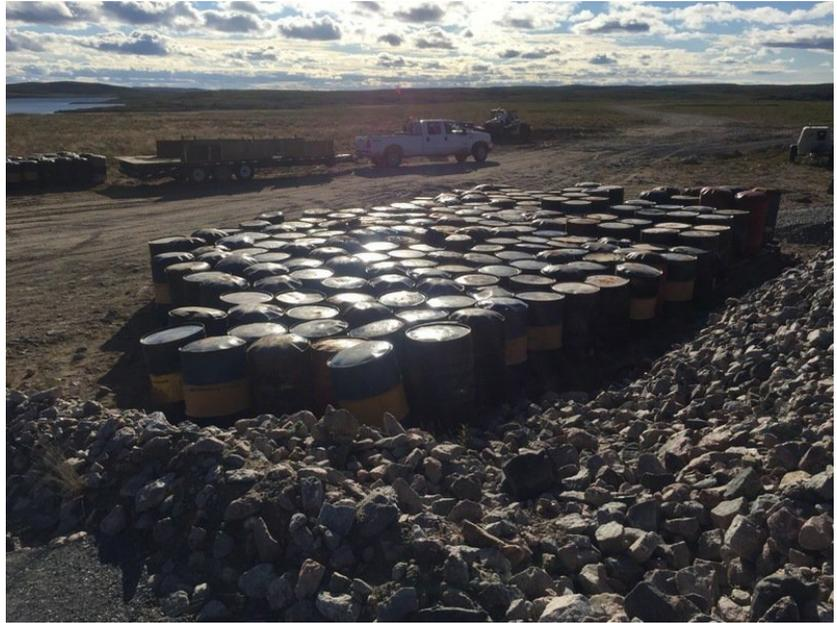
Drums of PHC contaminated soils empty and awaiting steam cleaning (where found to contain residue).
