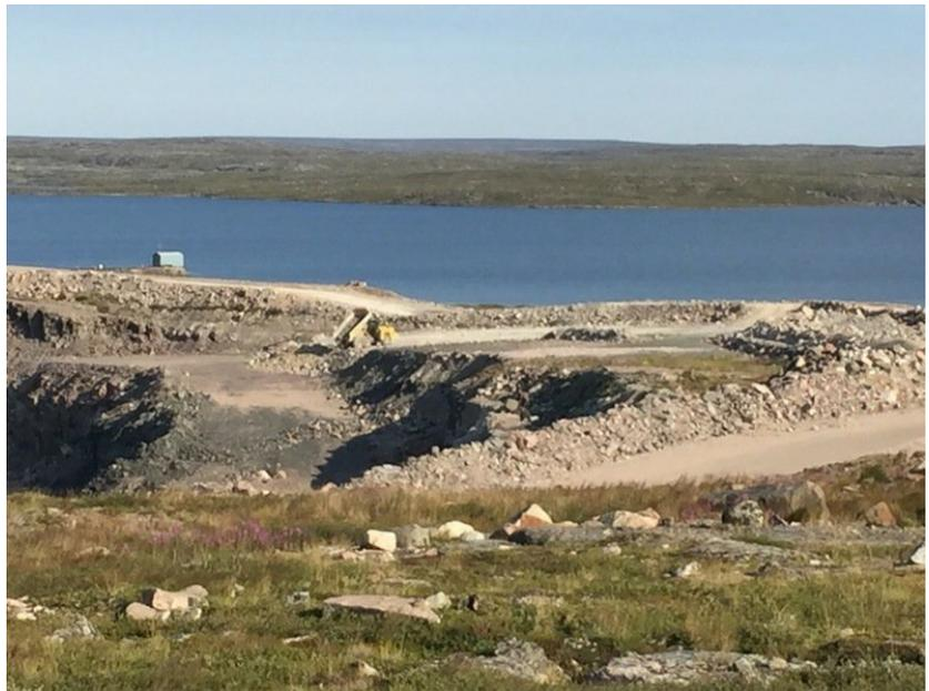
Excavated materials from C1 Diversion Berm cut hauled to pad at north end of pit
