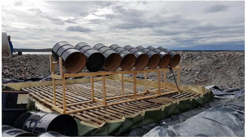
steam rack on pallets inside berm
