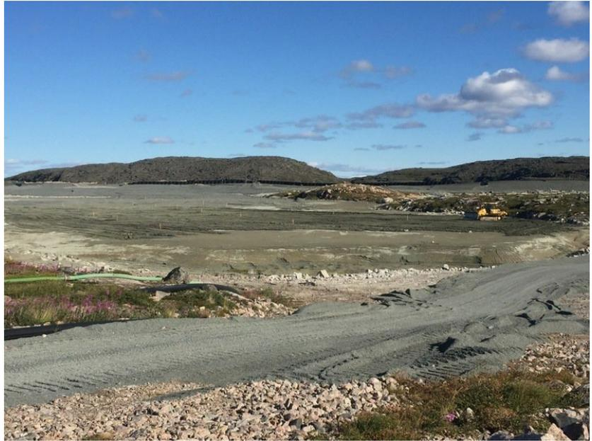
Pre-grading westward to Dyke A (sufficiently dry), stopping at the low/wet area adjacent to Dyke A
