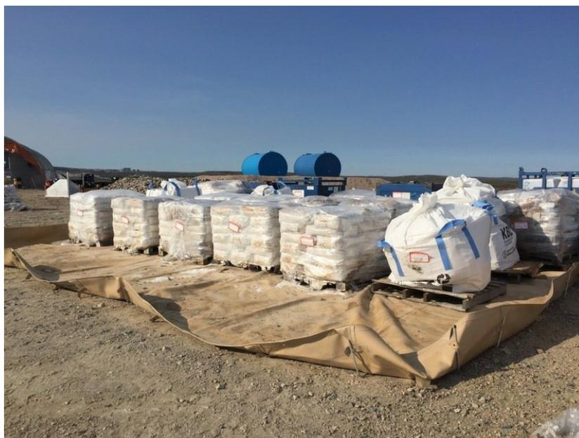
Temporary storage area at airstrip - Non-regulated solids (polymer), glycols and cubes of waste products within Insta-berm
