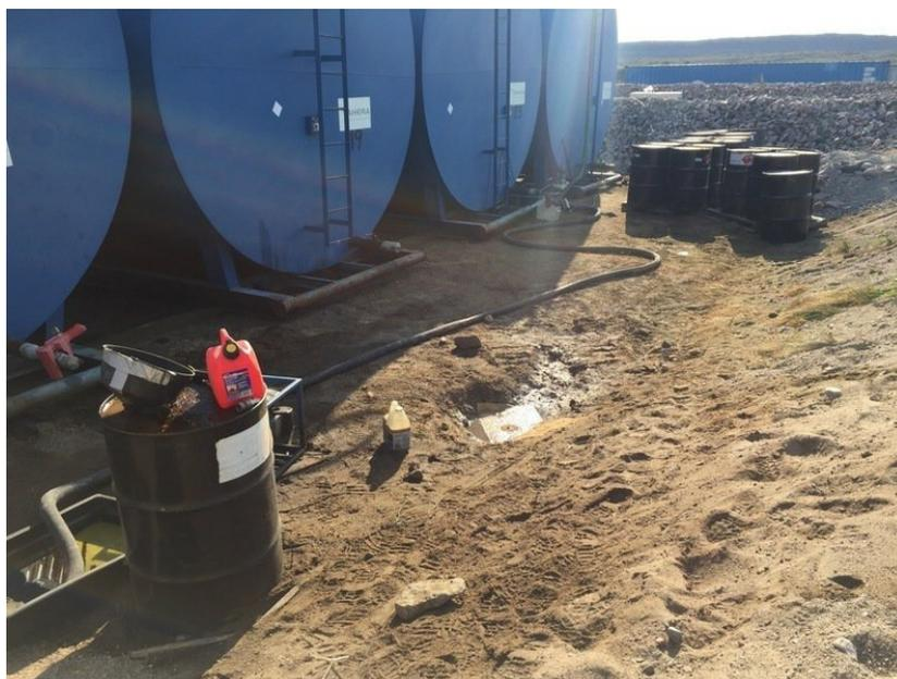
Within berm, some minor spillage may be happening when transferring fuel products.
