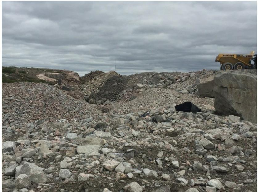
Diversion Channel backfilled from south to north to facilitate plug placement
