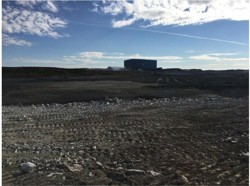
Cover placement now within roughly 200m of Dyke A, though final grading still required
