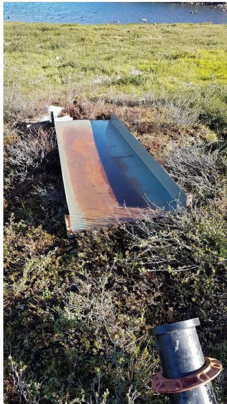
no erosion at discharge
