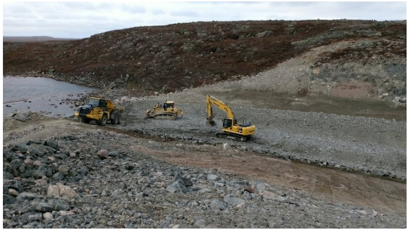
Placement of rip rap at last west section.
