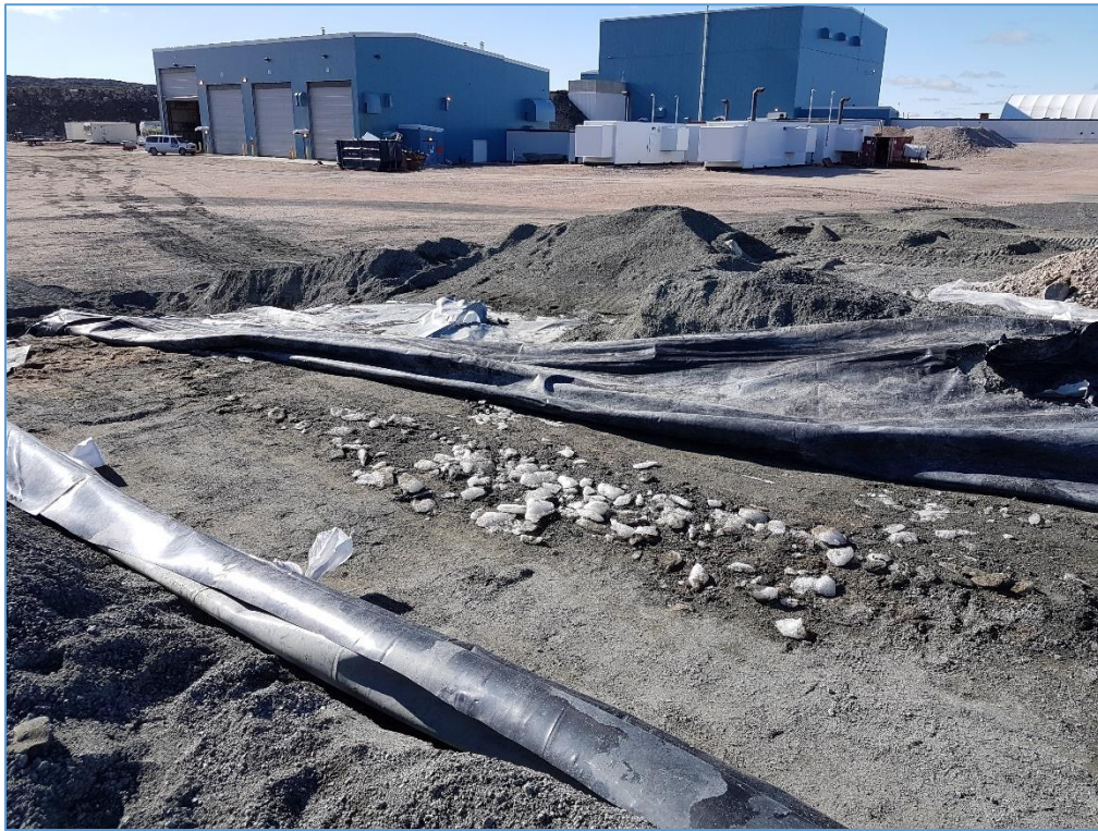
August 4 th , PHC Soil Containment Cell – Exposed underlying Coarse PK cushion layer.
