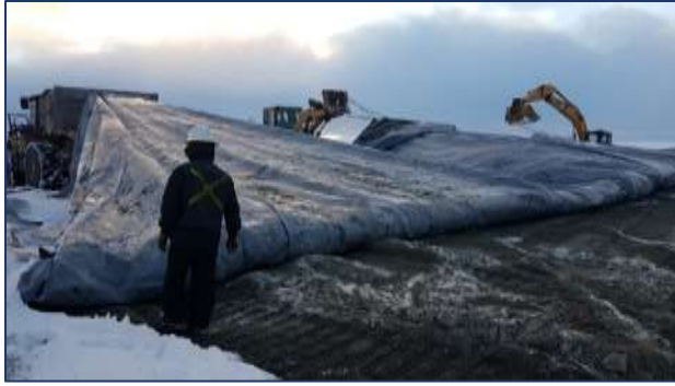
Photo 40. Pulling the liner over the southwestern half.
