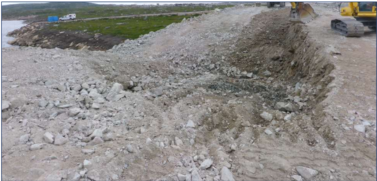
Photo 15. Easy digging in coarse, unfrozen material (looking north).
