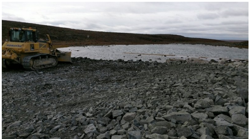
Tie in of rip rap at the west end of channel with surrounding terrain.
