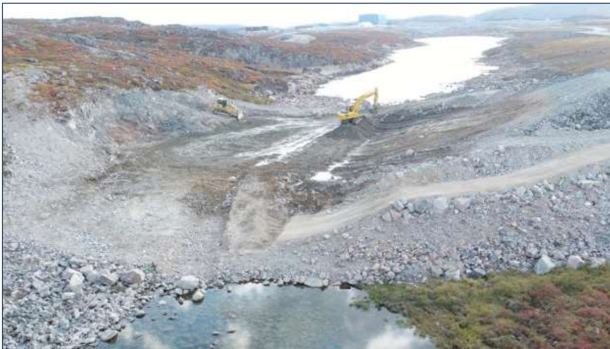
Photo 6. Excavation in the channel area; bedrock abutment on the north (left) side; blasting took place in the flat area (looking east/upstream).
