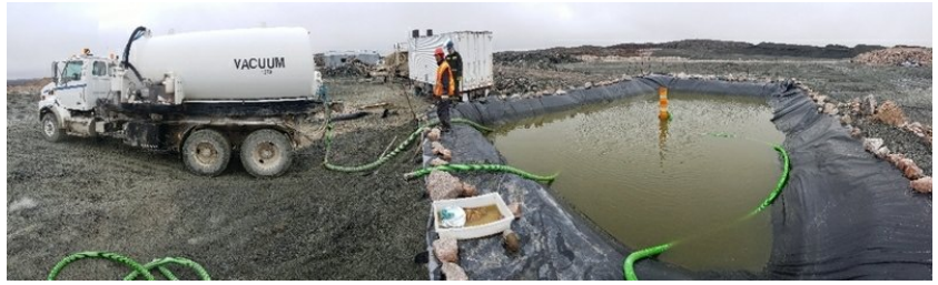
cell 7 gray water pumped into vac truck discharged into northeast side of pit
