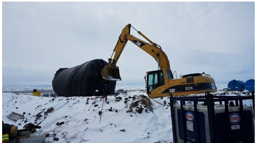
excavator lift backend to get the rest of waste fuel in to drums from blue tanks at phase4
