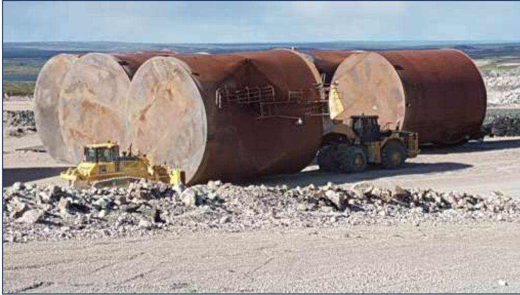
Photo 36. Placing the cleaned fuel tanks from Phase 1 into a laydown area on July 16 (looking northeast).
