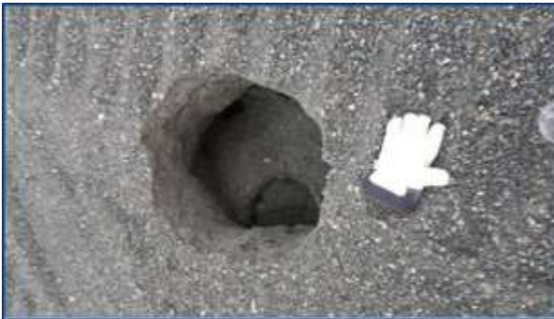
Photo 33. Close-up of sink hole in coarse PK cover.
