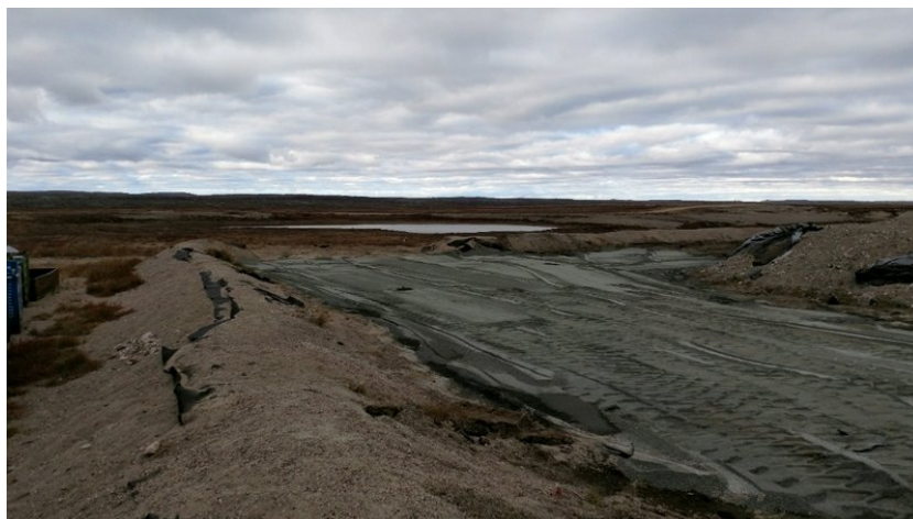
Former HWT barrel storage area - impacted soil removed, berm breached.
