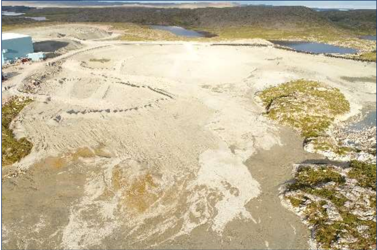
Photo 29. Overview of PKCA showing line of coarse PK piles up ready to be spread with a dozer (looking east).
