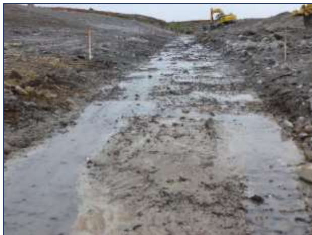
Photo 22. Channel during final excavation (looking east).
