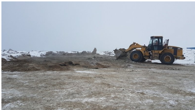
950 loader spreading gravel phase4
