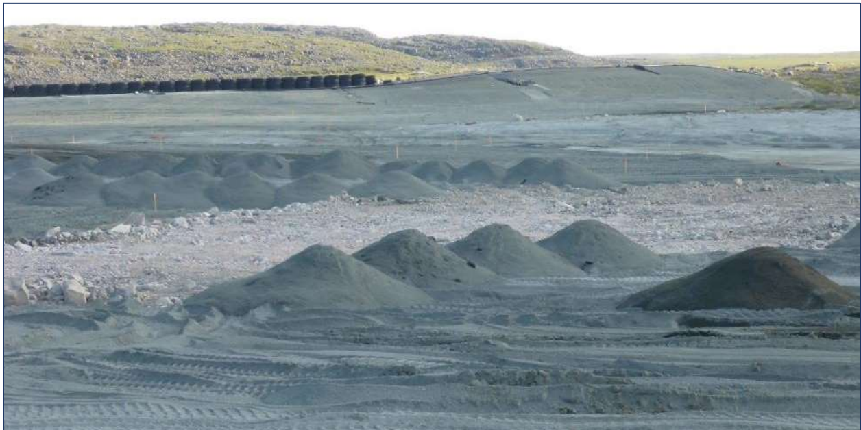
Photo 30. Close-up of coarse rock in drainage path, piles of coarse PK ready to spread, and equipment tracks in the coarse PK.
