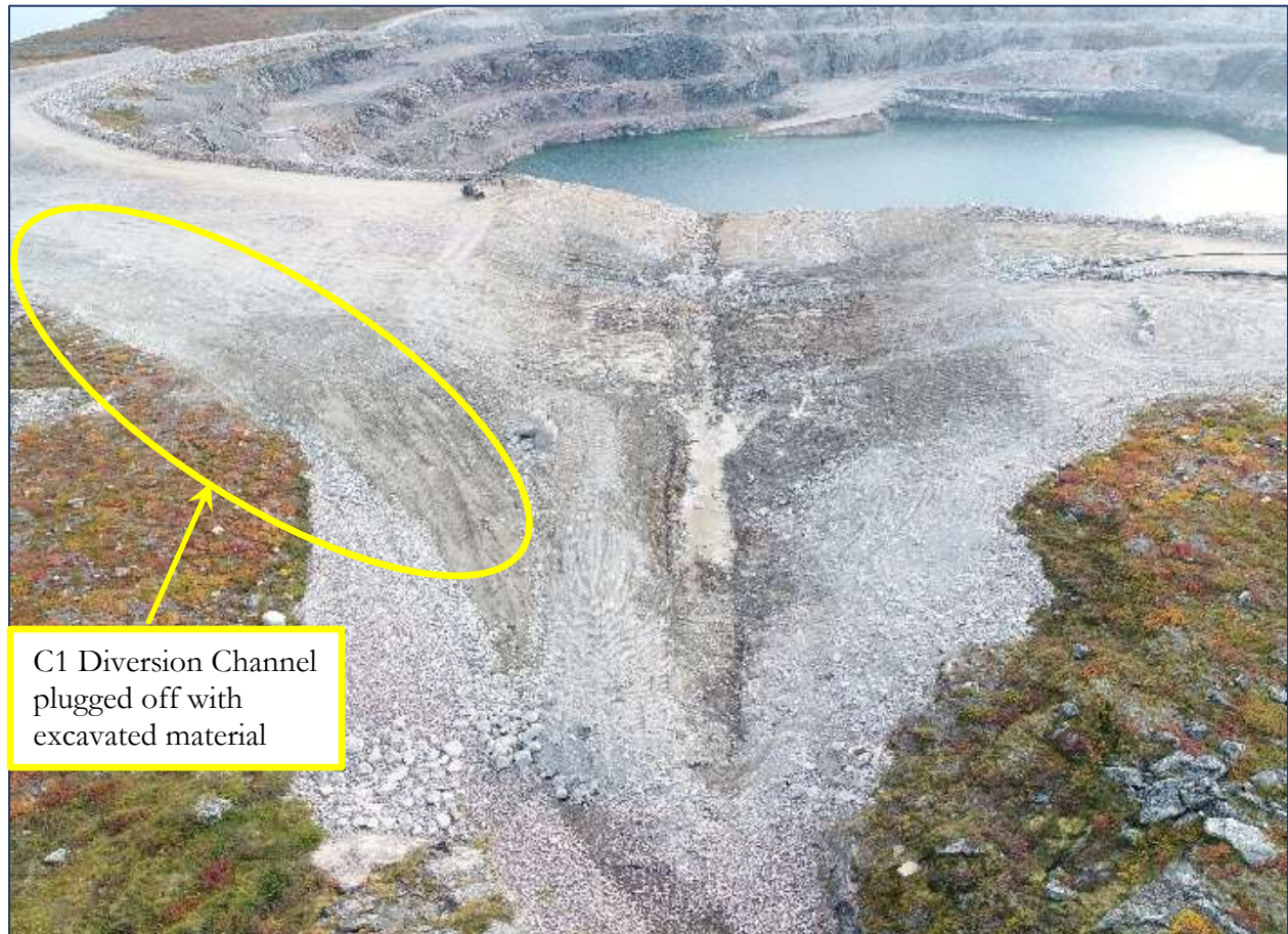
Photo 21. Overview of the C1 Diversion Breach construction nearing completion (looking east).
