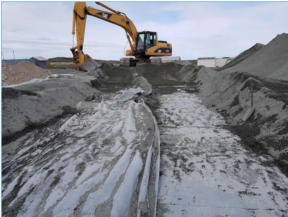
August 2 nd PHC Soil Containment Cell, looking west – uncovering LLDPE liner.
