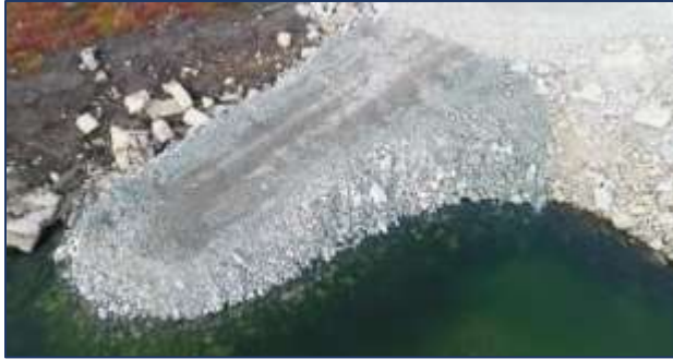
Photo 18. Energy dissipation ramp at outlet.
