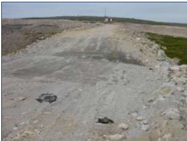
Photo 27. Remnant geotextile in the breach area (looking west). Photo 28. Original ground at the channel outlet.
