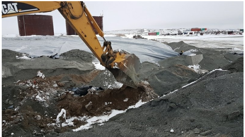
excavator covering liner at phase1
