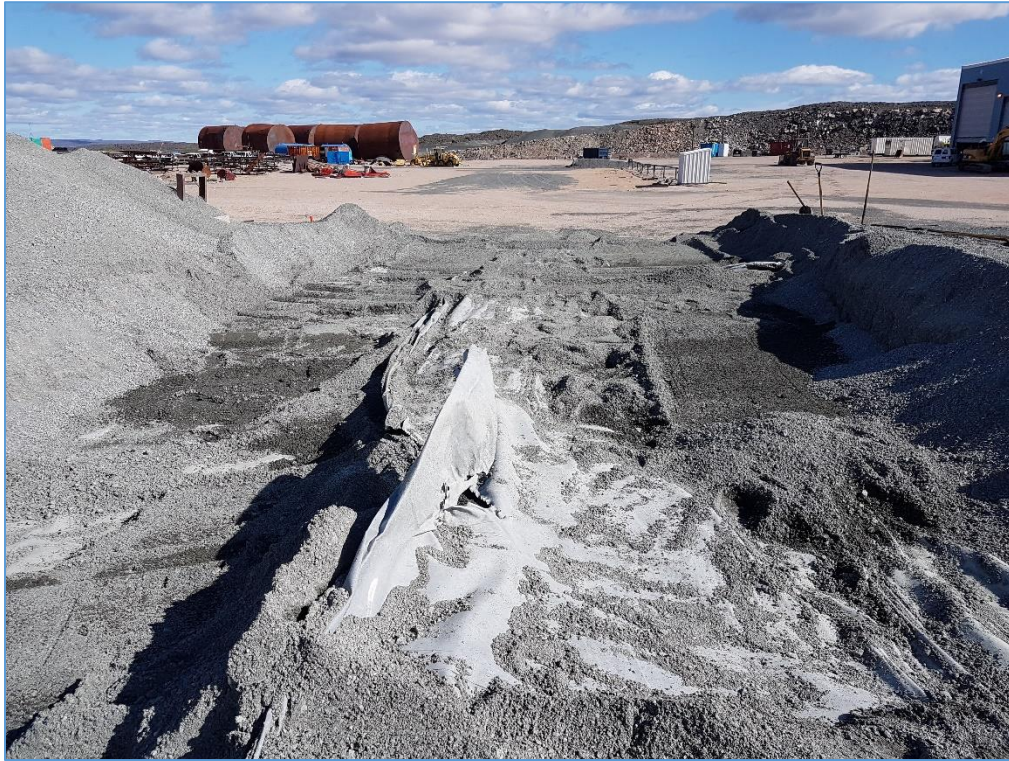
August 1 st PHC Soil Containment Cell, looking east – uncovering LLDPE liner.
