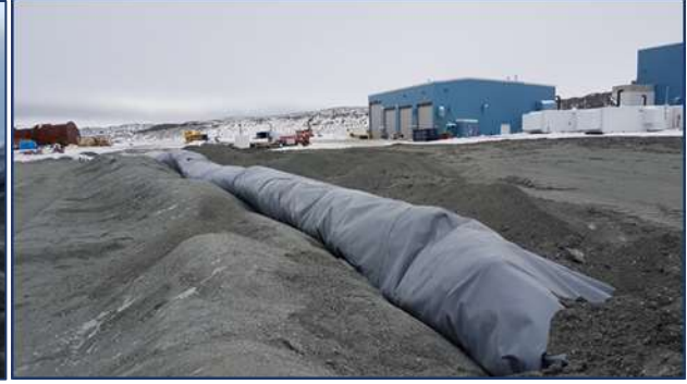
Photo 41. Bulge in the liner where snow was trapped.
