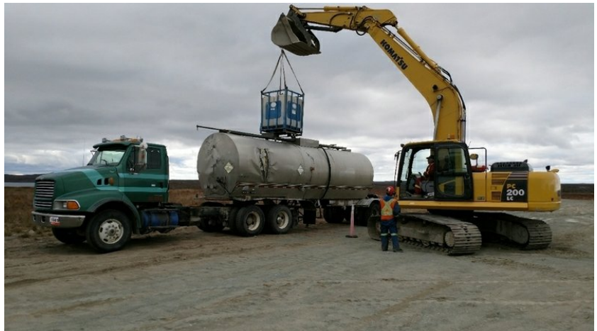
Transfer of contact water stored in totes to the tanker.
