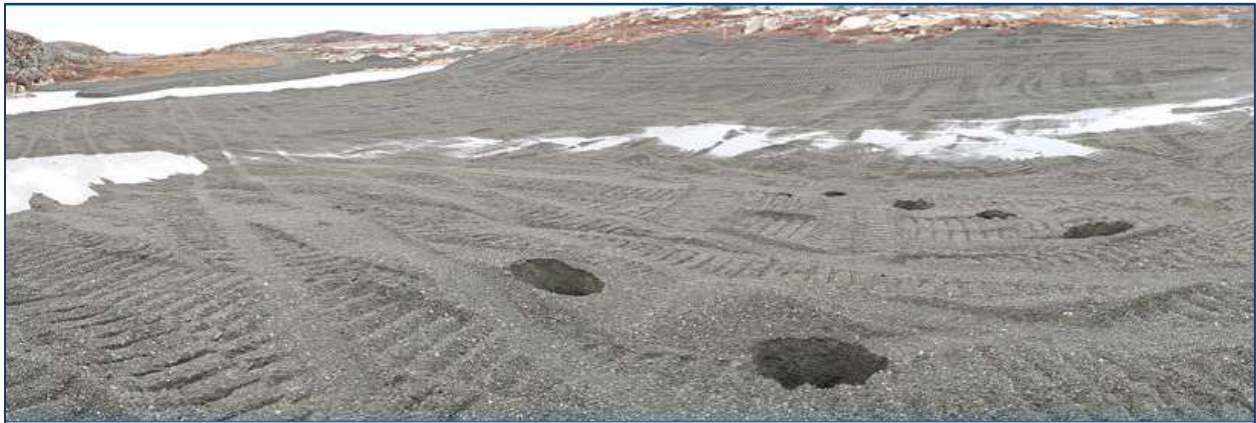
Photo 32. Sink holes developed in the coarse PK cover in the southeast area of the PKCA (looking northeast).
