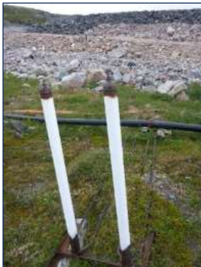
Photo 4 Inactive thermosyphon pipes.
