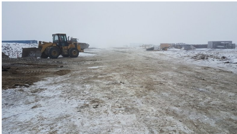
980 spreading gravel phase4
