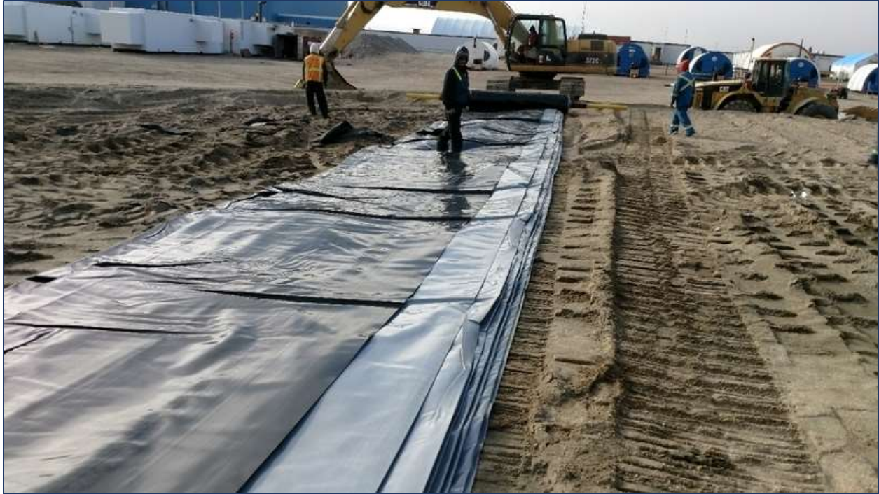
Photo 38. Preparing the liner to pull over the contaminated material.
