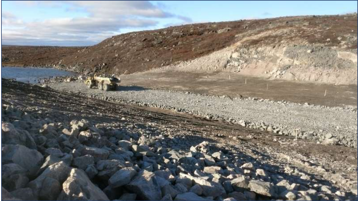
Photo 7. Placing riprap in the channel; grade stake markers visible on north/far side (downstream to the left).
