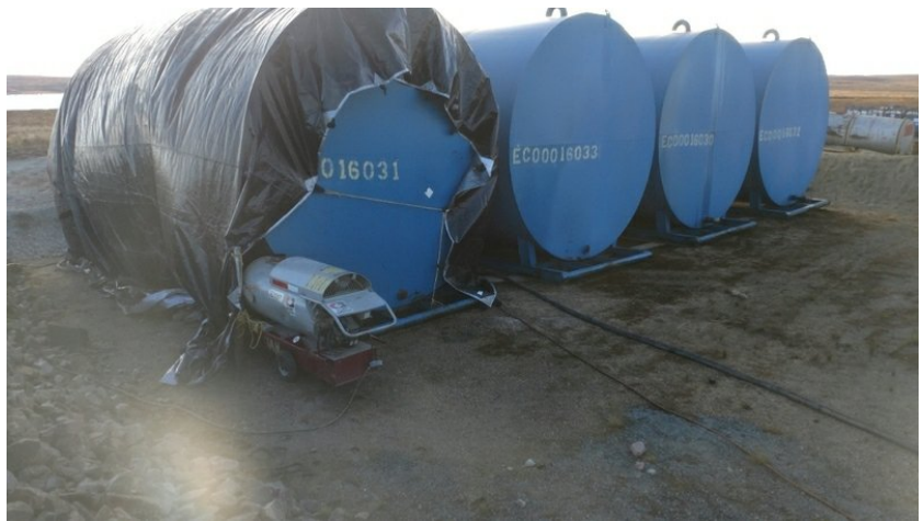
Frost fight set up at the back of T22.
