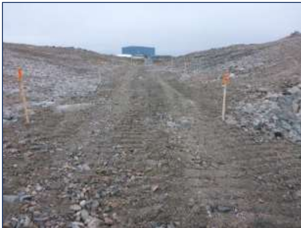
Photo 16. Channel staked ready for riprap (looking east).
