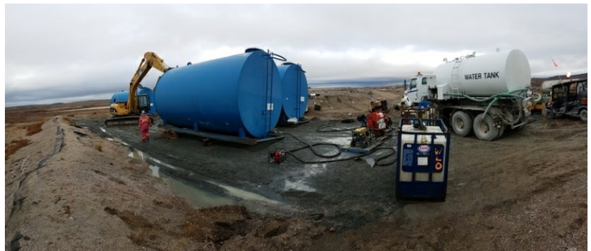
Steam cleaner plugged with sand change tank to water truck
