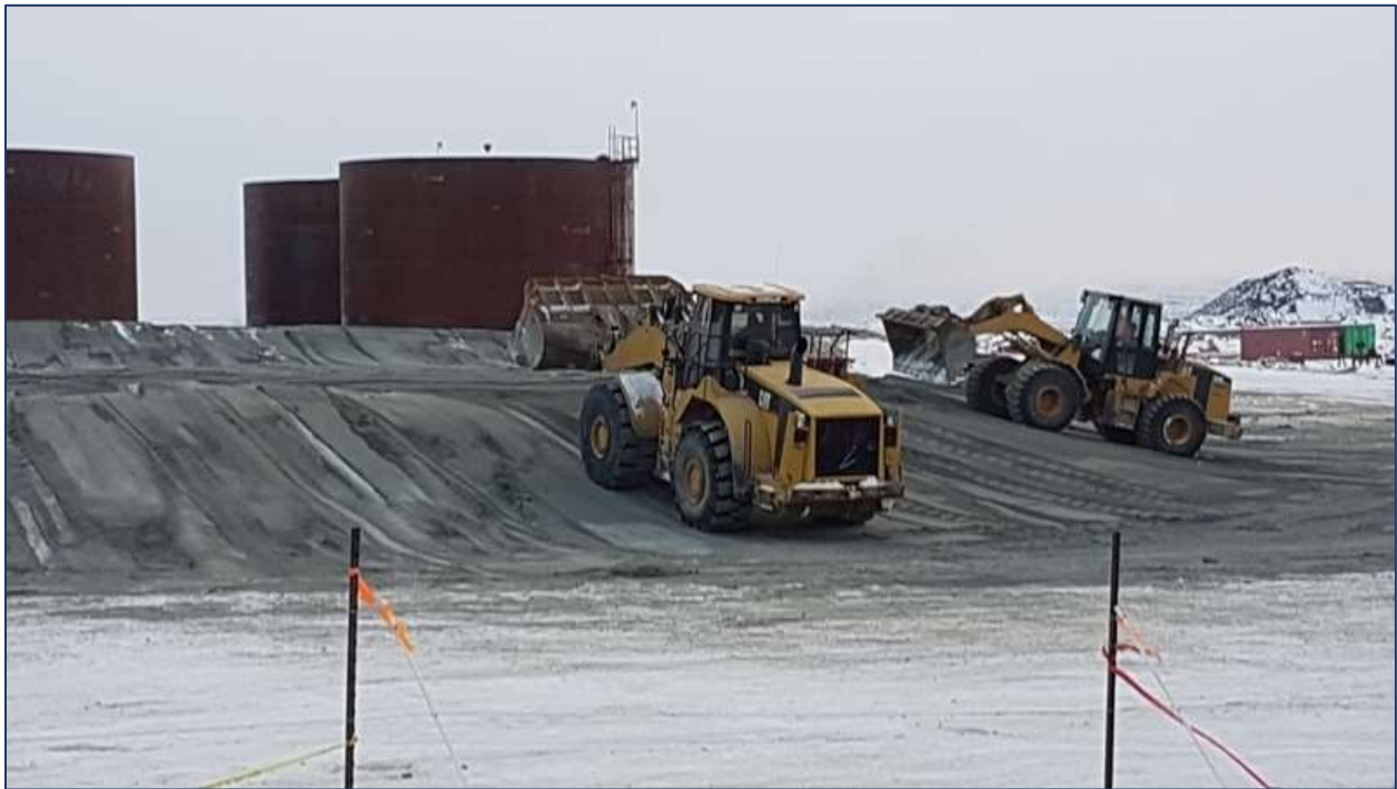
Photo 42. Covering the liner with coarse PK at the Phase 1 Contaminated Material Containment Area (looking north).
