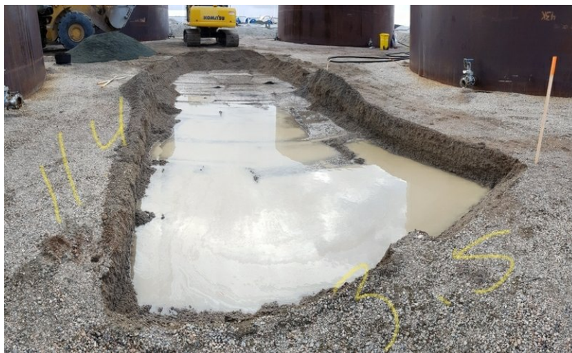
Between Tank 11 and 12; 11.4 m ×3.5 m and 0.55 m depth
