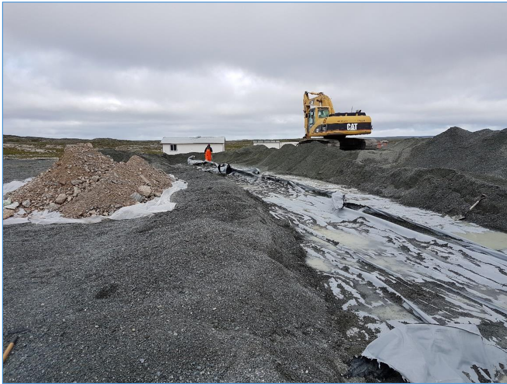
August 3 rd PHC Soil Containment Cell – Stockpiled excavated stained soil to be placed in cell.
