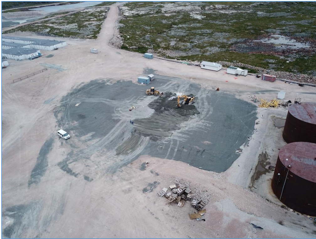
August 5 th , PHC Soil Containment Cell – Placement of protective Coarse PK cover.
