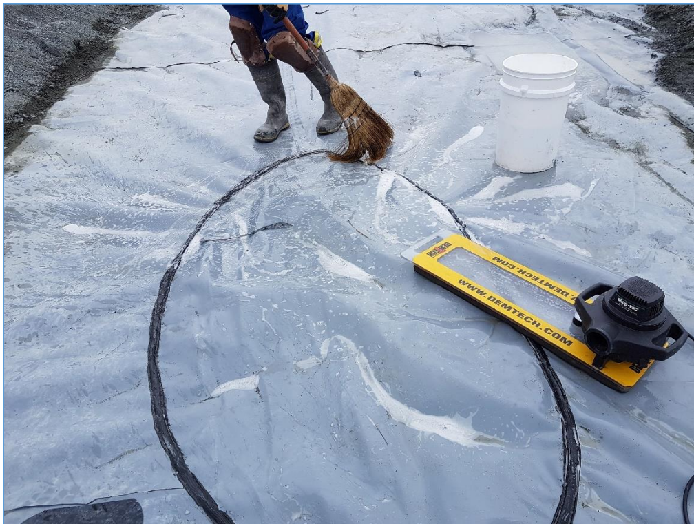
August 5 th , PHC Soil Containment Cell – Vacuum test of extrusion welds.
