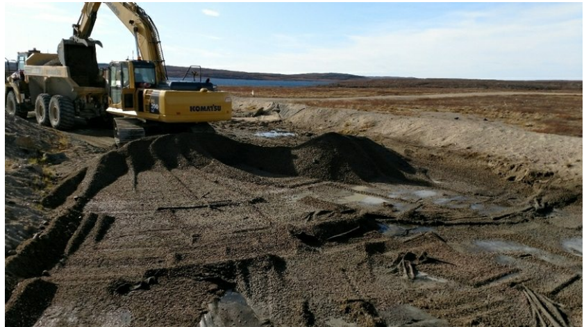
Impacted soil excavation.
