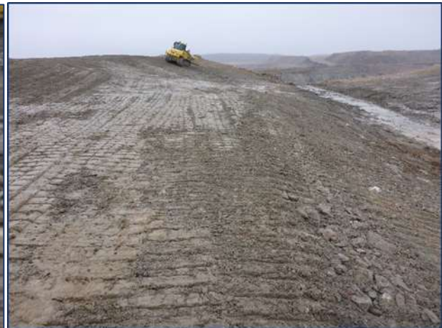
Photo 23. Dozer grading the north slope (looking east).
