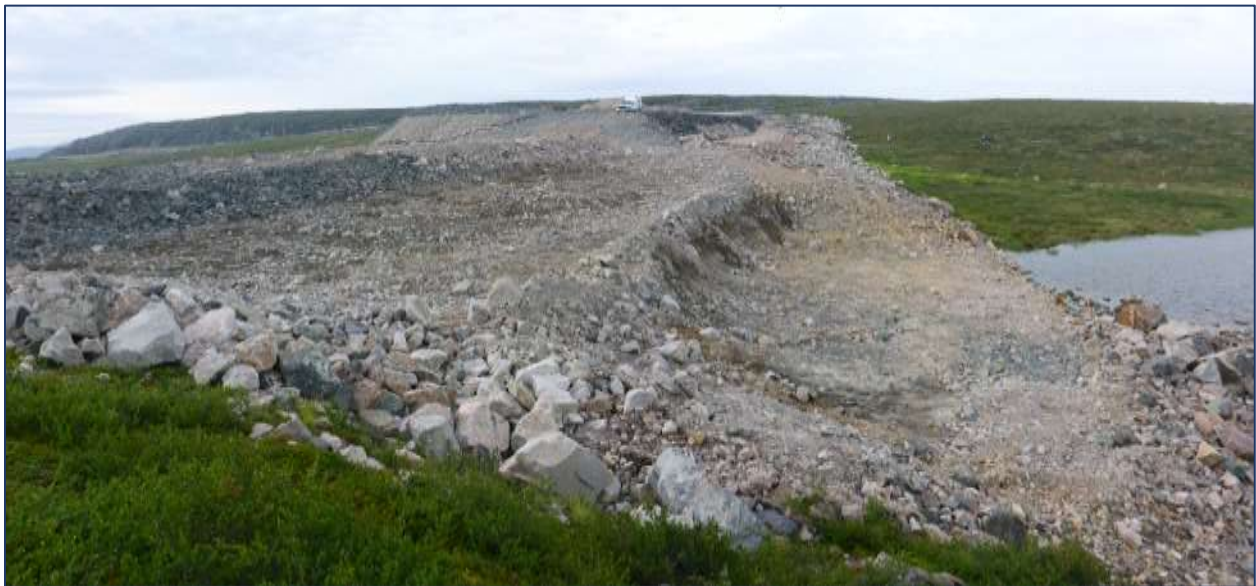
Photo 3. Two excavation benches on the downstream side of West Dam; frozen ground was pervasive (looking south).
