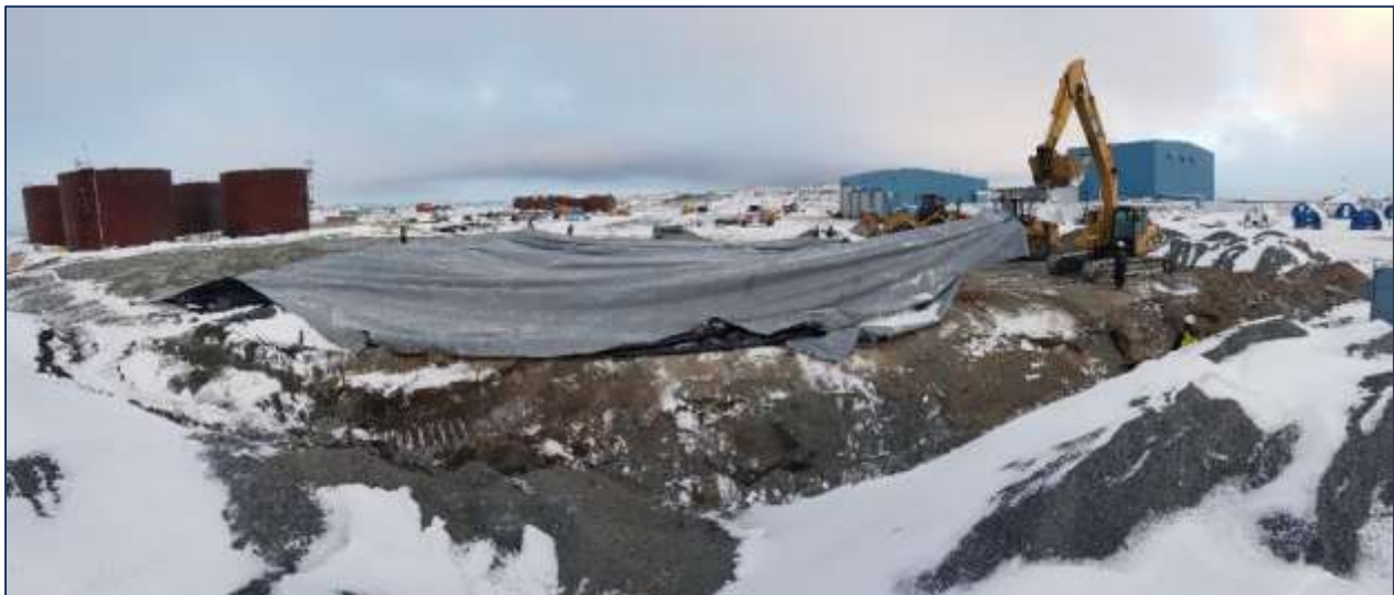
Photo 39. Pulling the liner over the southwestern half of the Phase 1 consolidation area.
