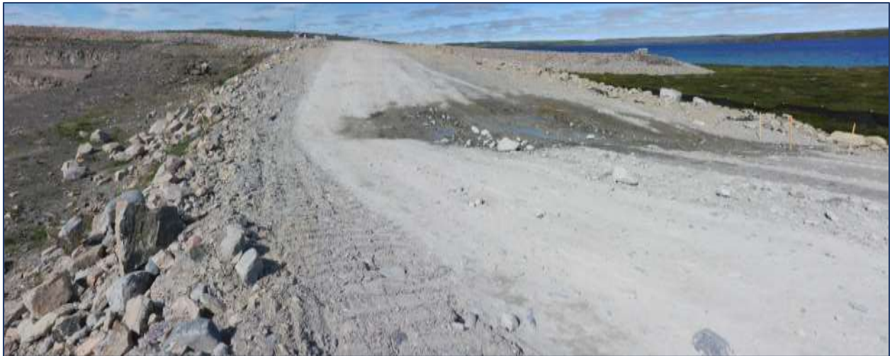
Photo 26. Overview of Open Pit Outfall Breach area and absence of ground on the upstream (left) side (looking west).
