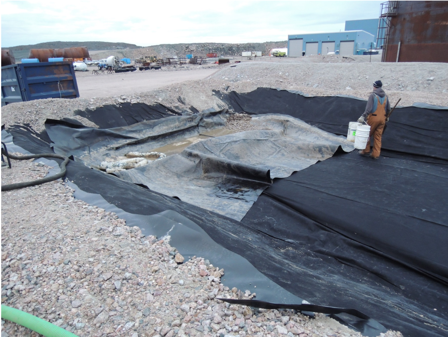
Picture #4 – Removal of Soil & Sludge by Shovel
