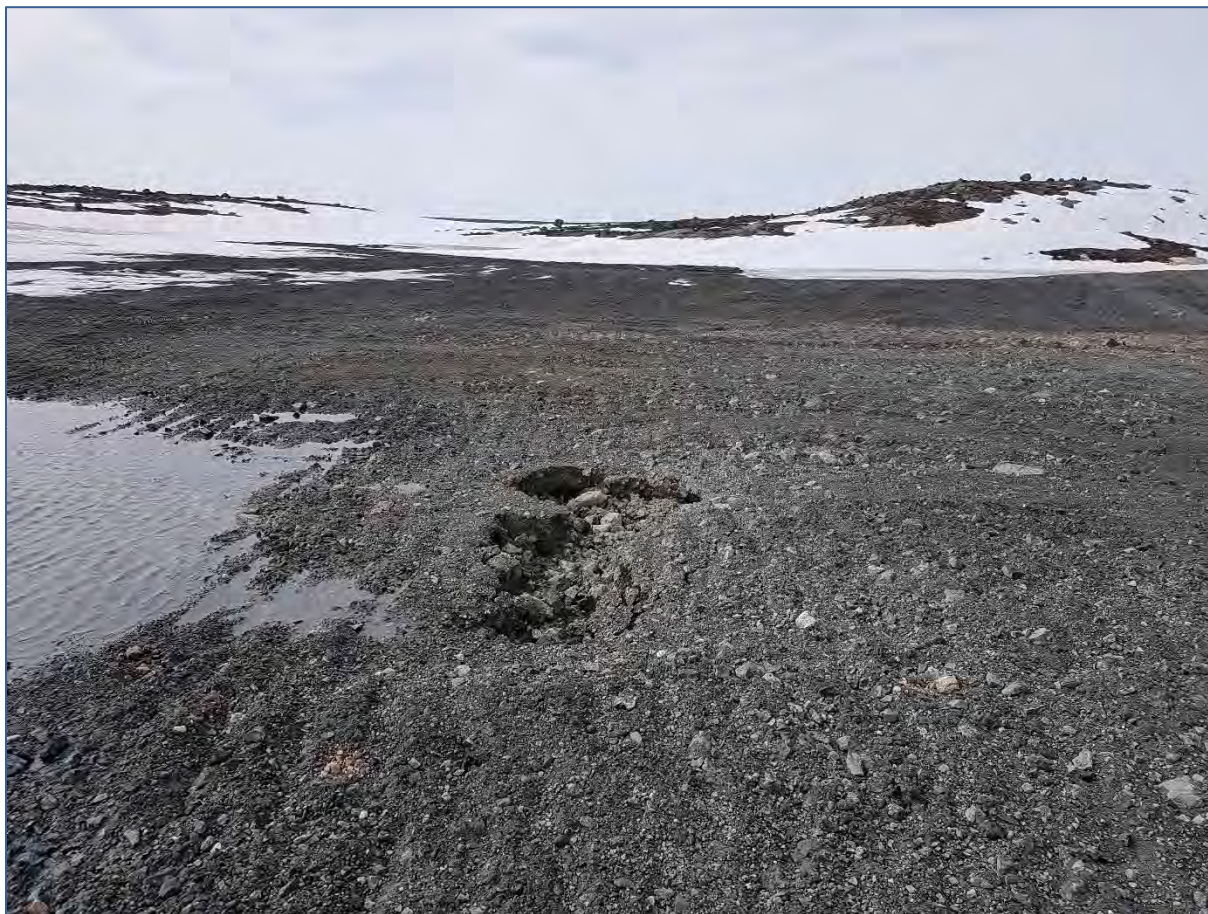
Photo 14: June 5, 2018 PKCA Cover, North PKCA – New Pot Hole.
