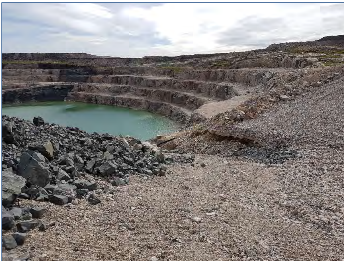
Photo 25: August 2, 2018 C1 Channel – Looking South, Erosion at Outlet into Open Pit.
