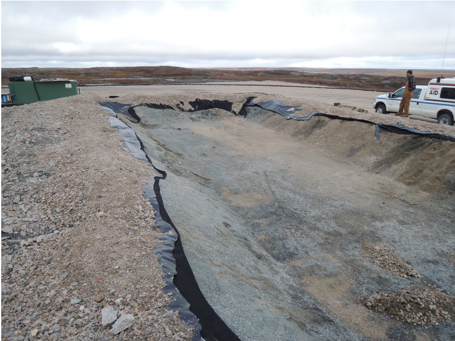
Picture #5 – Both Geomembrane and Geotextile Removed
