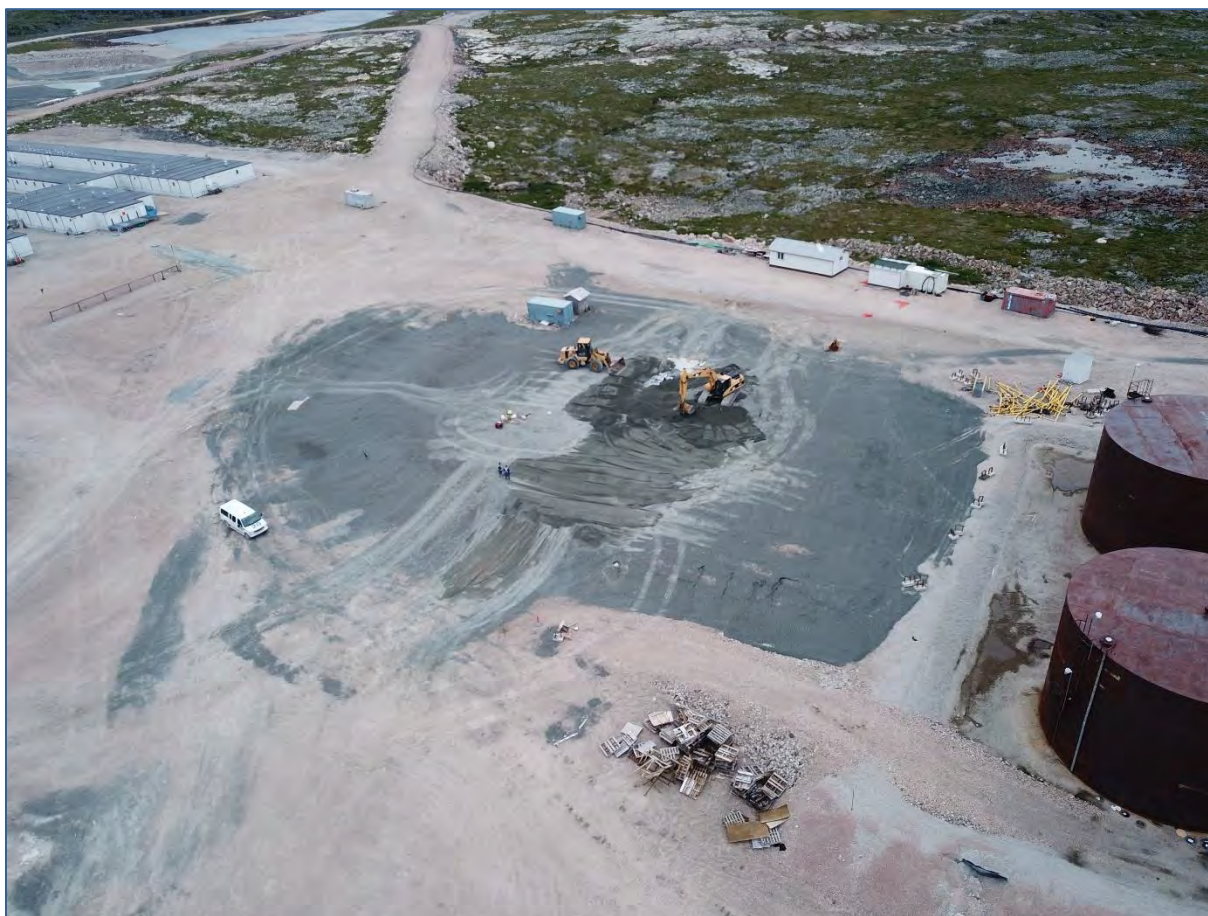
Photo 9: August 5, 2018 PHC Containment Cell Cover – Post-Deficiency Repair.
