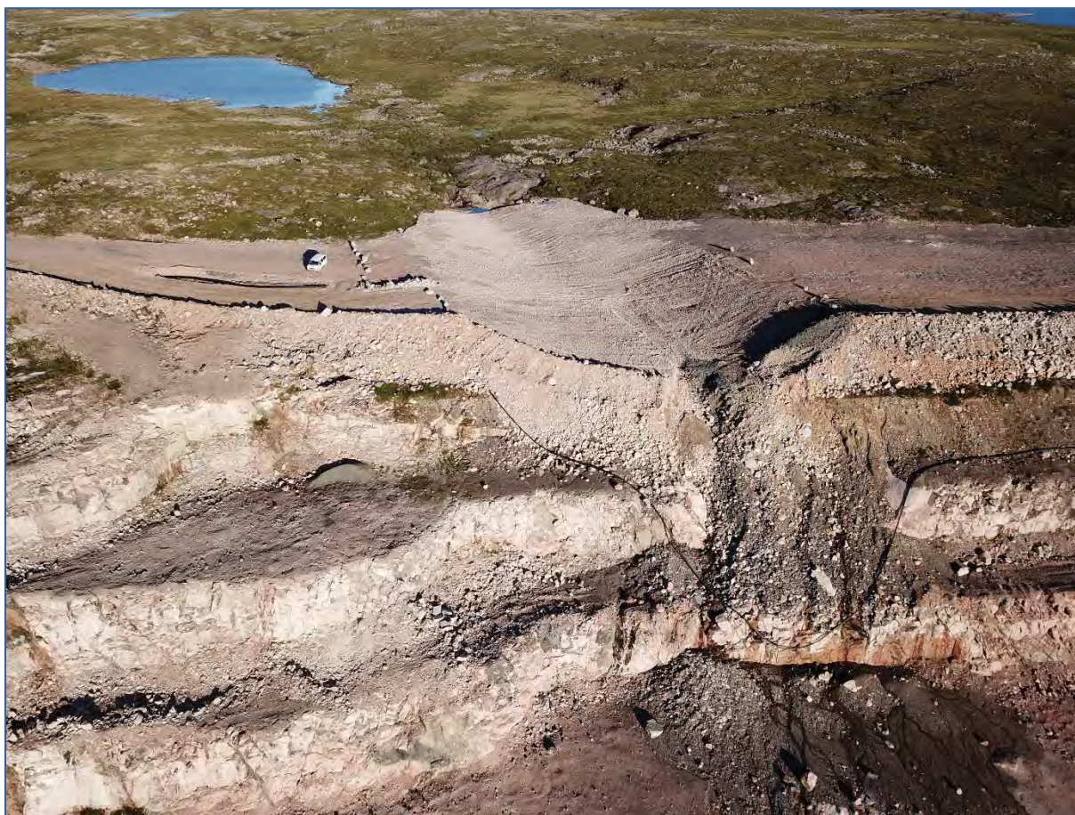
Photo 26: August 4, 2018 C1 Channel – Looking West, Erosion at Outlet into Open Pit.
