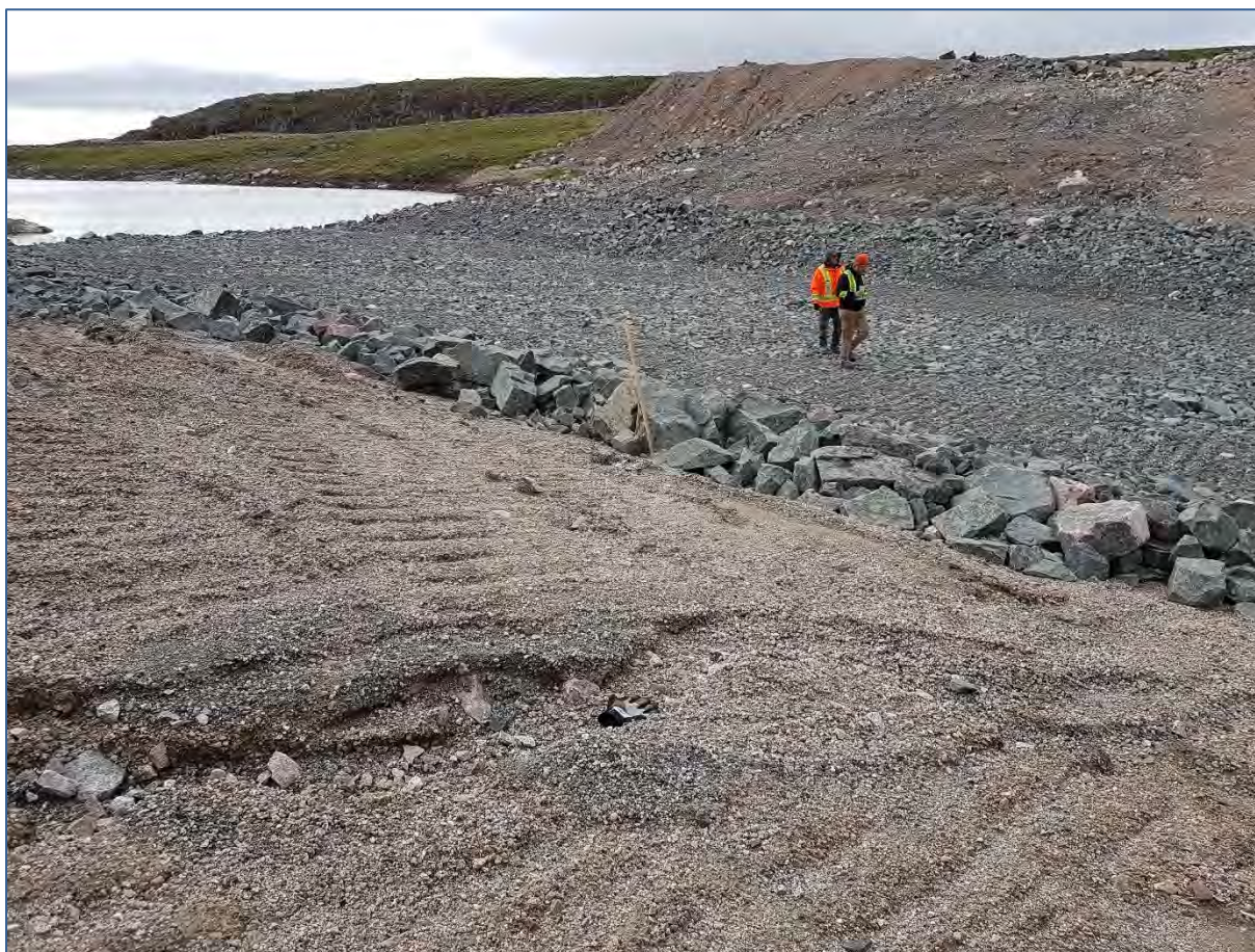
Photo 5: August 3, 2018 West Dam Breach – North Bank Erosion Gully.
