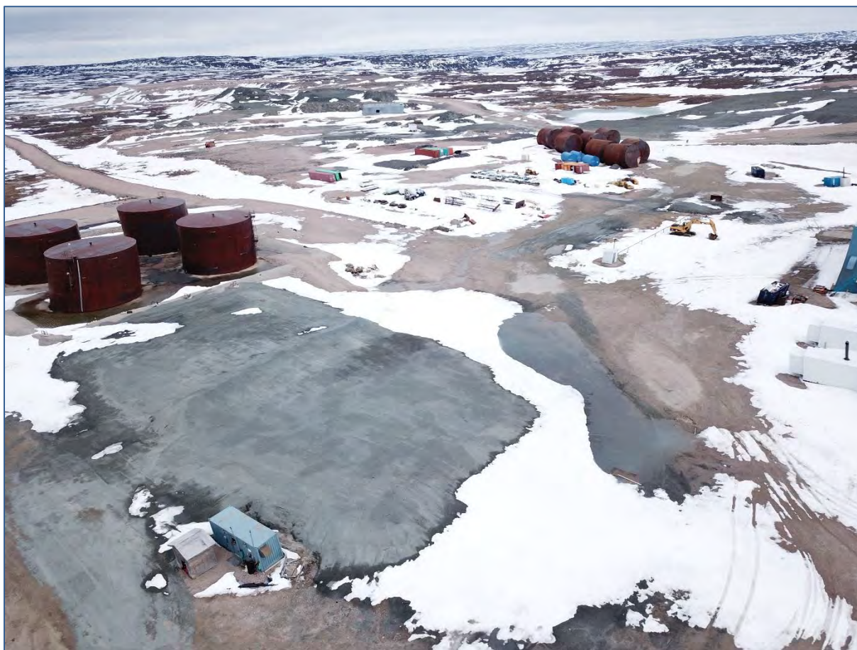
Photo 7: June 6, 2018 PHC Containment Cell Cover – Pre-Deficiency Repair (mound in middle).
