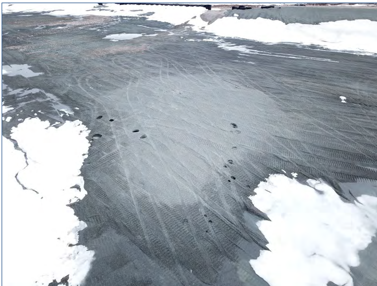
Photo 19: June 6, 2018 PKCA Cover, Southeast PKCA – Previously Identified Pot Holes.
