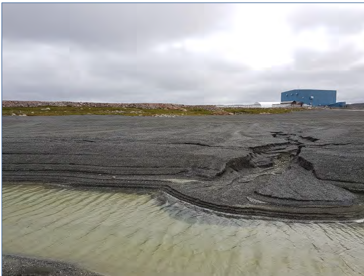
Photo 20: August 3, 2018 PKCA Cover, North PKCA – Outlet of Erosion Channel near ponded water adjacent Divider Dike A.
