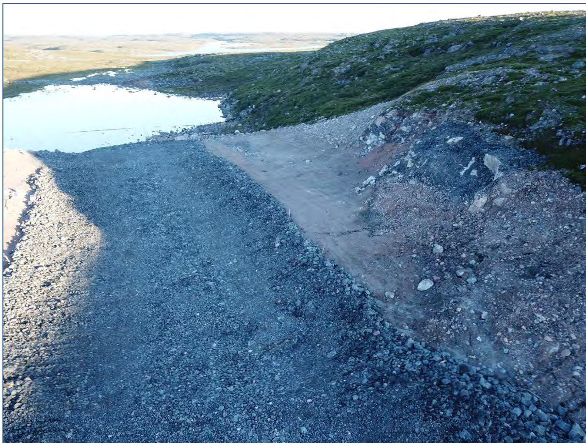
Photo 6: August 4, 2018 West Dam Breach – North Bank.
