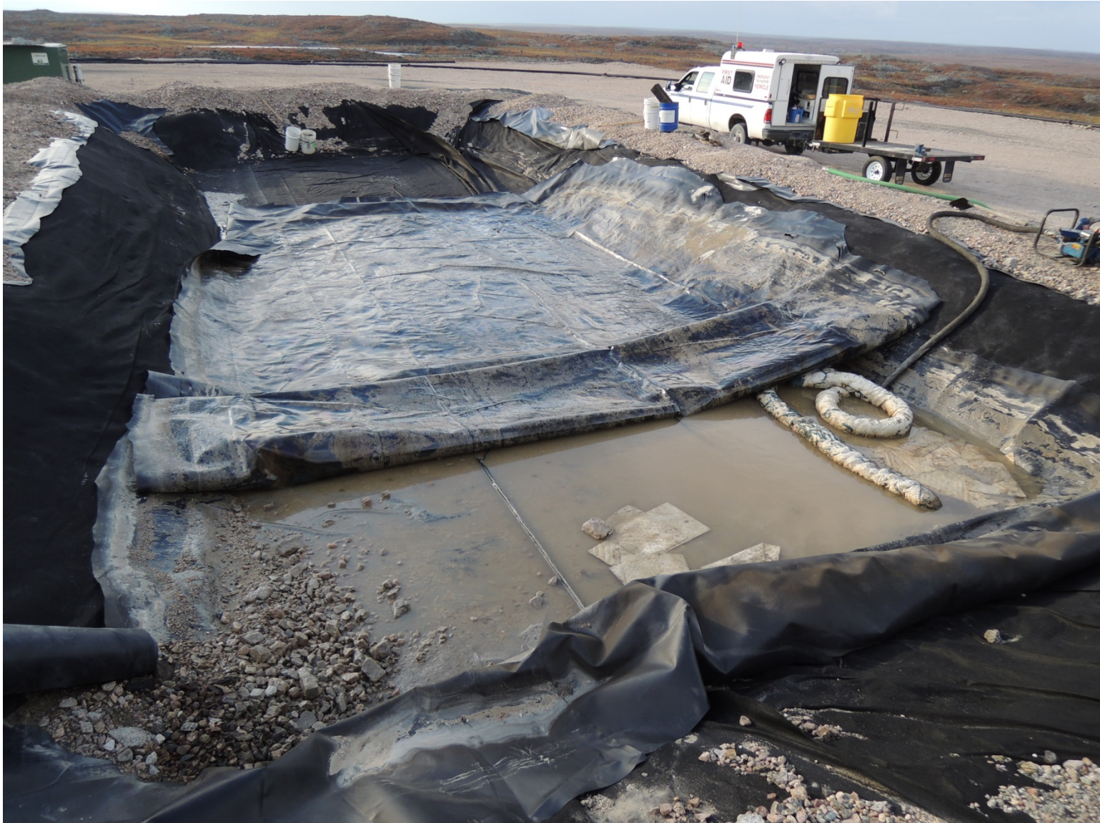
Picture #3 – Peeling Back Geomembrane to Consolidate Water/Gravel/Sludge
