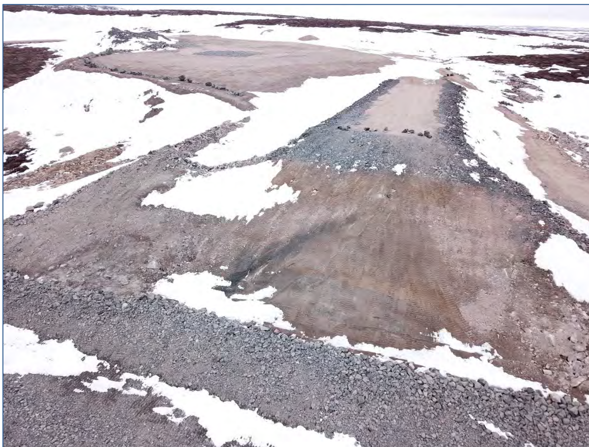
Photo 3: June 6, 2018 West Dam Breach – South Bank.
