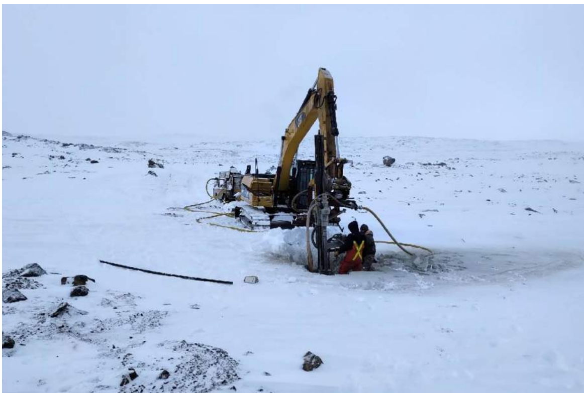
Photo 2 – Borehole Drilling Operation - Typical
