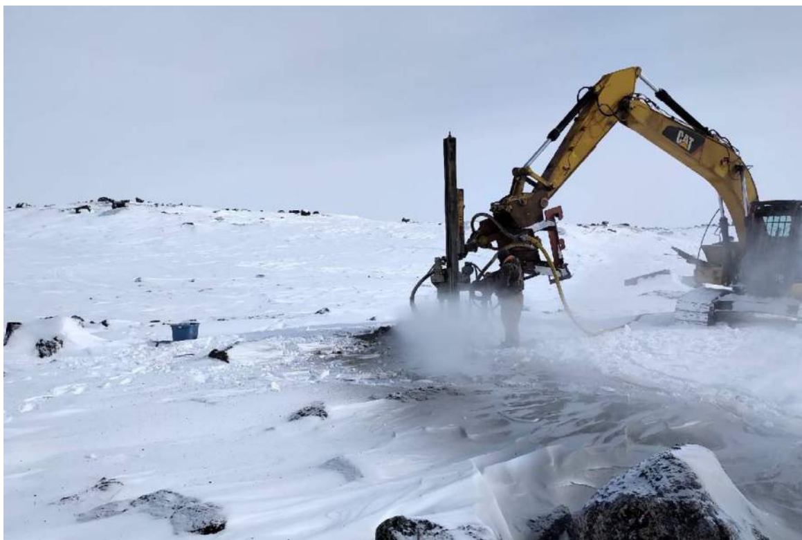
Photo 3 – Borehole Drilling Operation - Typical
