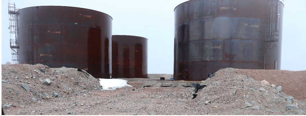
Photo 9: Phase II fuel tanks with breach in berm
