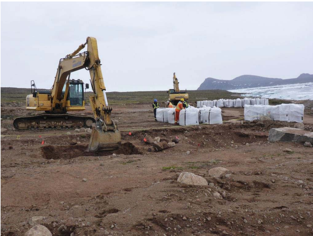
Figure 4. Excavating contaminated soil from APEC 12-3 and containerizing the soil at FOX-D Kivitoo.
