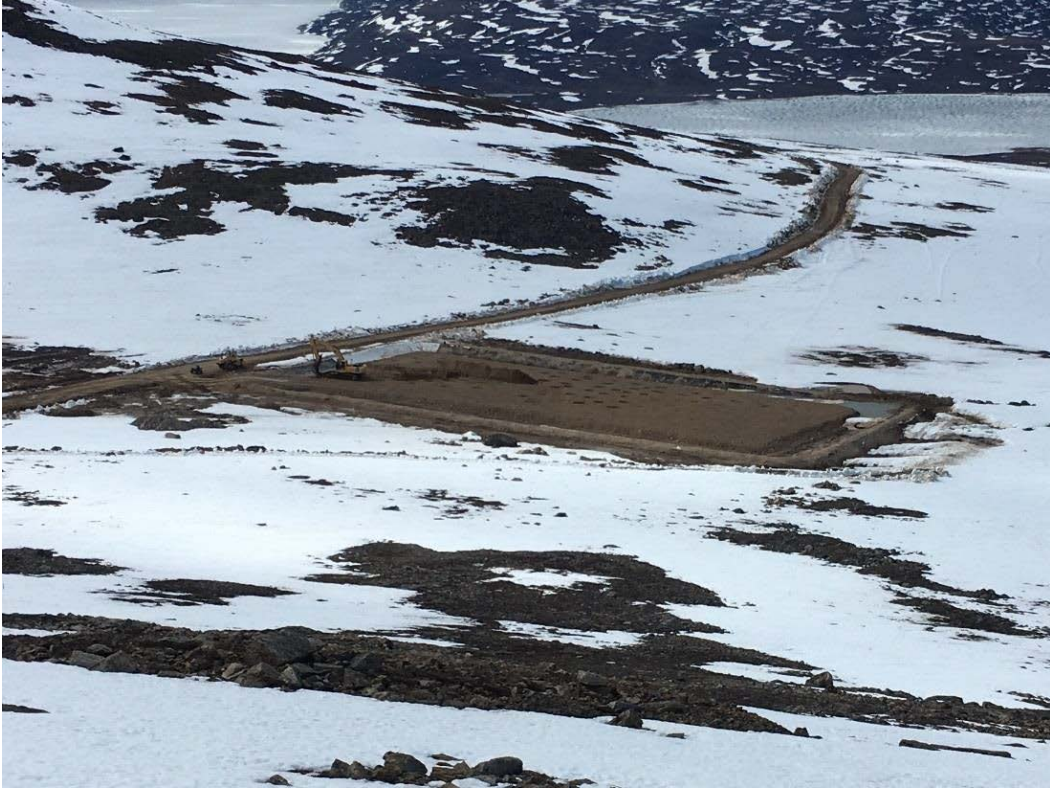
Figure 3. Consolidating remediated soil within the landfarm at FOX-D Kivitoo.
