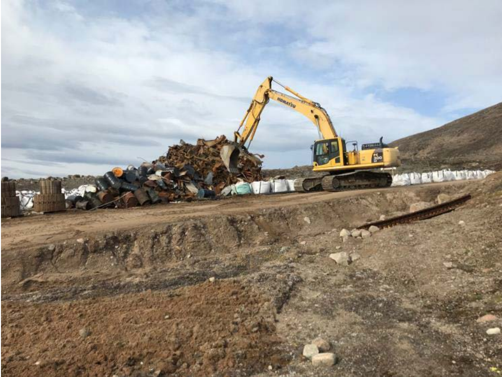
Figure 5. Sorting metal debris at the Temporary Storage Area for containerization at FOX-D Kivitoo.
