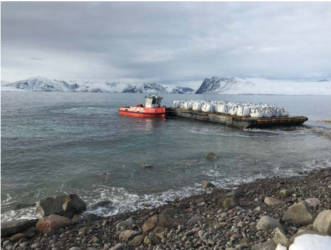
Figure 10. Barge transferring soil bags to the sealift at FOX-D Kivitoo.
