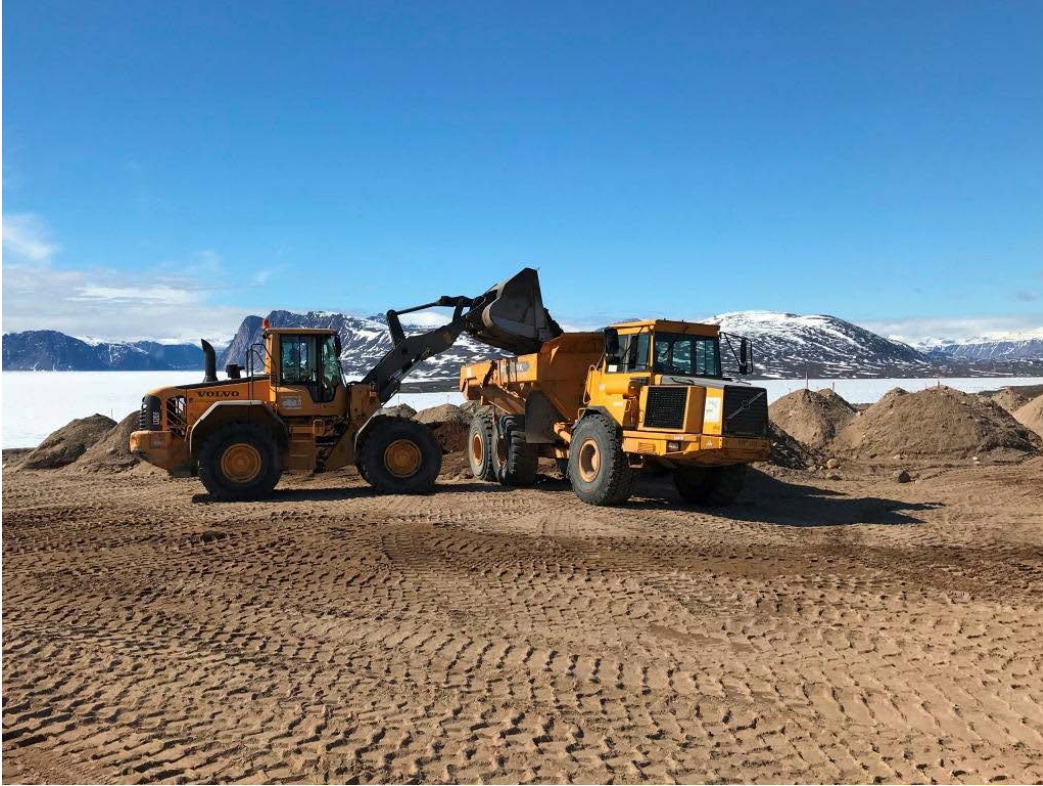
Figure 7. View of loader loading rock truck with material from clean stockpiles within the Material Processing Area for transport to APEC 11B – Lobe A at FOX-D Kivitoo.
