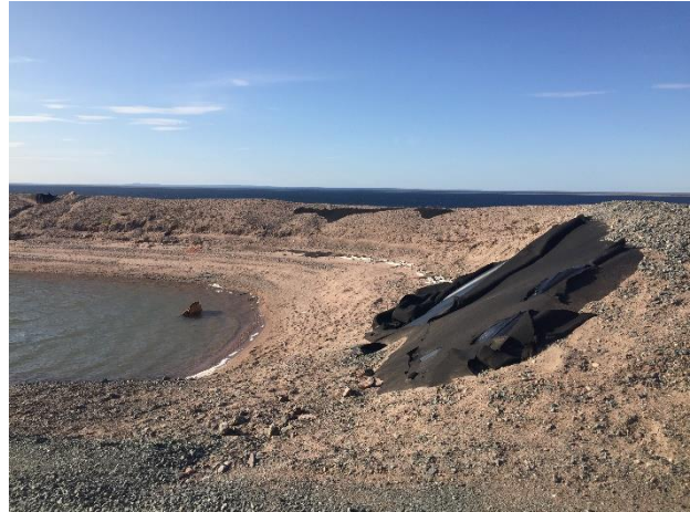
Photo 30: Exposed Liner at the Baker Lake Fuel Tank Farm
