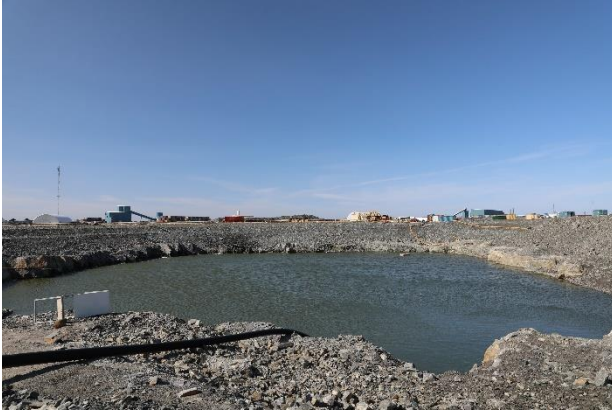
Photo 37: Saline water pond, which stores saline water from underground operations at the Meliadine Gold Mine Project.
