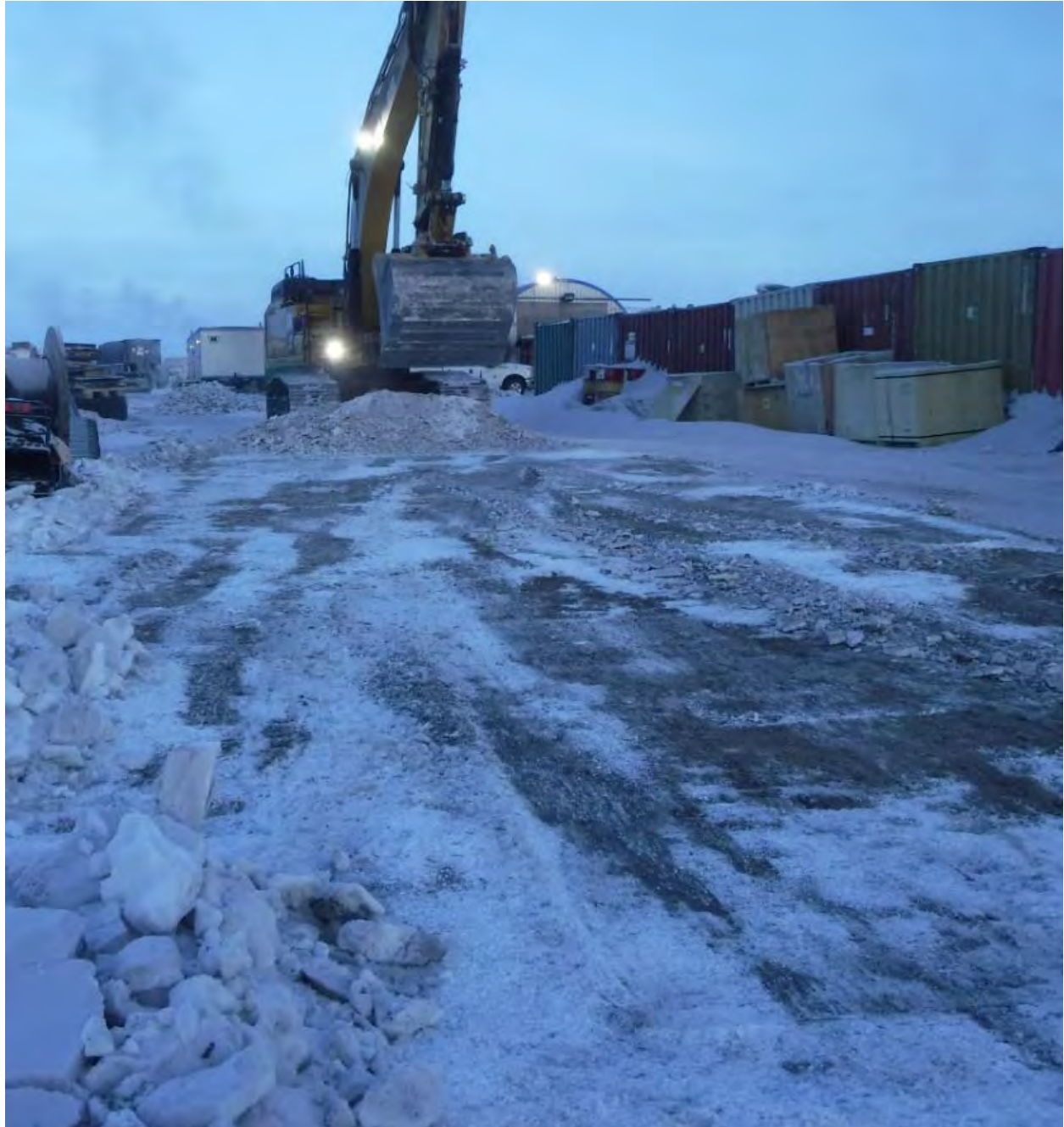
Photo 3 – Impacted ice/snow being scrapped up by excavator
