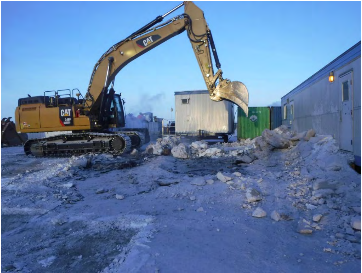
Photo 2 – Impacted ice/snow being scrapped up by excavator
