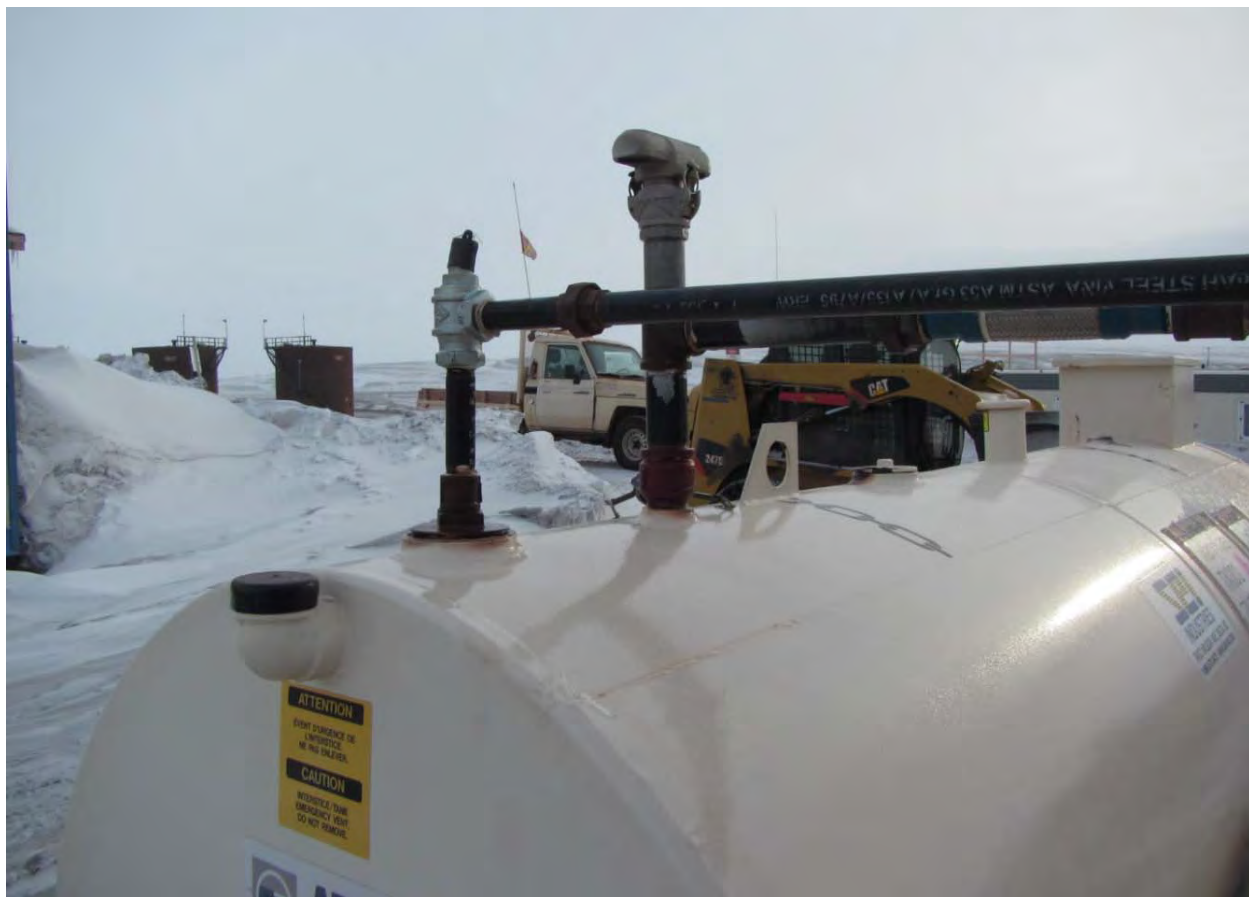
Photo 3. Vent pipe and whistle before retrofit
