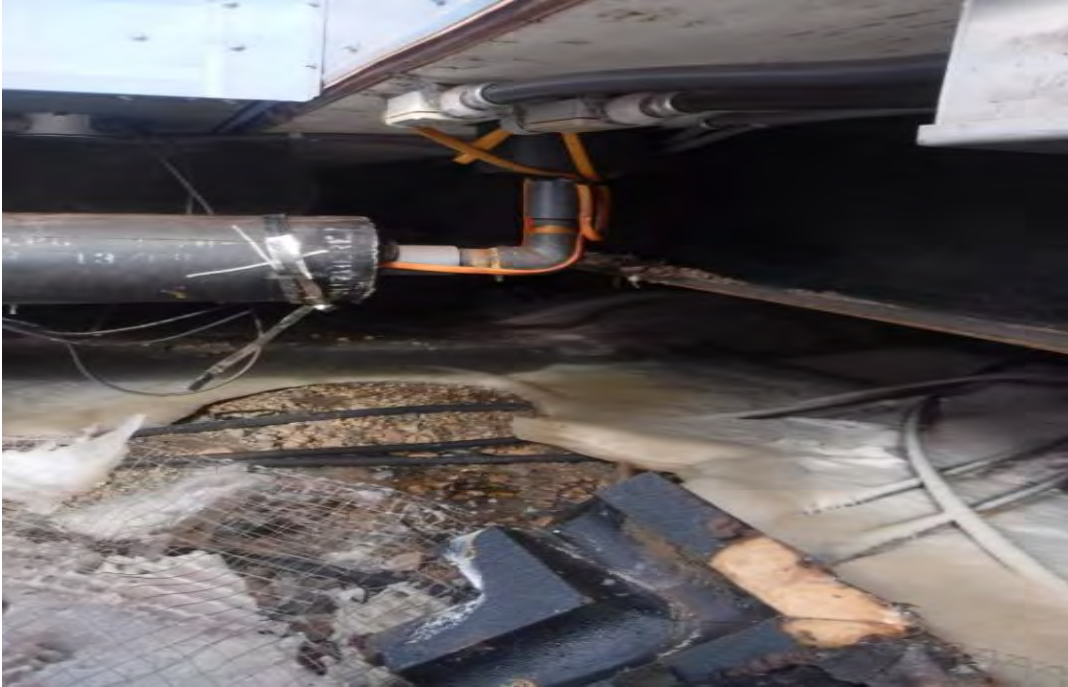
Photo 1. Discharge line before elbow repair
