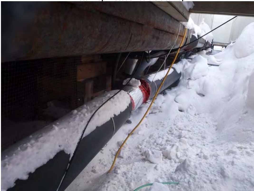
Photo 2. Gravity Drain Line after repairs completed
