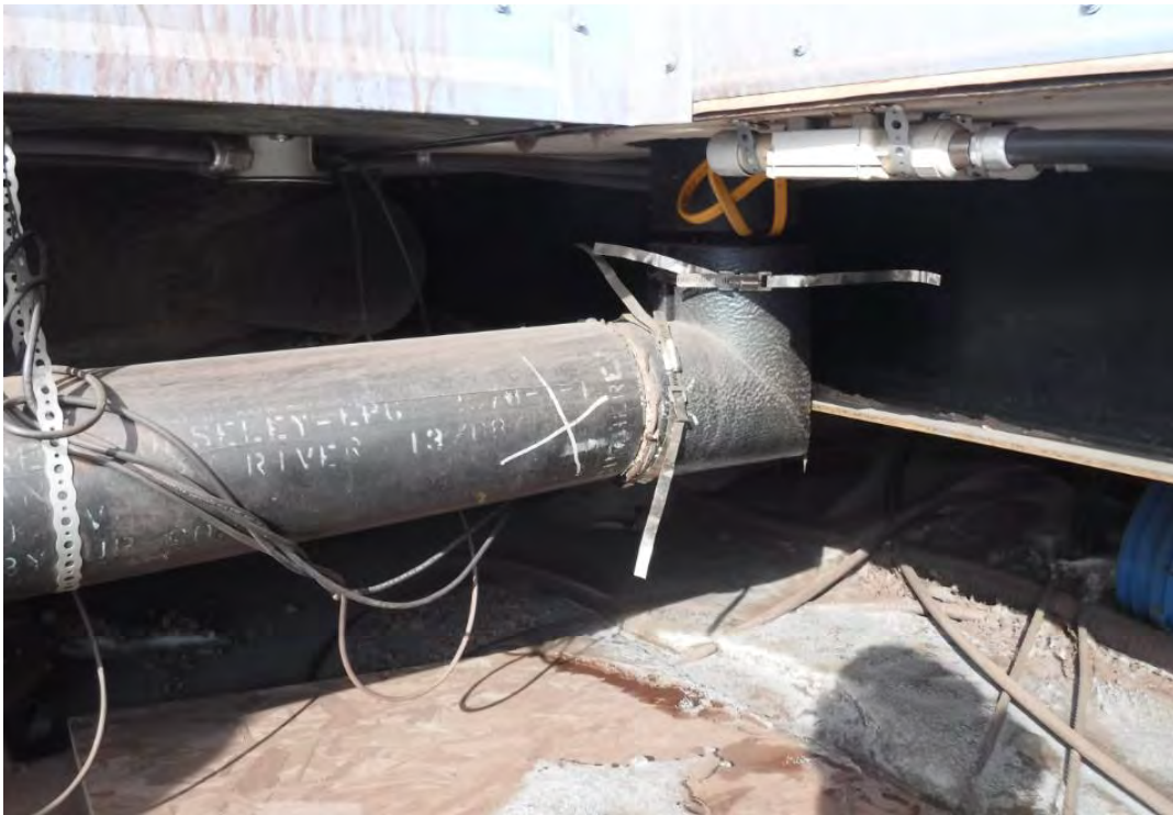
Photo 2. Discharge line following elbow repair
