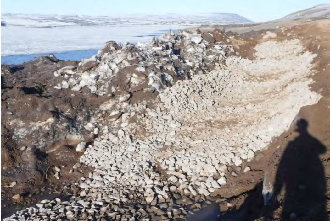
Photo 3. June 6, 2018: Bank armoring with riprap
