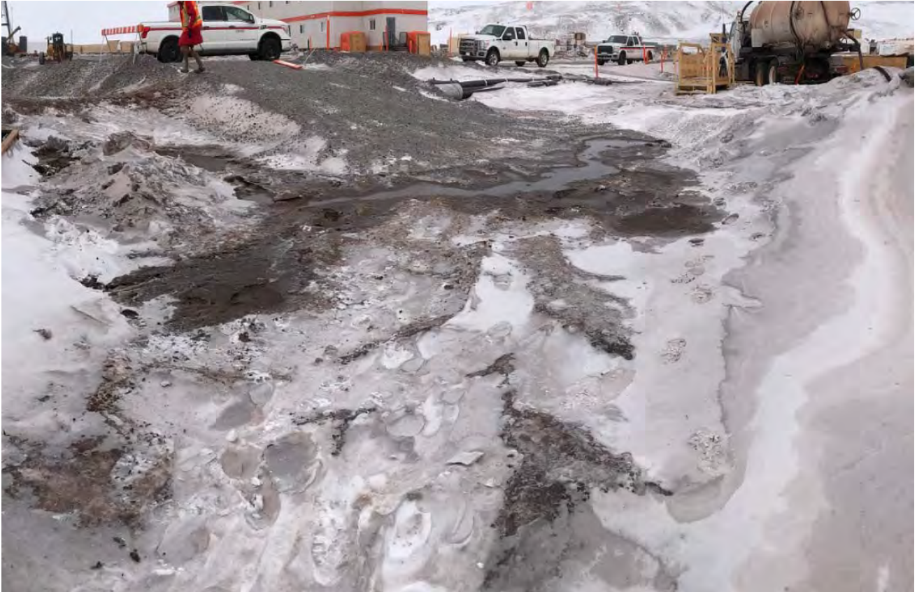
Photo 1. Overflow spill on ground surrounding the WWTP
