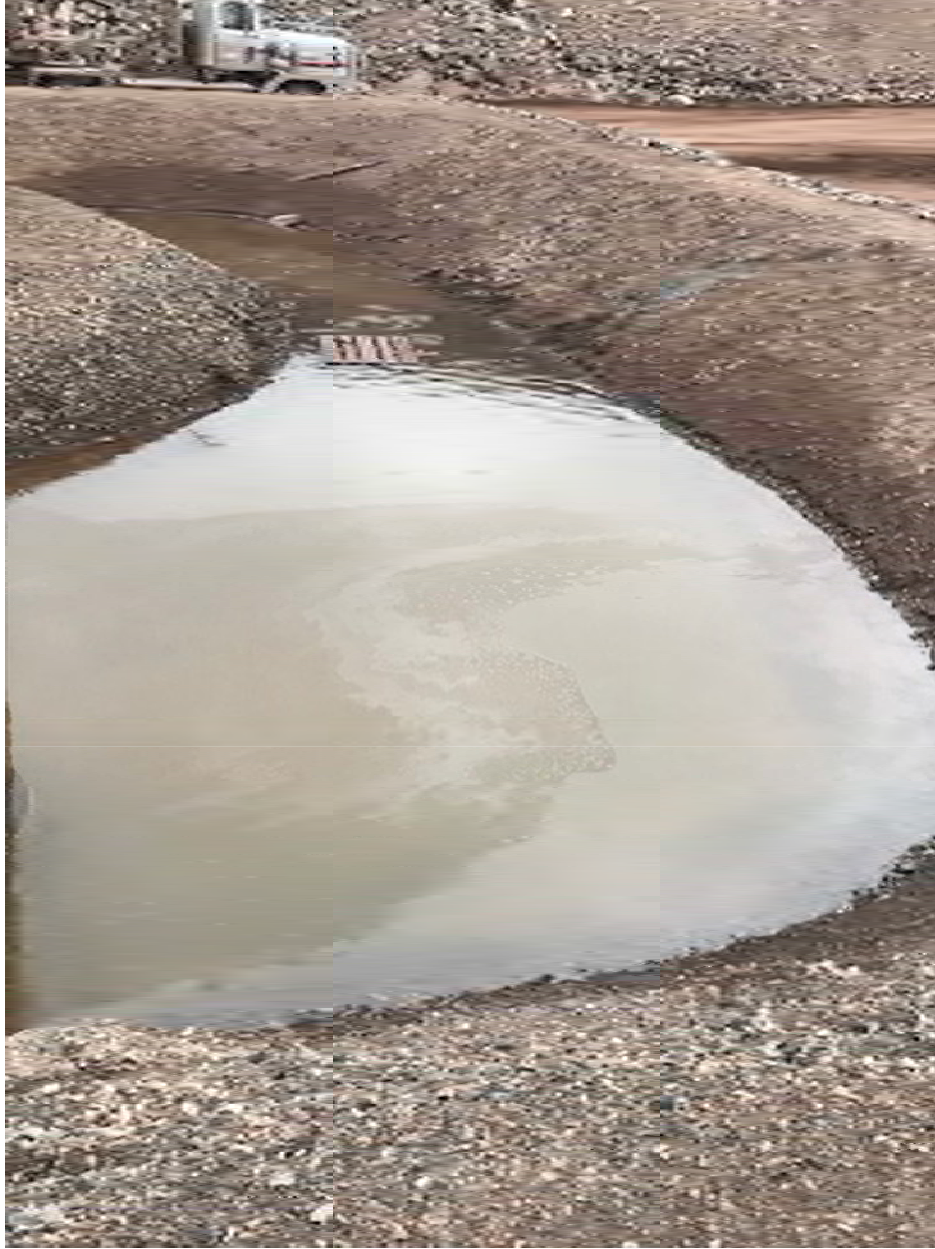
Photo 2. Spill contained within fuel mod berm.
