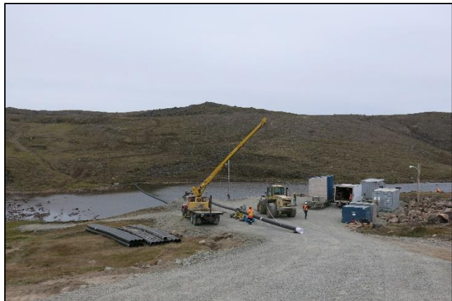
Water pipeline being assembled to carry water from Niaqunguk River (Apex River) to Lake Geraldine Reservoir (#5(d) in Itinerary above)
