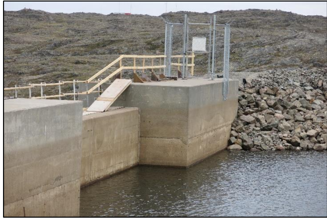
Lake Geraldine Reservoir spillway showing the current water level relative to the level required to fill the reservoir (#3 (b) in Itinerary above).
