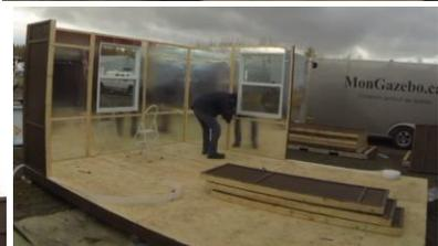
Complete this step by installing the Me6 exterior door with V2 screws around the door (sides and floor, interior and exterior). You must add the handle provided (refer to the instructions on the packaging).
