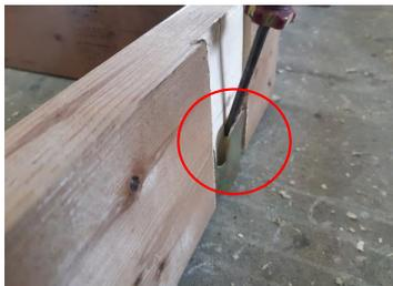
Screw the floor panels together using V3 screws.
