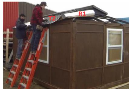
Put outside R3 tape at the 4 corner joints before putting the T5. Then fix the ridges (T5) in each corner to close the joint of the sheets at the four corners. Screw the ridge directly into the sheet metal by putting 2 min. Sheet metal screws (V4) on each side (and NOT centered on the bend 'as the sheet is embossed).
