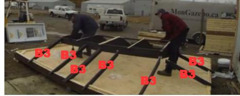
Now secure the B4s from the corners of the roof contour to the corners of the pinion. (with V3).
