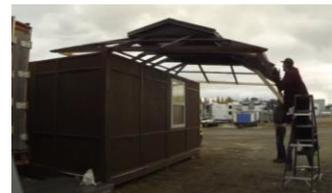
**\* IMPORTANT: ALWAYS screw up (from the inside of the top of the walls to the roof structure) as the screw heads will be easily accessible to change a section of wall as needed in the future. Otherwise you will have to remove sheets of sheet metal to make this same change of wall section.**
