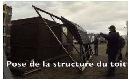
Change your position to pick up the corners that remained on the ground and lift them by sliding the structure on the top of the walls. Place the roof structure (parts B1) exactly on the outside walls and screw generously with V2 (see note below) \* with the outside walls.
