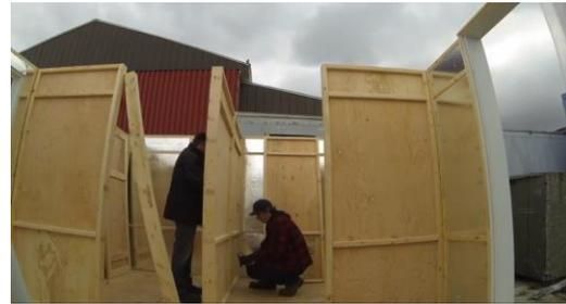
Screw (with V2) the pieces P1 vertically on the sides where the doors of the 3 openings will close (put notch towards the inside of the rooms / entry as on schema). Then screw the pieces P2 in the top of the frames and the P3 in the bottom (as on diagram) always with screws V2.
