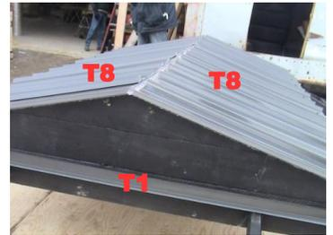
**WARNING:** the screws must be put on the embossing of the sheet (and NOT in the hollow).
