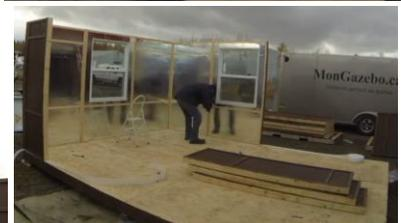
Complete this step by installing the Me6 exterior door with V2 screws around the door (sides and floor, interior and exterior). You must add the handle provided (refer to the instructions on the packaging).
