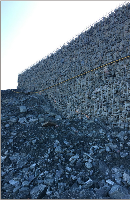
Photo 5: Crusher Ramp - MSE wall
