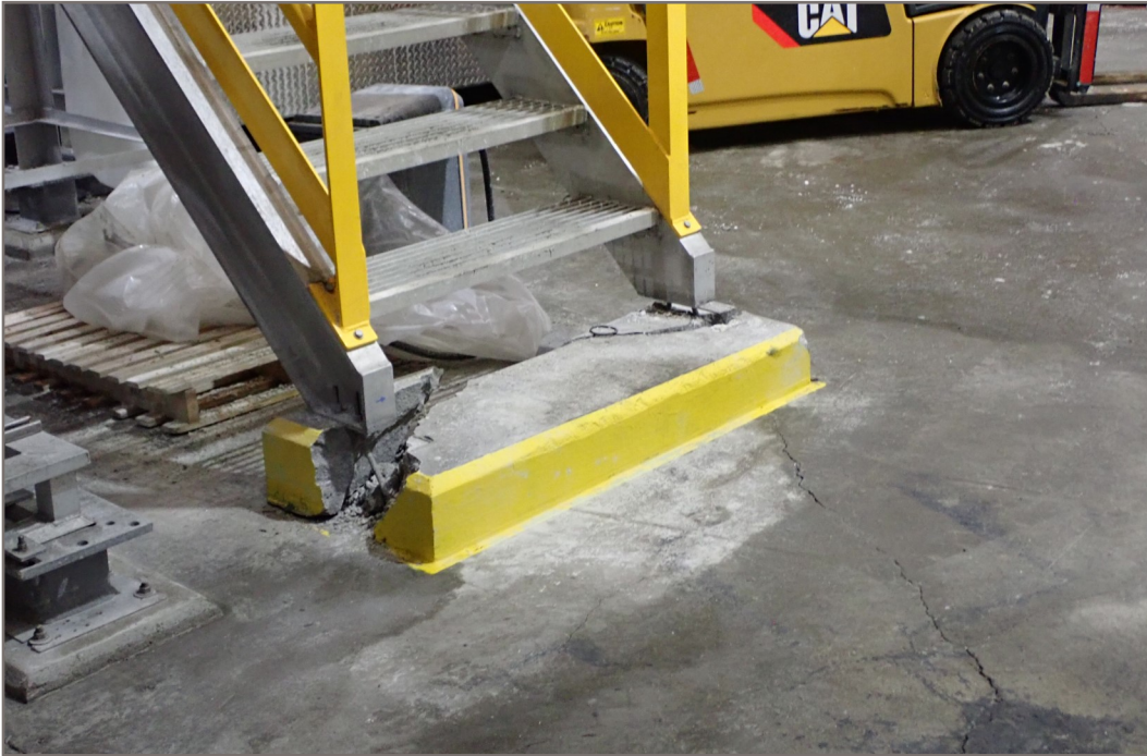
Photo 11: SWTP Distress due to floor movement
