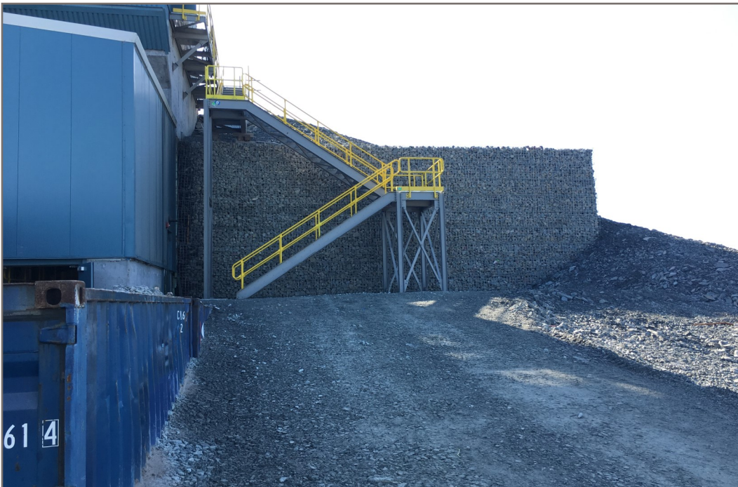
Photo 6: Crusher Ramp - MSE wall
