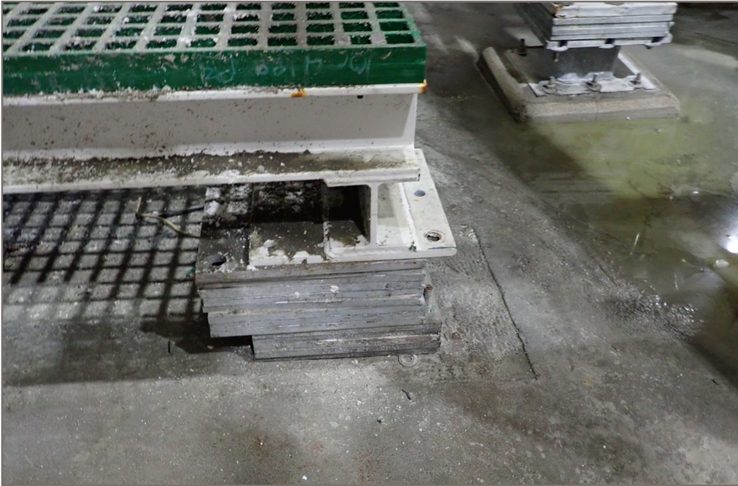
Photo 9: SWTP Shims to level the plant
