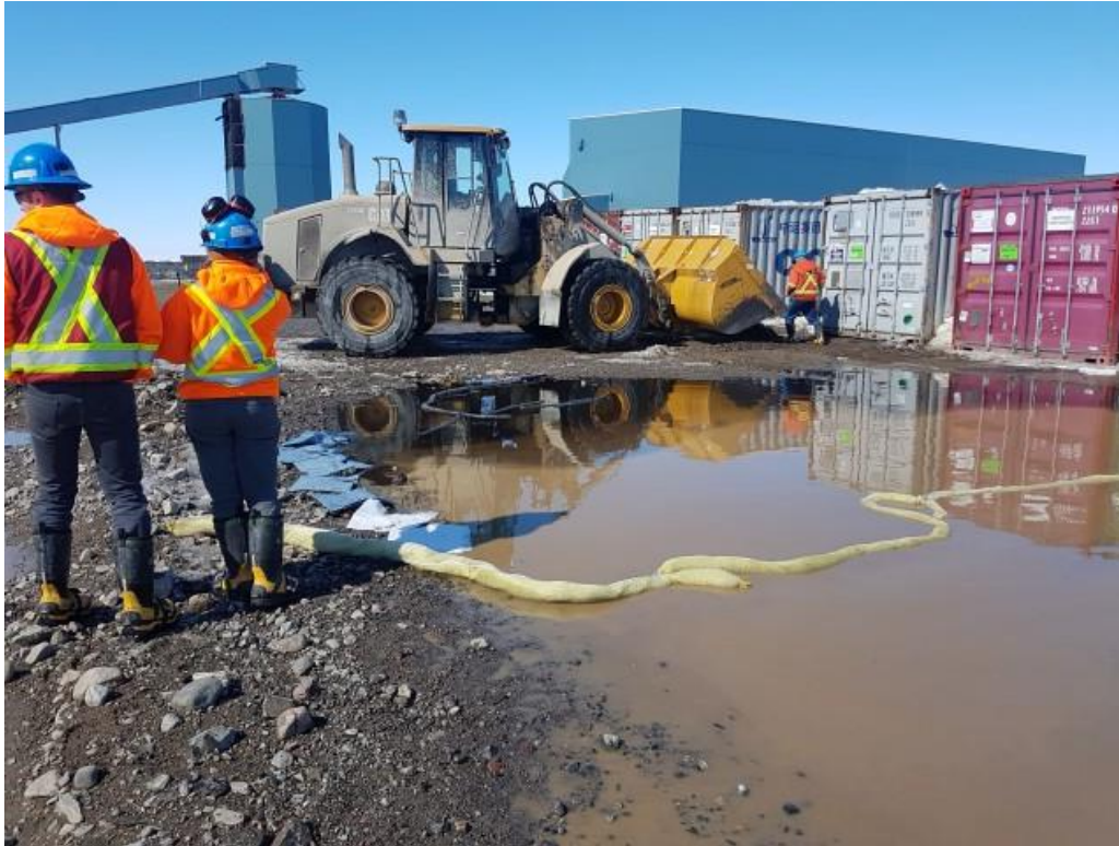
Figure 2: Waste oil contained by hydrocarbon boom at hazmat laydown.
