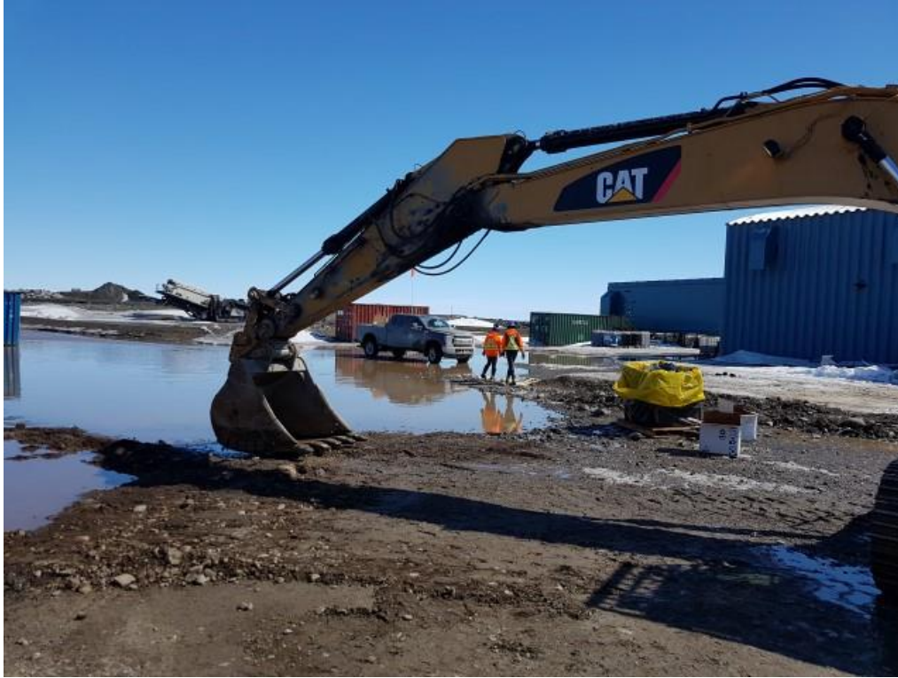
Figure 5: Sump used to collect floating waste oil was backfilled.
