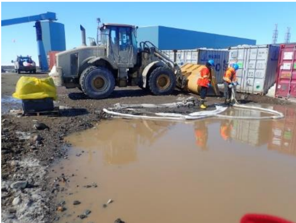
Figure 4: Loader used to transport waste oil contaminated road base to landfarm.
