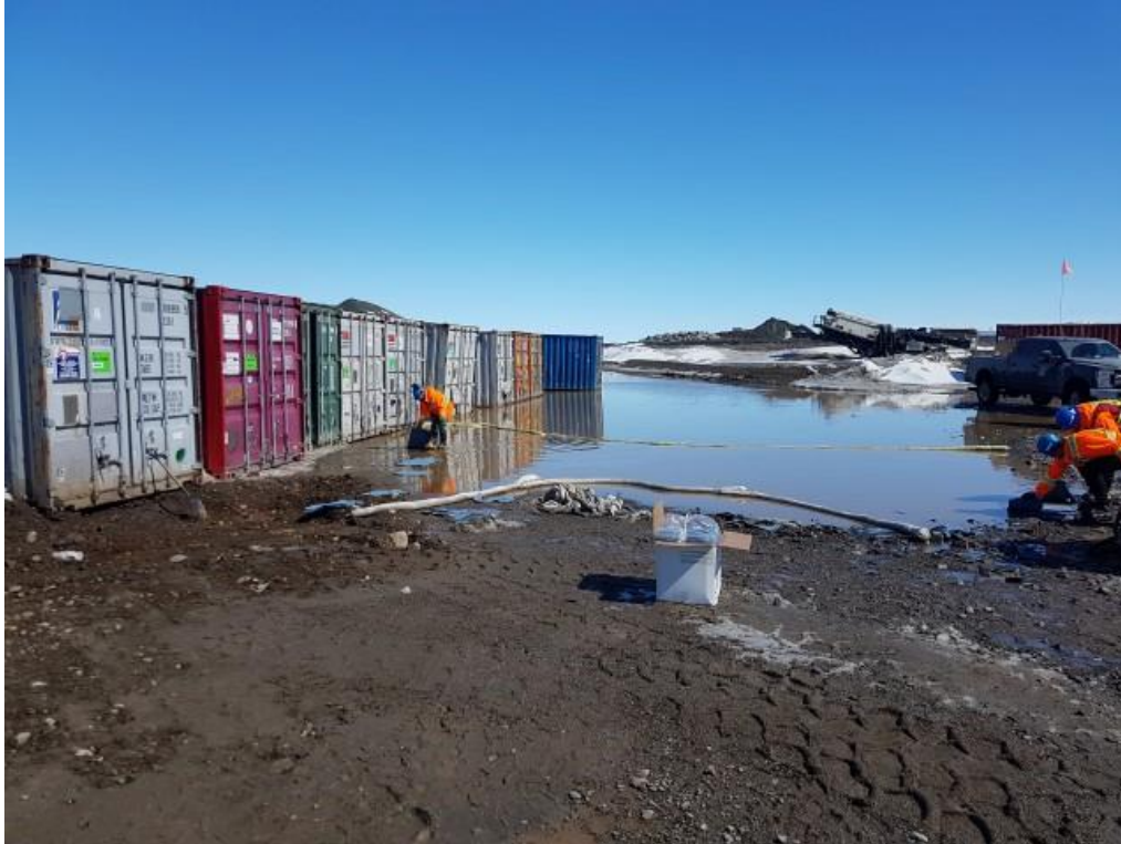
Figure 3: Waste oil was absorbed using spill response supplies.
