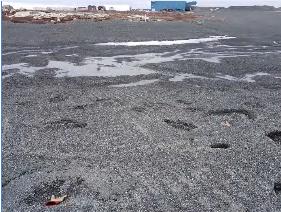
Photo 23: June 18, 2019 PKCA Cover, Looking N – View of potholes.
