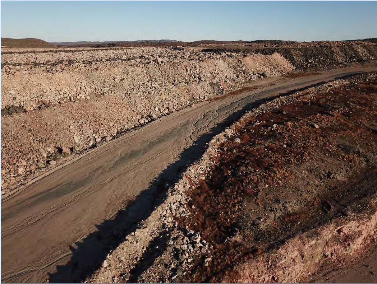
Photo 50: Sept. 10, 2019 Road Section – Fall Photo of Main Road section by N pit access with drainage erosion.
