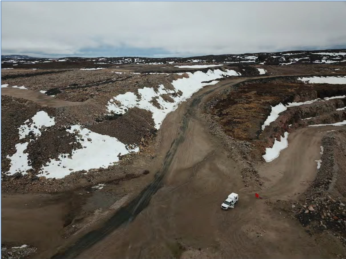
Photo 49: June 18, 2019 Road Section – Photo of Main Road section by N pit access with drainage erosion, UTM coordinates 12 W N478414 E7319738.
