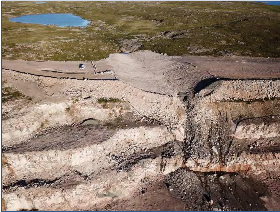
Photo 27: August 4, 2018 C1 Channel, Looking West – 2018 photo of erosion at outlet into Pit.
