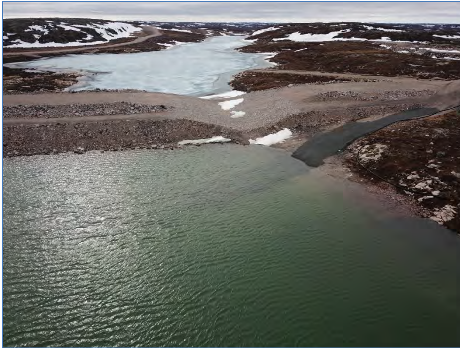
Photo 13: June 18, 2019 PKCA Cover, Looking W – Ponded water covering access road.
