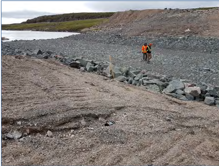
Photo 3: August 3, 2018 West Dam Breach – 2018 photo of erosion gully on North Bank.
