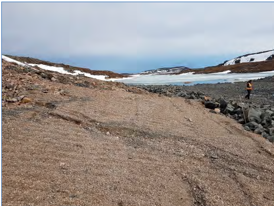
Photo 4: June 17, 2019 West Dam Breach – No significant change in erosion gully on North Bank.
