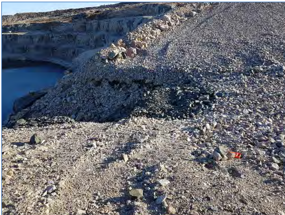
Photo 35: Sept. 10, 2019 C1 Channel, Looking E – Eroded section into Open Water @ 6.3 m in Fall.
