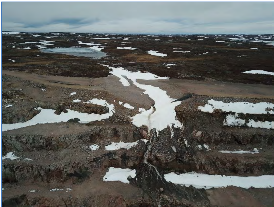
Photo 28: June 19, 2019 C1 Channel, Looking W – Erosion at outlet into Pit.
