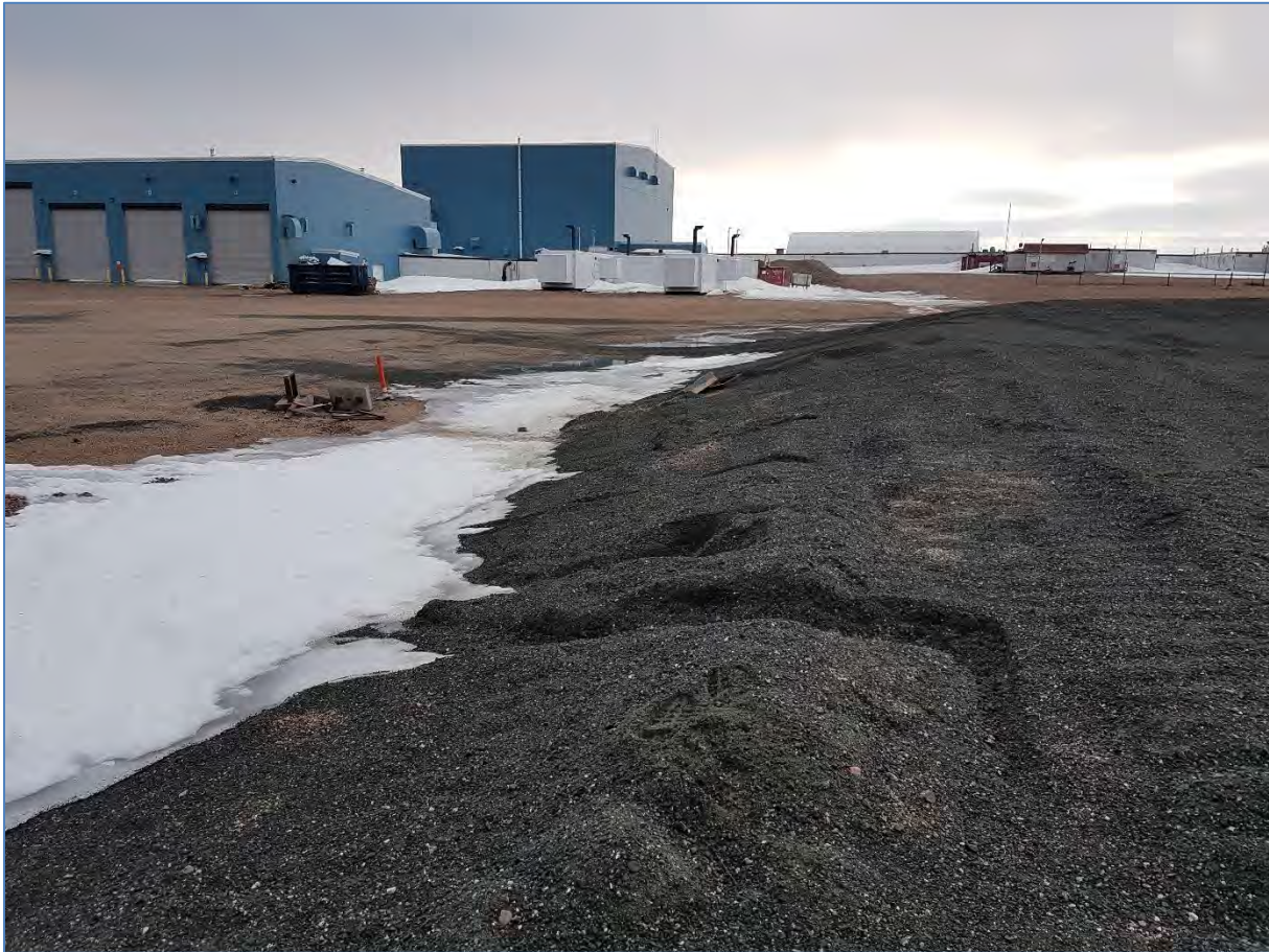
Photo 10: June 17, 2019 PHC Containment Cell Cover, Looking S – Drainage erosion on East Bank.
