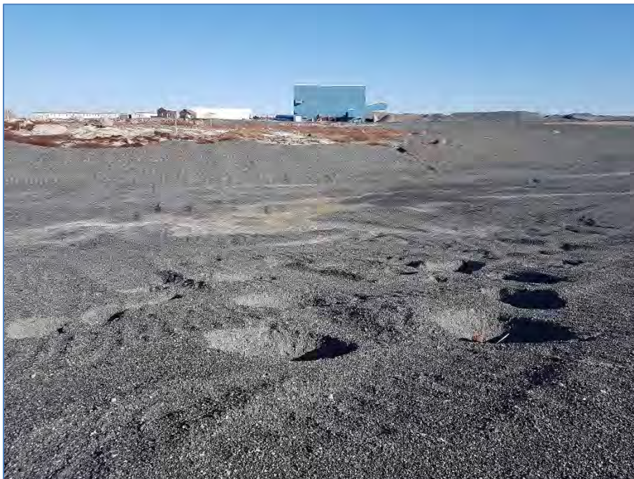
Photo 24: Sept. 11, 2019 PKCA Cover, Looking N – Fall view of potholes.
