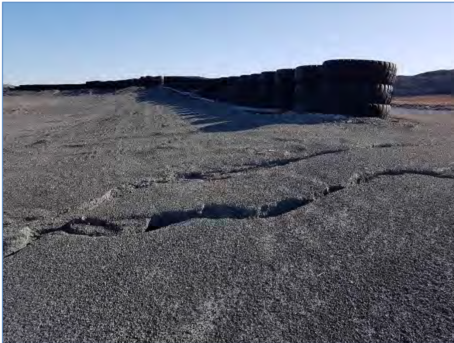
Photo 18: Sept. 11, 2019 PKCA Cover, East PKCA – Some erosion from drainage into PKCA.
