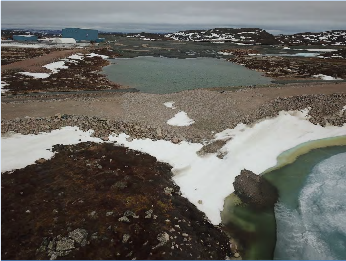
Photo 25: June 18, 2019 Divider Dike A, Looking E – Dike and energy dispersion ramp.
