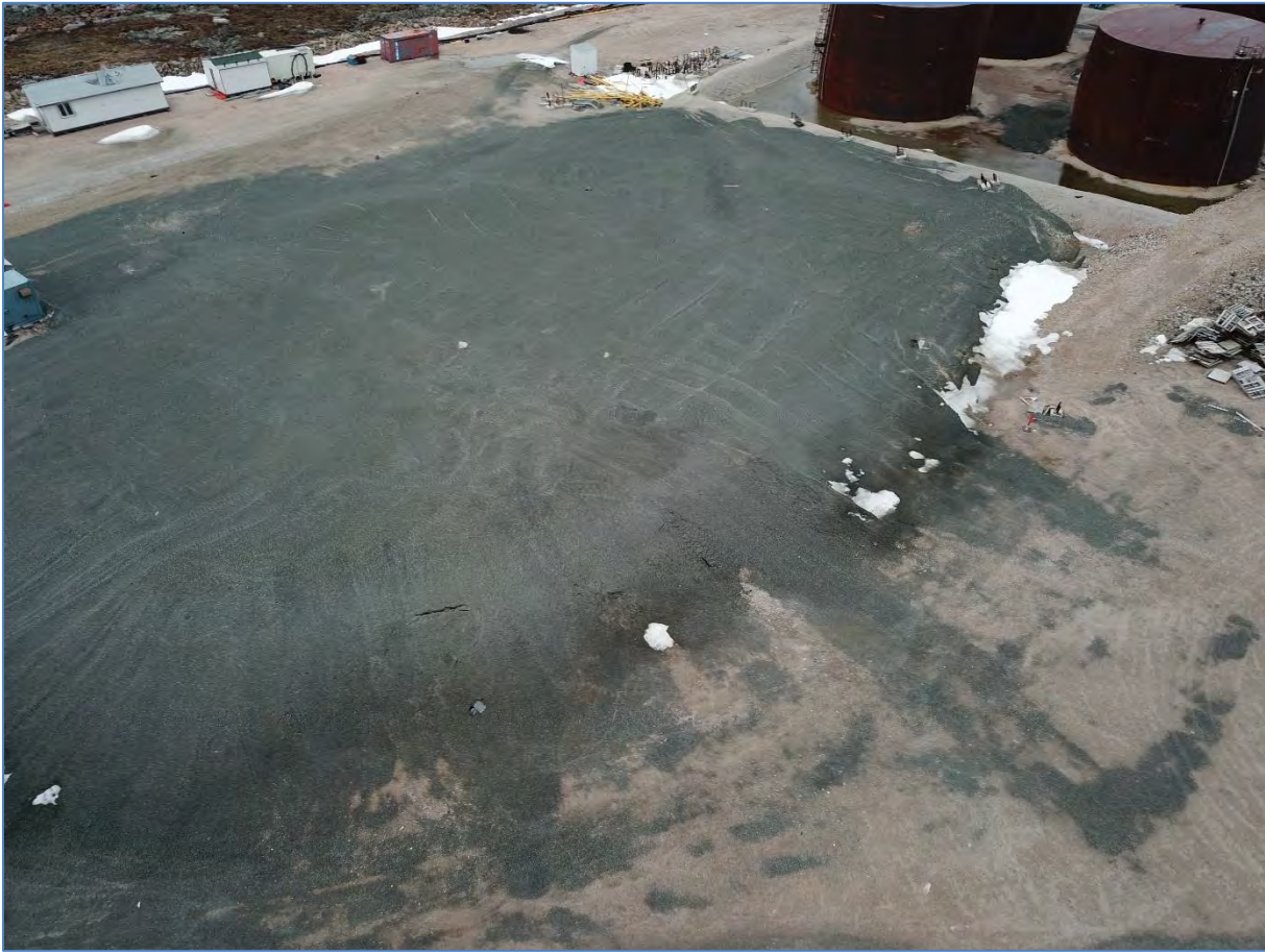
Photo 7: June 18, 2019 PHC Containment Cell Cover, Looking N – Some settlement and drainage erosion along East Bank.
