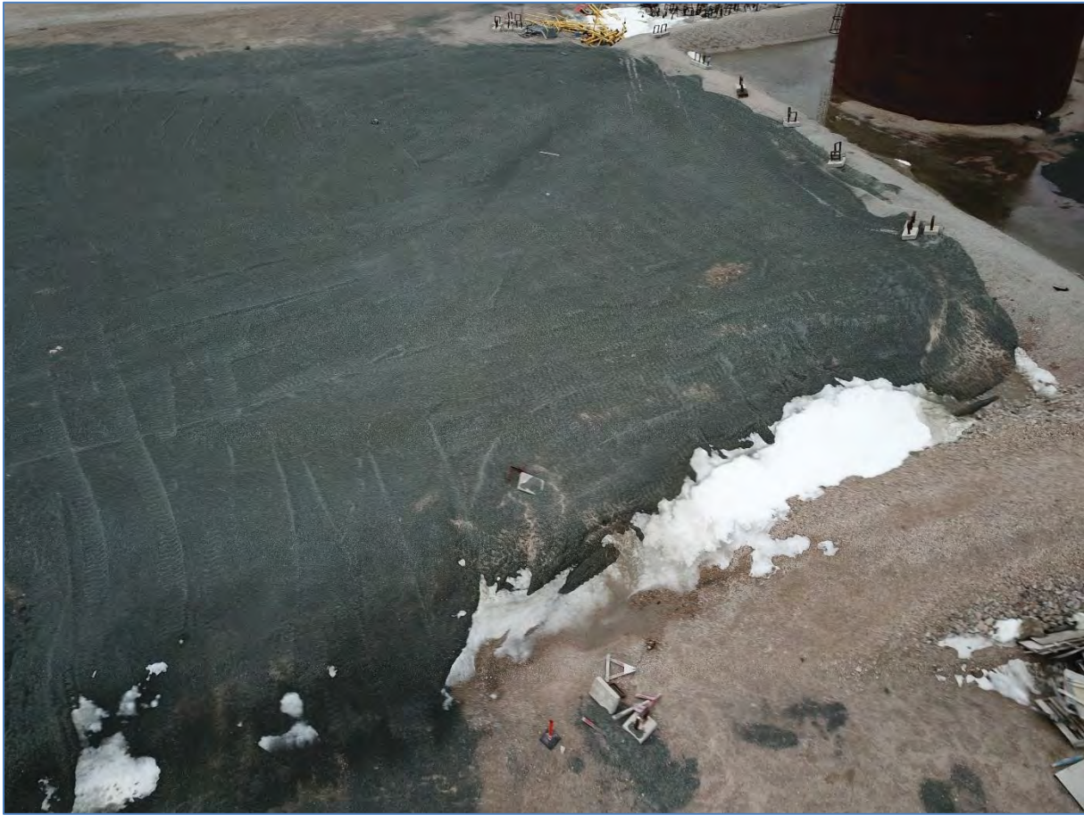
Photo 8: June 18, 2019 PHC Containment Cell Cover, Looking NW – Drainage erosion in north corner of East Bank.
