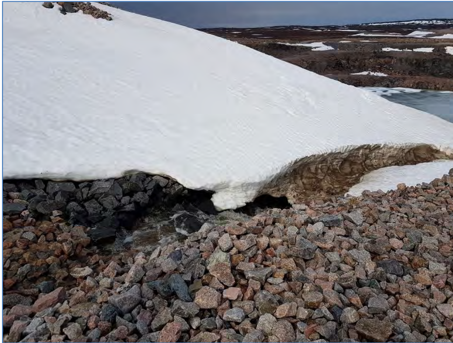
Photo 34: June 17, 2019 C1 Channel, Looking E – Water runoff under snow into Open Pit.
