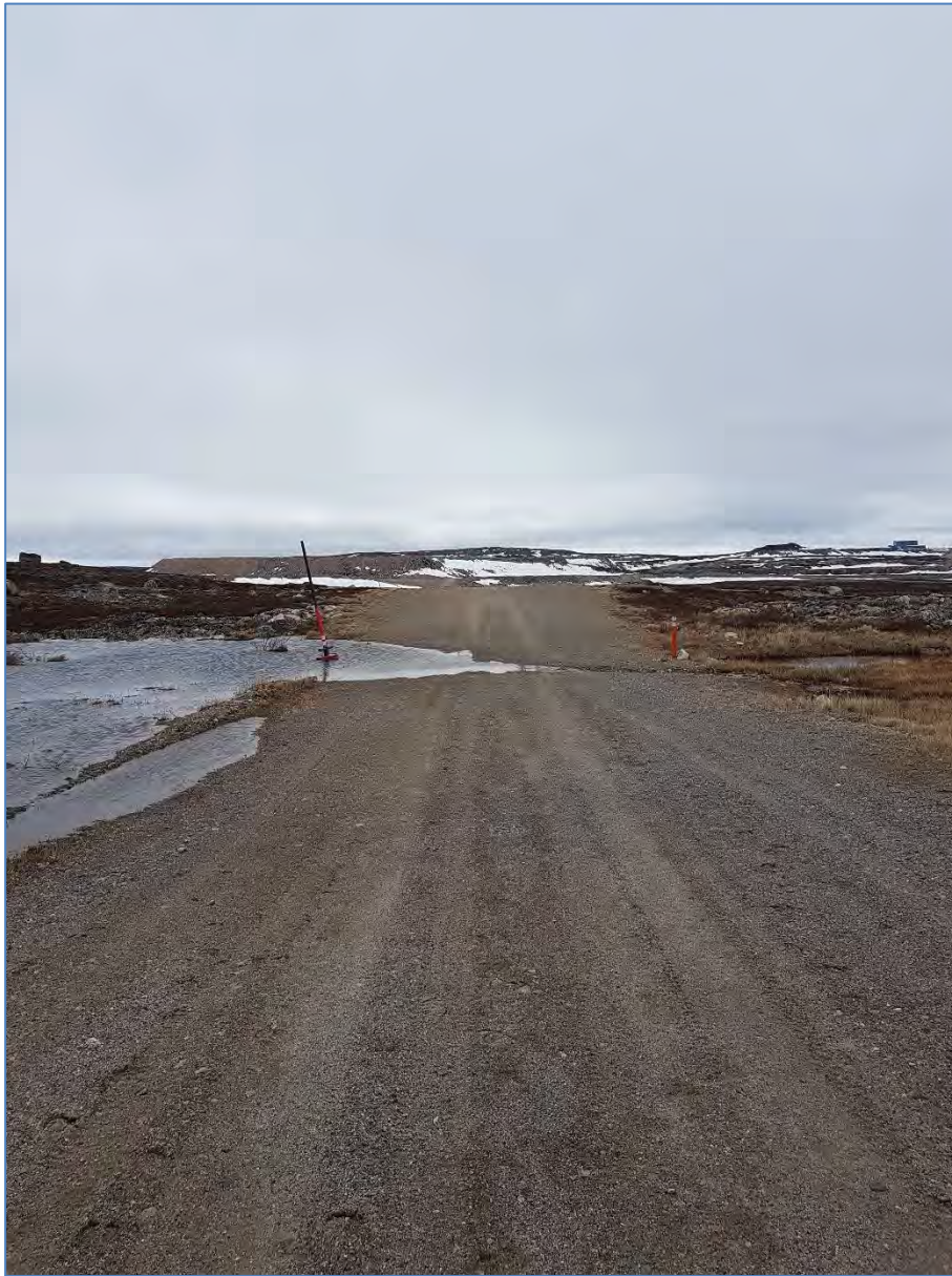
Photo 48: June 18, 2019 Road Section – Photo of partially flooded Main Road section between HWTA and Open Pit, UTM coordinates 12 W N478868 E7320754.
