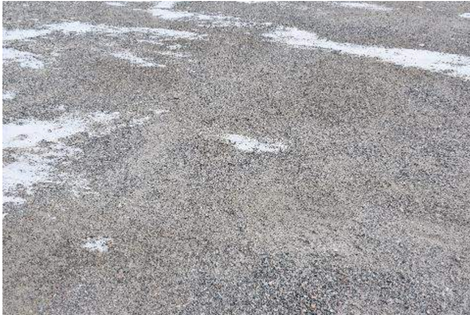
Photograph No. B3 Raveled, uneven ground of the apron, looking north
