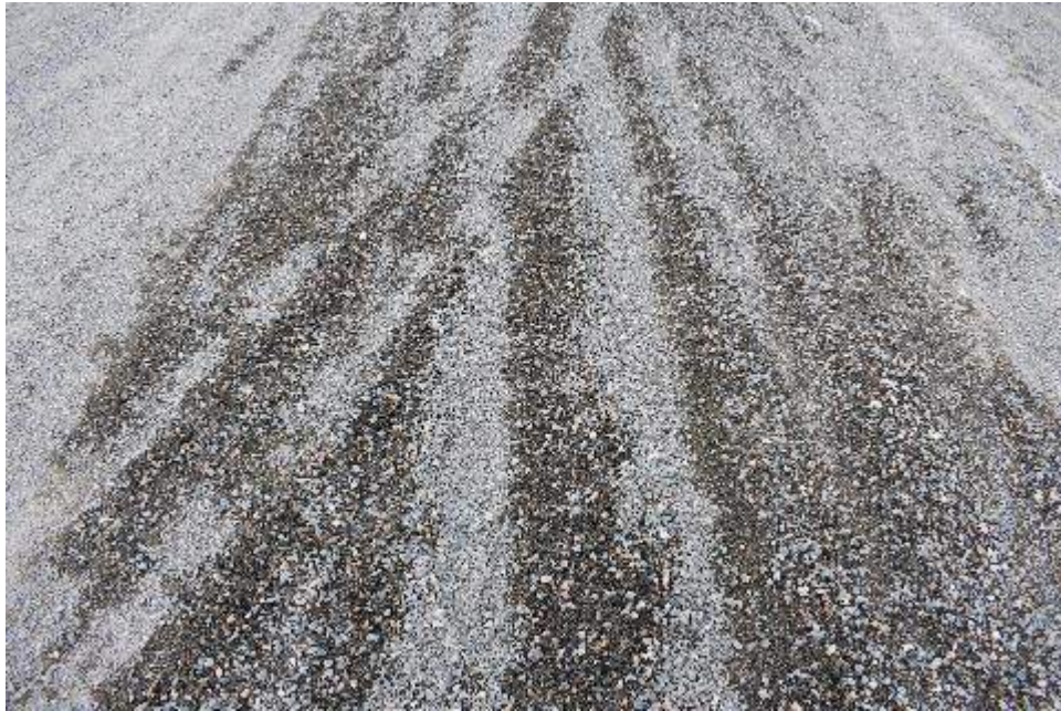
Photograph No. B11 Raveling at the center of the runway, looking north
