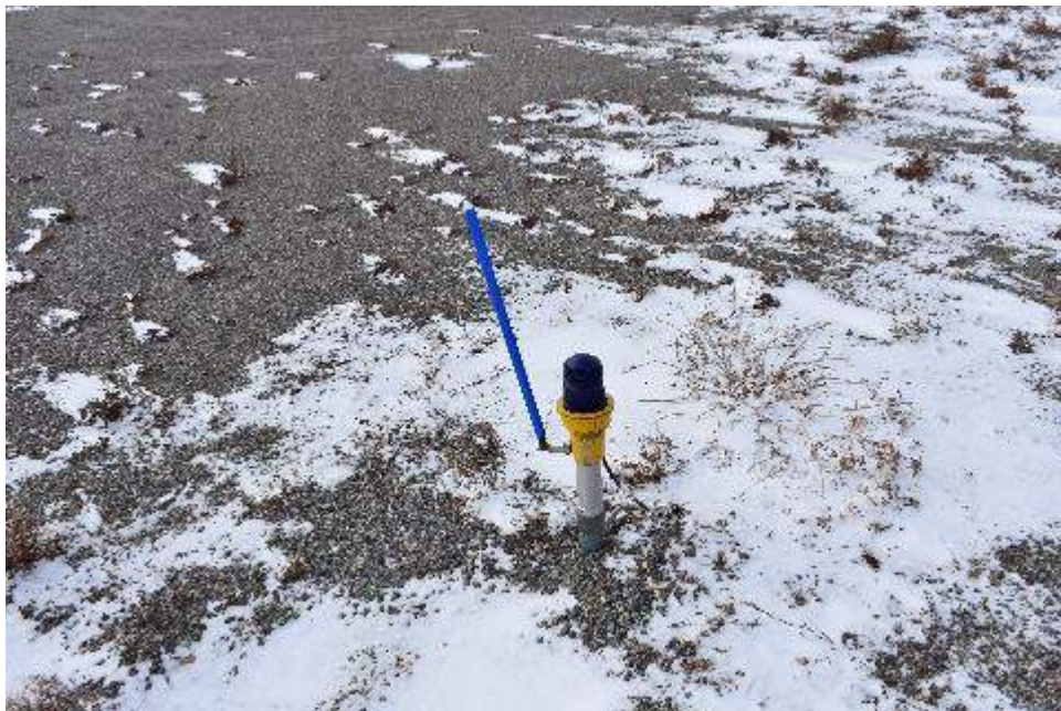
Photograph No. B6 Apron lights in good condition with snow markers attached, looking northeast
