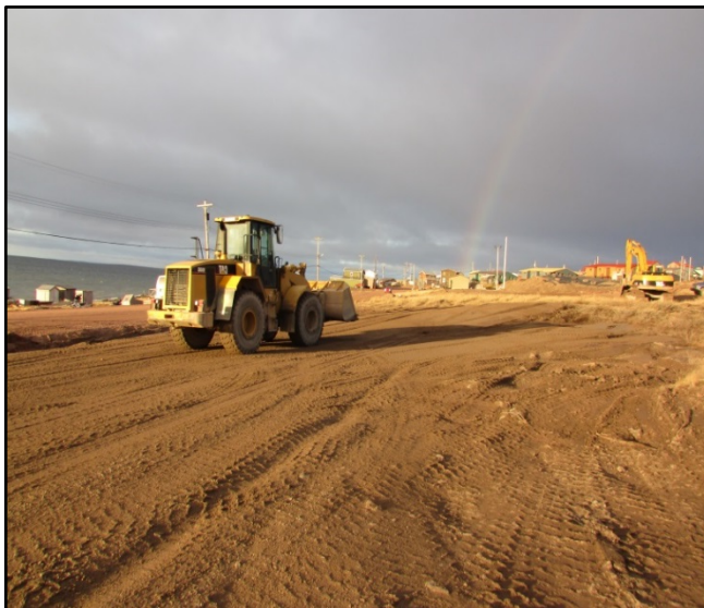
Photo 3 – Hot Spot TP 33 infilled and final graded
