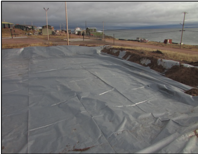
Photo 1 – Liner installed over base and berms
