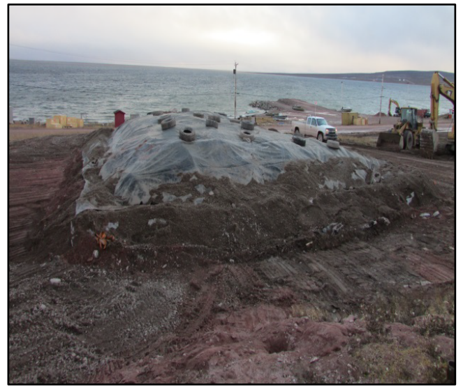
Photo 4 – Cell tarped with fill and tire ballast
