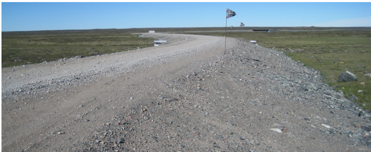
Figure 5-1b: The wide Meliadine Mine Road is 2+ m thick and built entirely from hauled and placed material, with no ditches.
