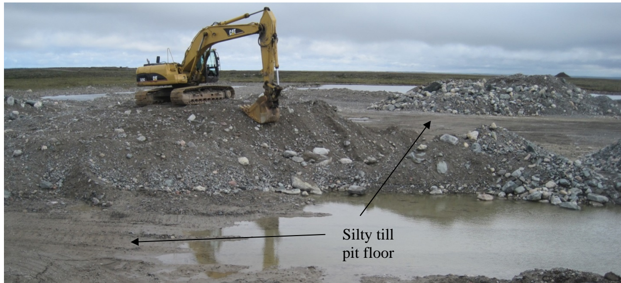
Figure 6-4: Excavated, unprocessed material in the Diane Pit. The silty till pit floor is visible, coinciding with the local groundwater table (Photo: July, 2016)
