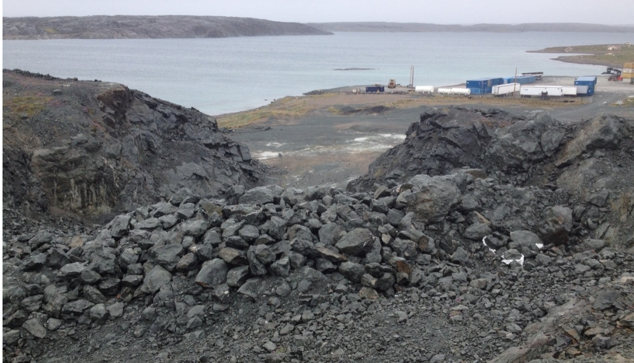
Figure 3-3: Existing bedrock quarry at the harbour south of the airport. It was initially used in 2007 to produce aggregates for the Hamlet. (Photo: July, 2016).
