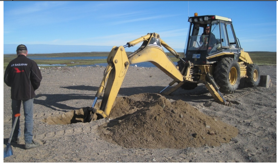
KM 19.0 on Diane River Road - Test Pit J5-S4 : Sand (fine to medium grain) with some gravel and trace cobbles. Permafrost at 6'3". No silty till.
