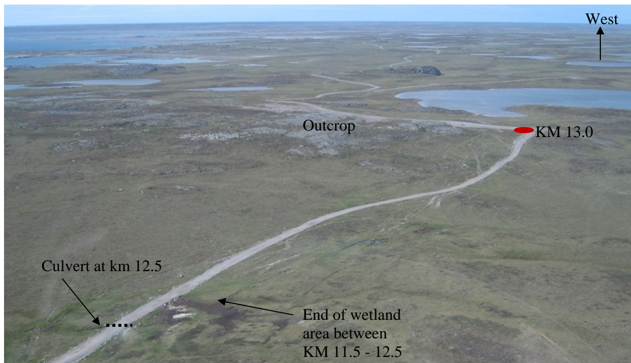
Figure 10-2: The present 3-4 m wide Diane River Road, looking west near KM 13.0. The sharp turns around the prominent outcrop slow traffic speeds (Photo: July, 2016).
