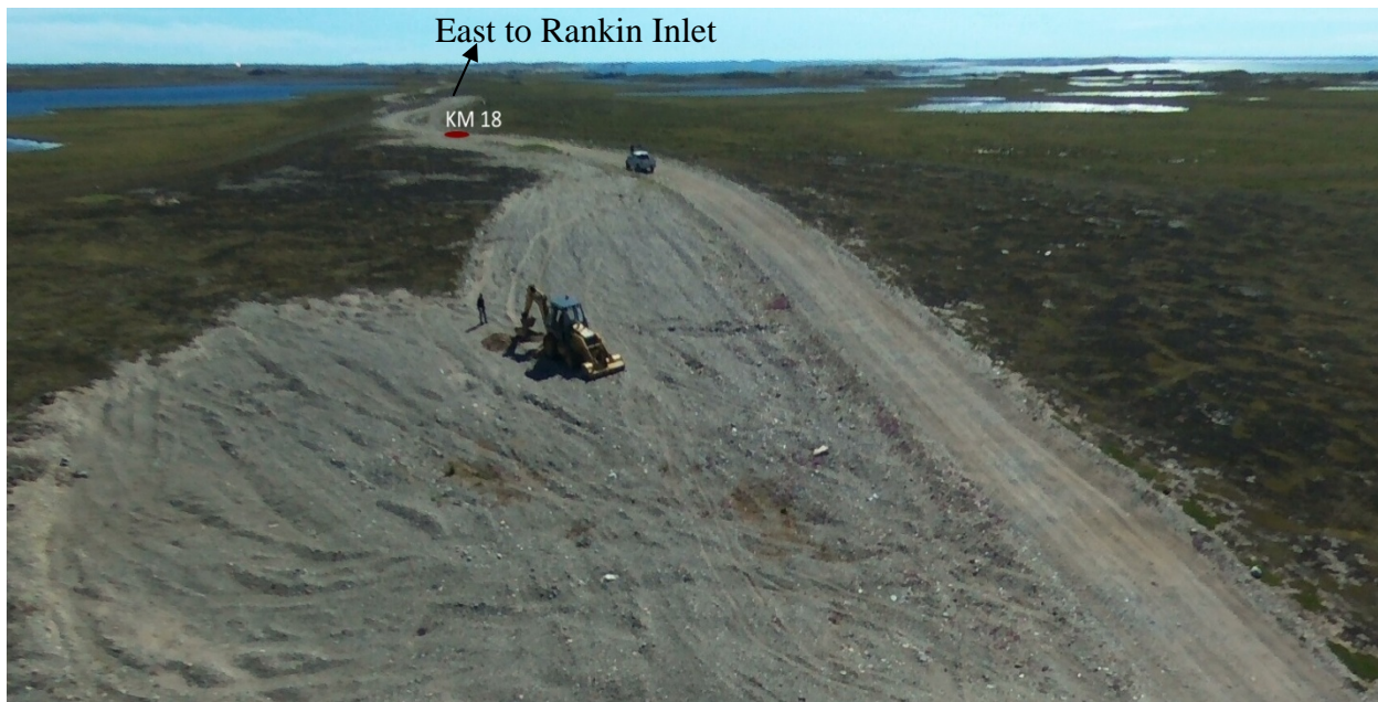
Figure 6-18: A test pit being excavated in the stripped area at the west end of the deposit at KM 18.0. The long narrow ridge can be seen extending eastward in the background, with the steep slope down to the north (left). (Photo: July, 2016).
