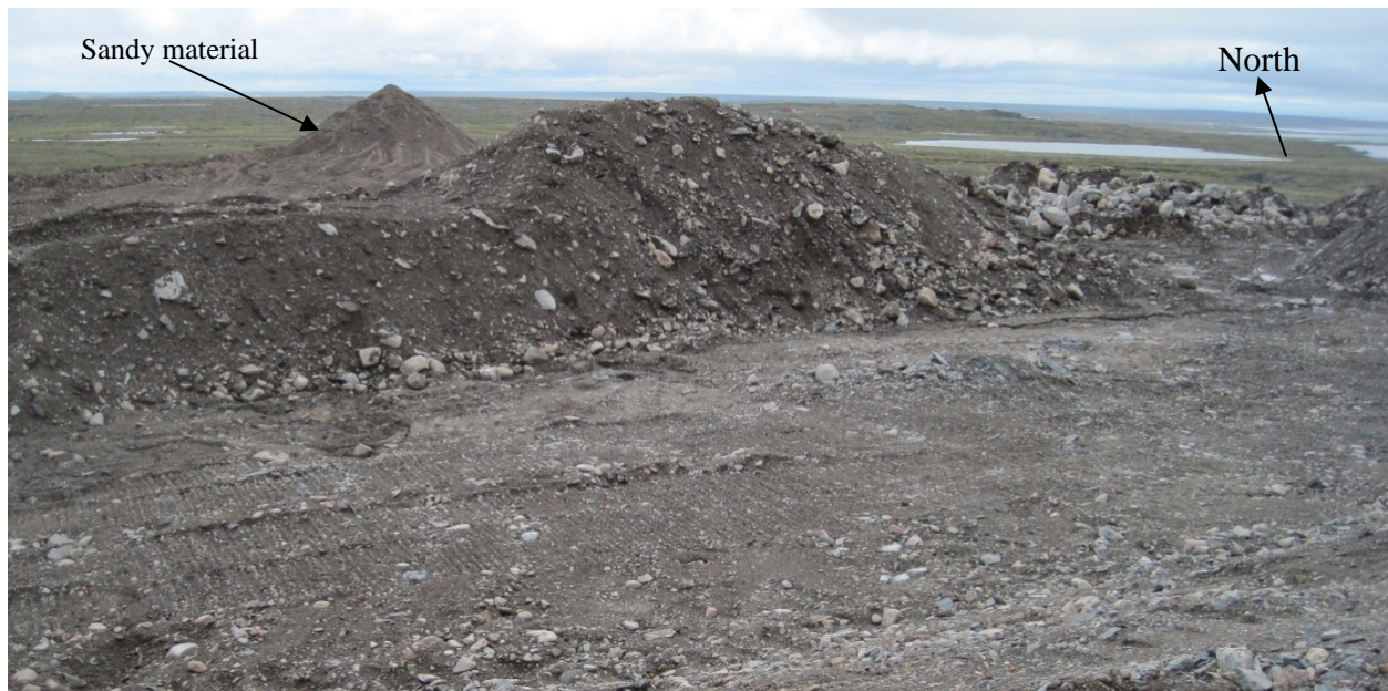
Figure 6-5: Recently excavated material from WSP Site 'A', which reportedly contains 86,000 m 3 of aggregate. View is north at KM 7.0 Diane River Road. (Photo: July, 2016).
