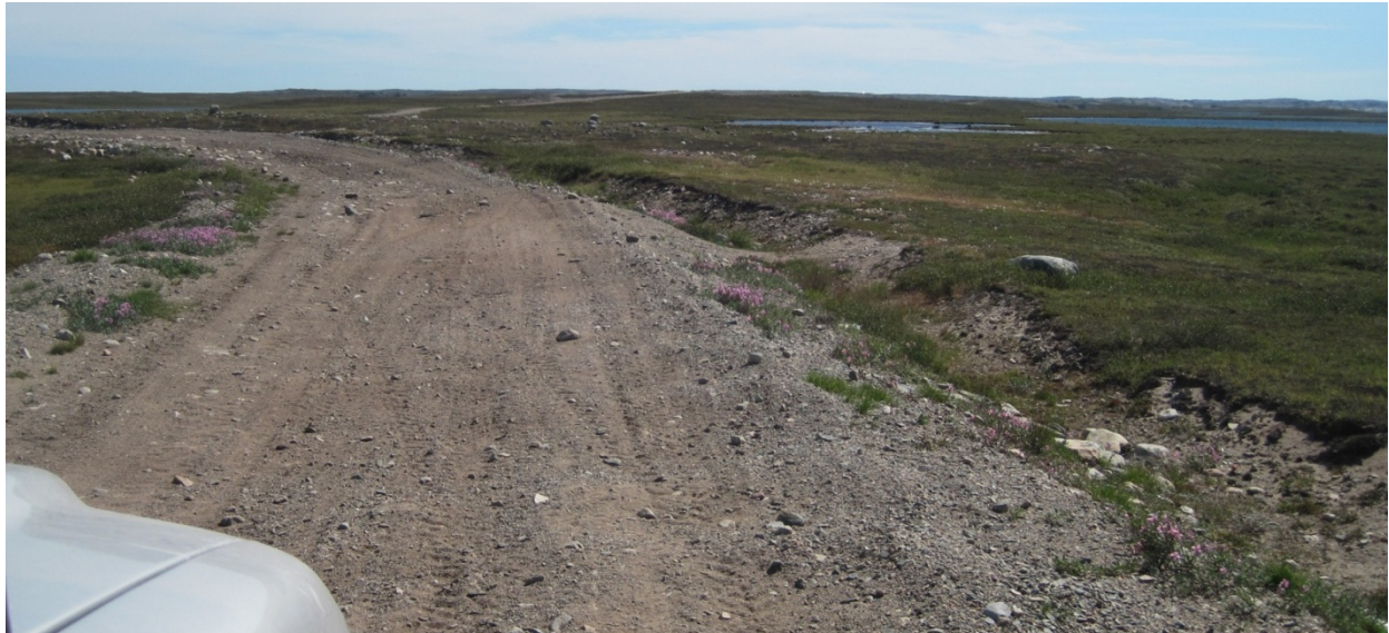
Figure 5-1a: The Diane River Rd. is an example of a narrow penetration road built with material from a drainage ditch with a thin sand and gravel running course where required.
