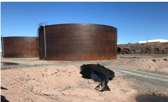
Photo 40: Exposed Liner at Fuel Tanks
