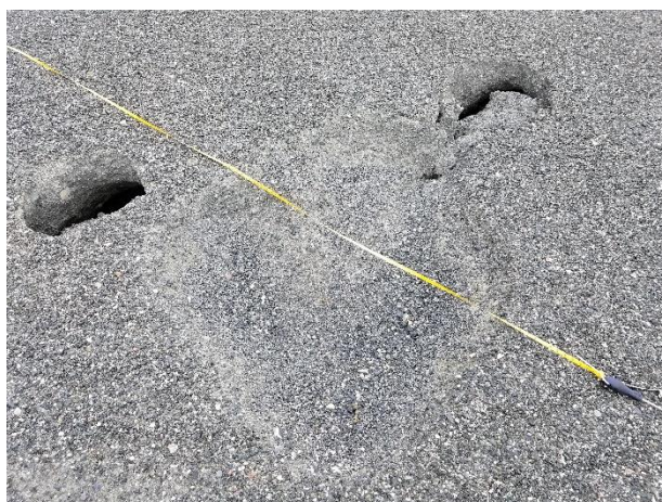
Photo 2: PKCA Sinkholes/Pothole
