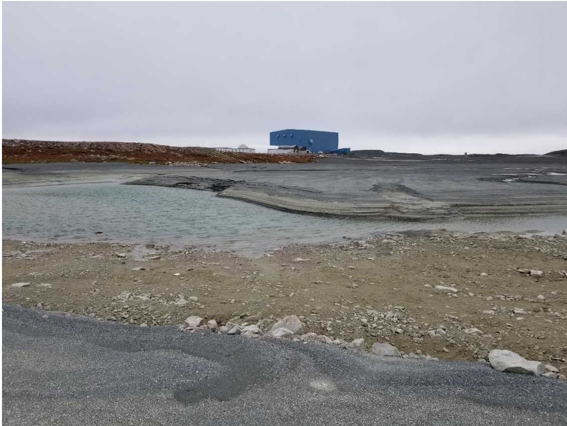
Photo 1: PKCA Water Ponding and Erosion
