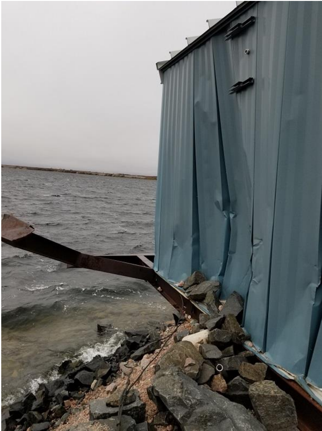
Figure 4: Ice Damage, Carat Lake Pumphouse
