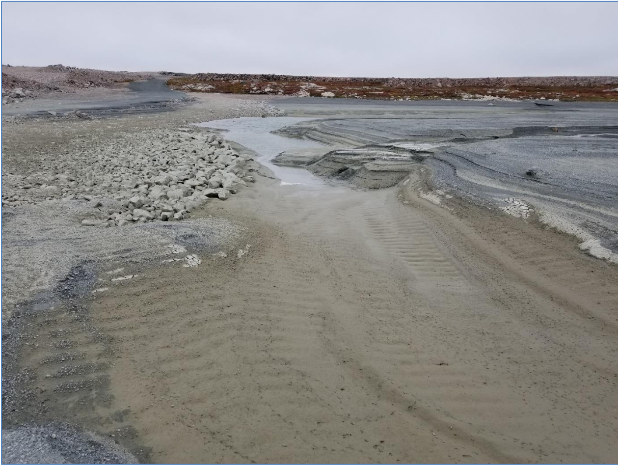
Photo 10: Sept. 1, 2020 PKCA Cover, Looking N – West end of North PKCA, wet exposed tailings.
