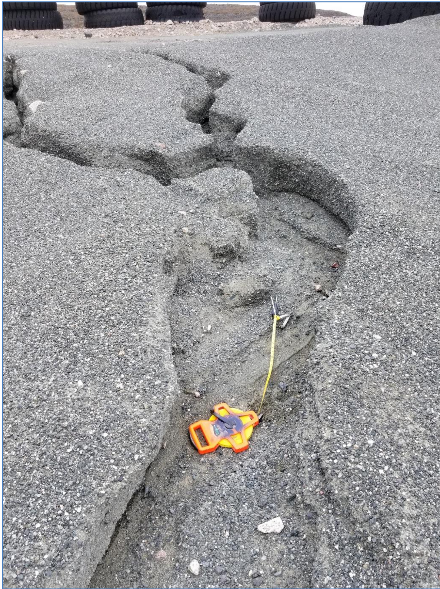
Photo 14: Sept. 1, 2020 PKCA Cover, East PKCA – Erosion from drainage into PKCA (some expansion from 2019).
