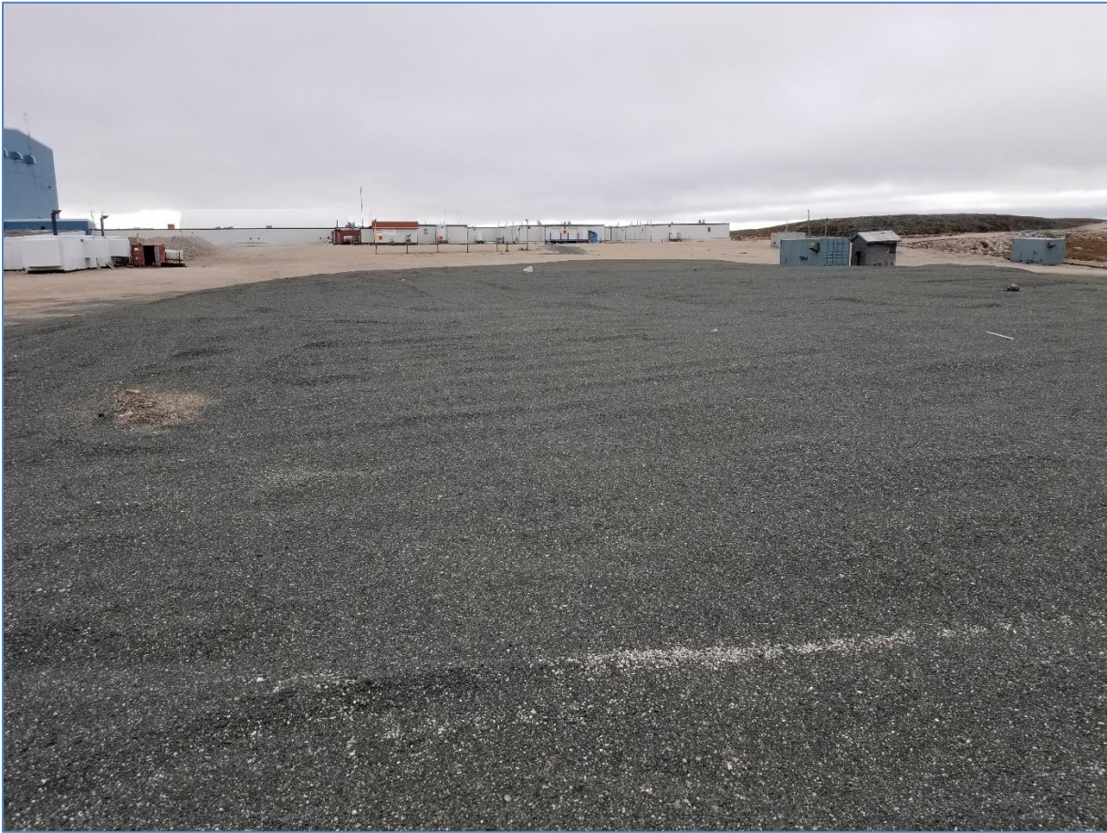
Photo 6: Sept. 1, 2020 PHC Containment Cell Cover, Looking SW (to camp) – Protection soil cover in good condition.
