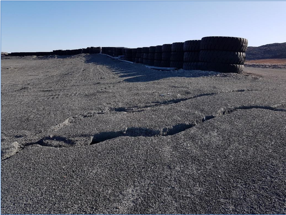
Photo 13: Sept. 11, 2019 PKCA Cover, East PKCA – 2019 photo of erosion from drainage into PKCA.
