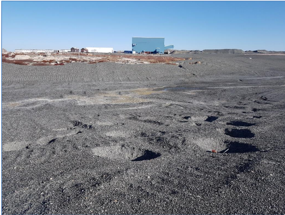
Photo 15: Sept. 11, 2019 PKCA Cover, Looking N – 2019 photo of potholes.
