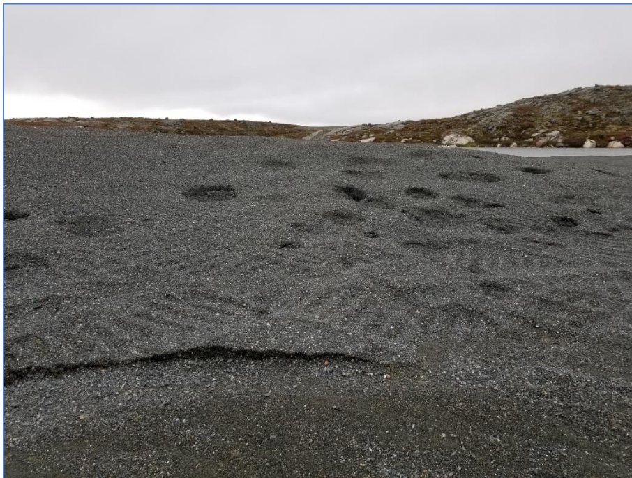
Photo 16: Sept. 1, 2020 PKCA Cover – Fall view of potholes (seasonally collapsed).
