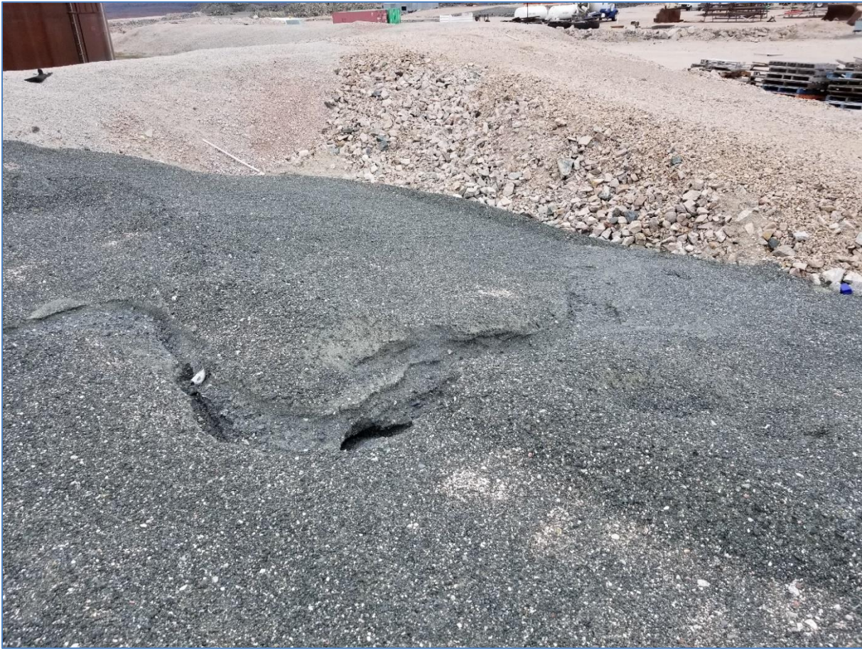
Photo 7: Sept 1, 2020 PHC Containment Cell Cover – Some minor drainage erosion in north corner of East Bank.
