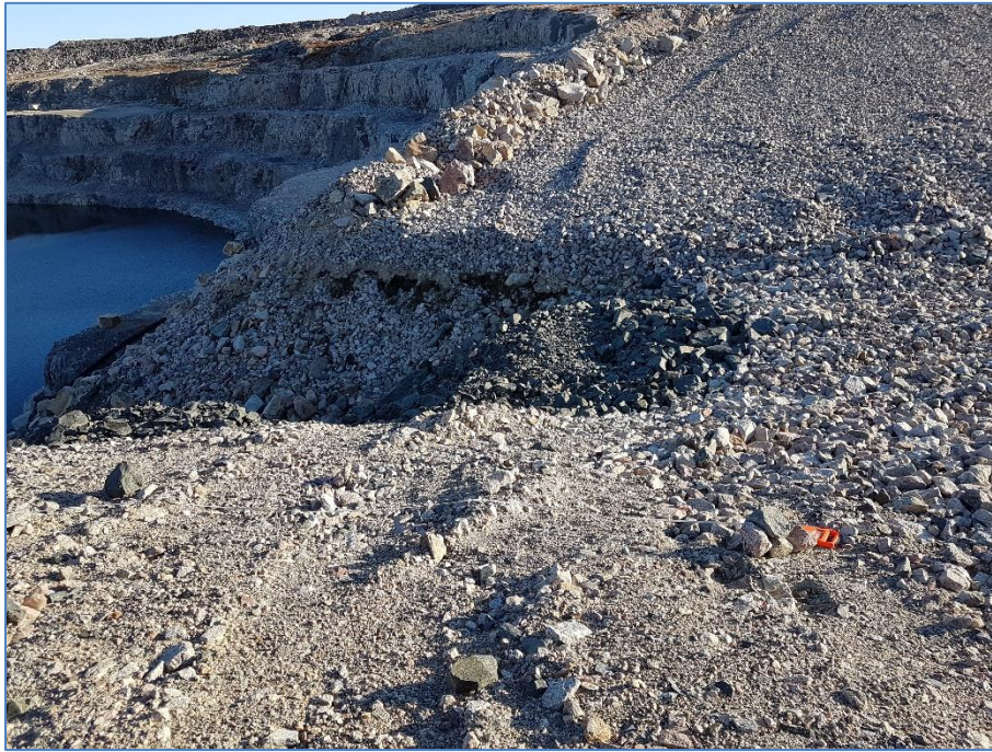
Photo 18: Sept. 10, 2019 C1 Channel, Looking E – 2019 photo of eroded section into Open Water @ 6.3 m in Fall.
