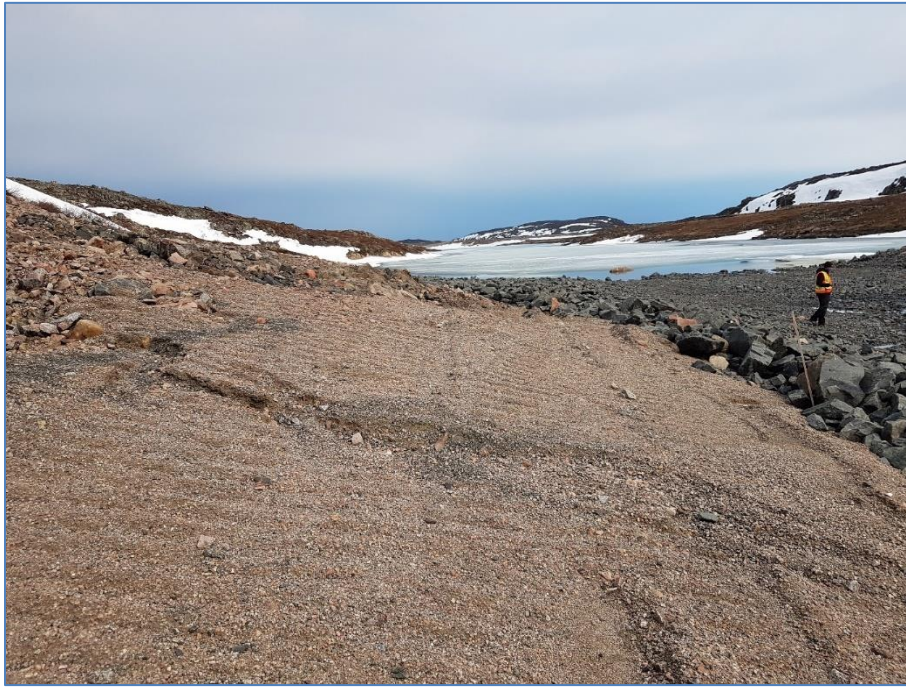
Photo 3: June 17, 2019 West Dam Breach – 2019 photo of erosion gully on North Bank.
