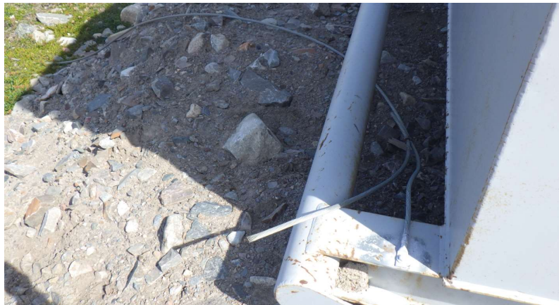
Figure 3-5 Surface Explosive Magazines – Grounding
