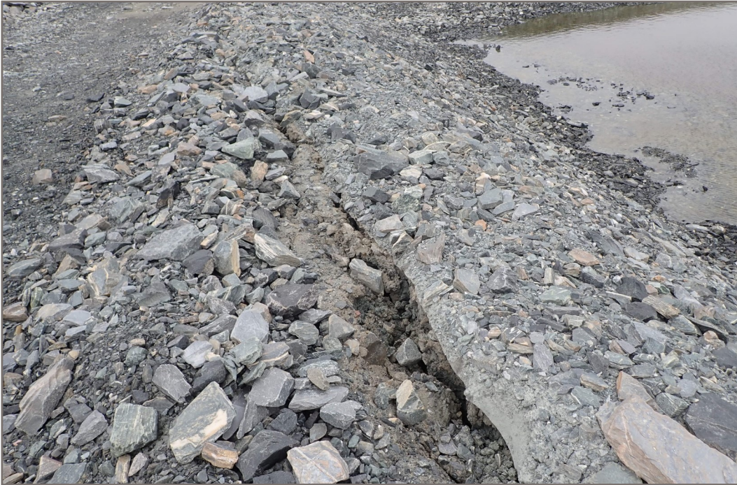
Photo 15: Dike D-CP1 - Subsidence and cracking at water collection pond downstream of the dike.
