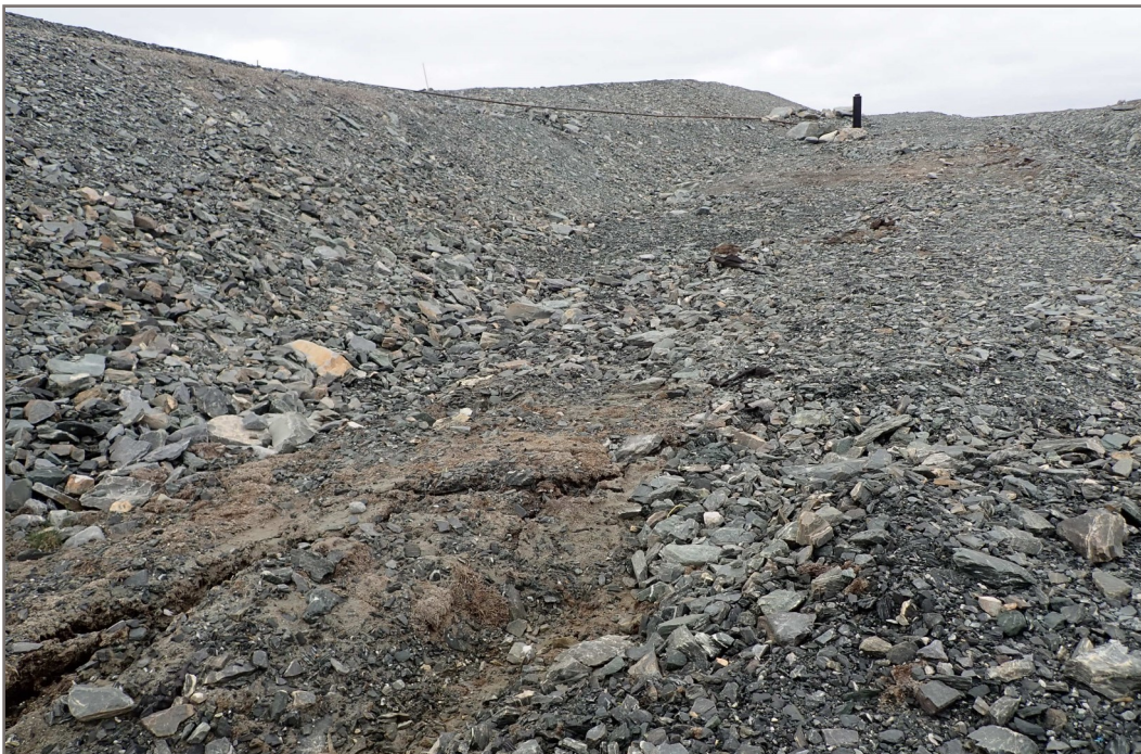
Photo 14: Dike D-CP1 - Subsidence and cracking between dike toe and water collection channel.
