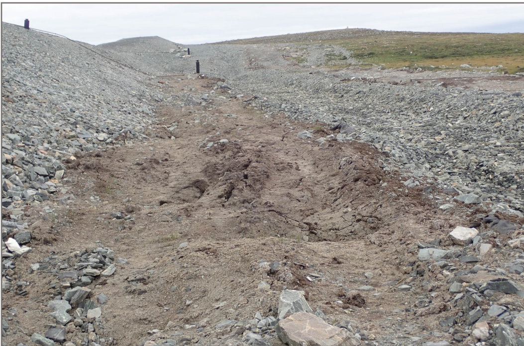
Photo 12: Dike D-CP1 - ground between the dike toe and water collection channel, settlement and subsidence
