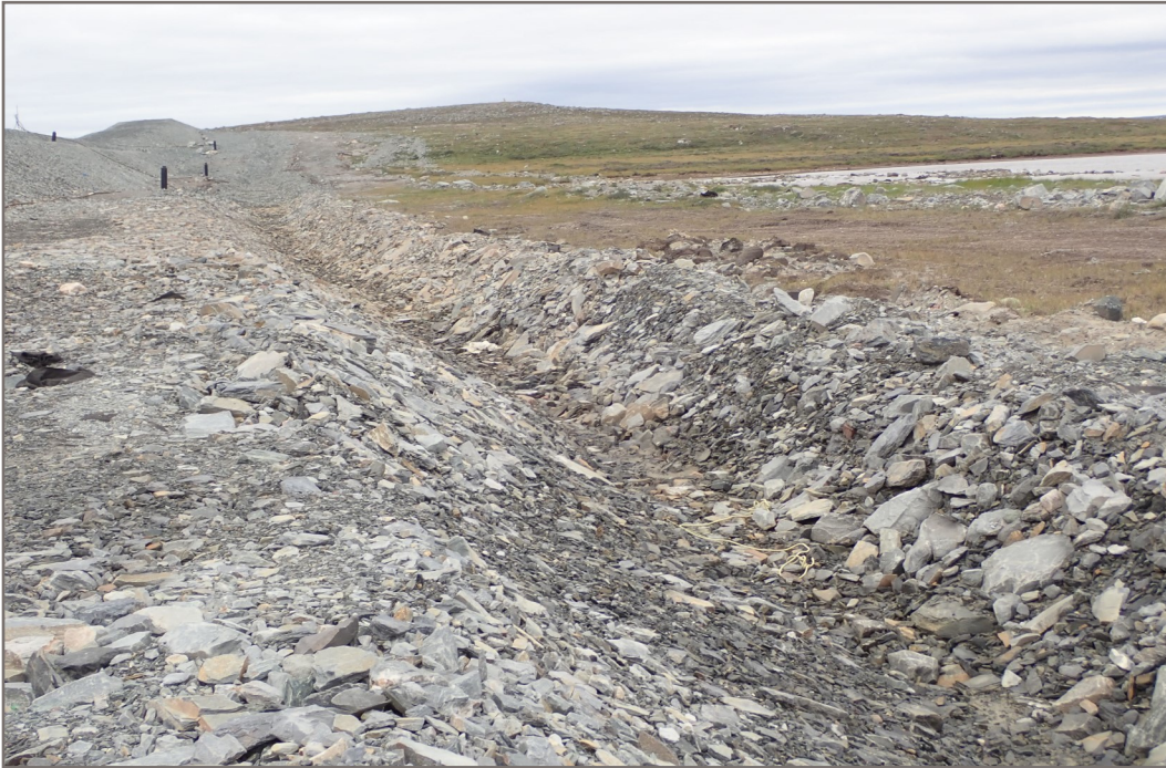
Photo 11: Dike D-CP1 - Water collection channel downstream of the Dike.
