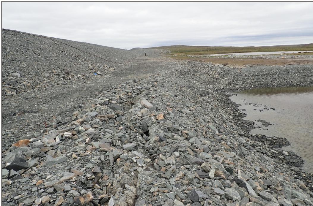
Photo 8: Dike D-CP1 - Downstream water collection pond, some cracking and subsidence at the upstream crest of the pond .
