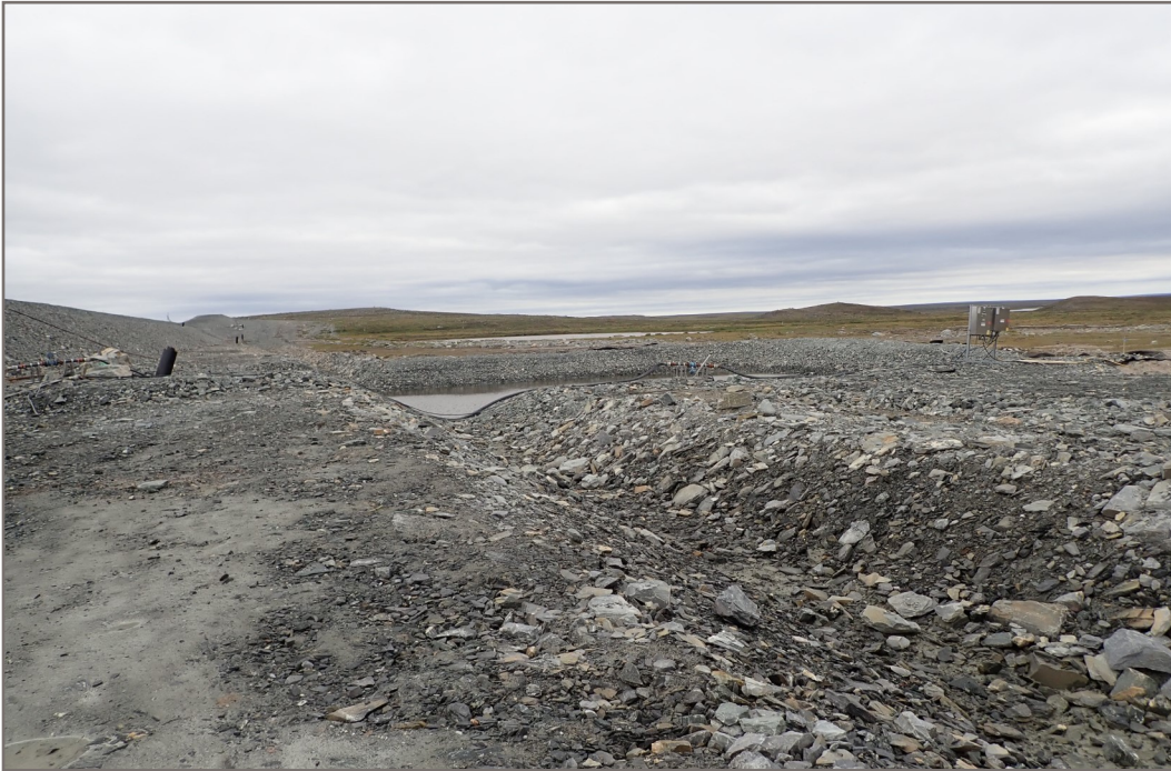
Photo 9: Dike D-CP1 - water collection channel at downstream toe of Dike (south end.)
