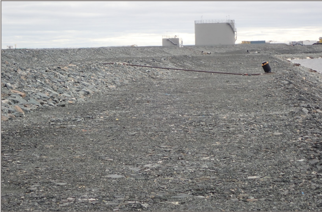
Photo 5: Dike D-CP1 - Upstream crest—some settlement is evident
