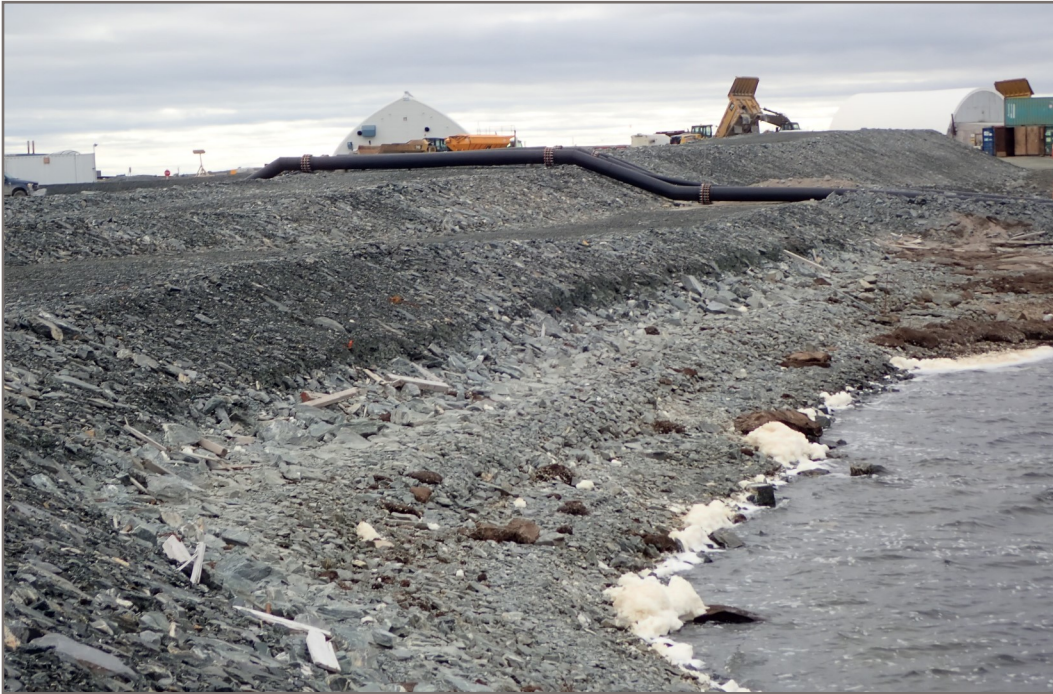
Photo 1: Dike D-CP1 - Upstream face—some wave and ice erosion evident
