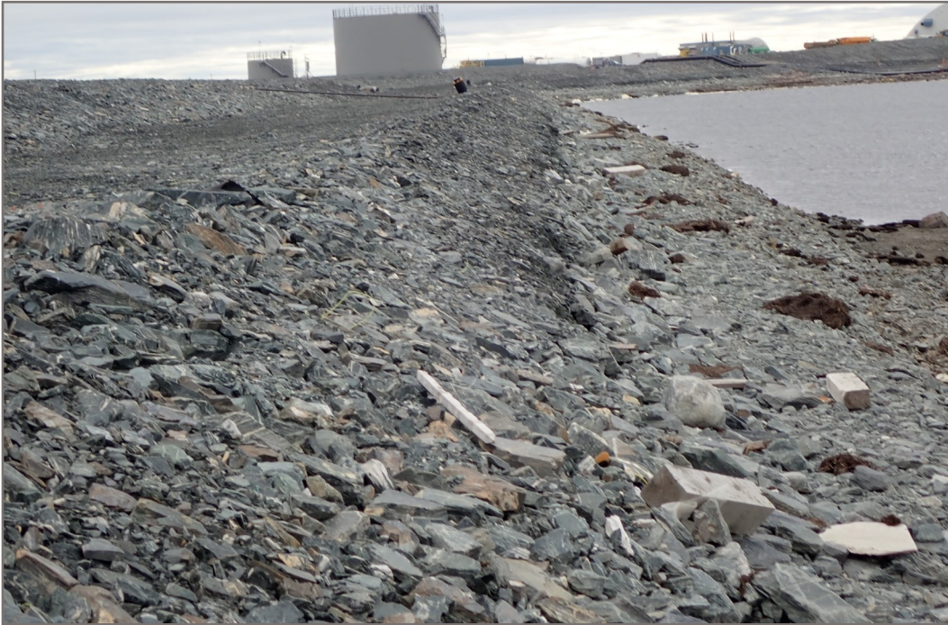
Photo 3: Dike D-CP1 - Upstream face—some wave erosion evident, scarp approximately 1 m high.
