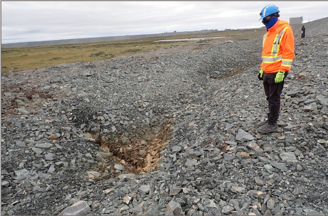
Photo 13: Dike D-CP1 - Subsidence in water collection channel, possibly caused by thaw of ice wedge below channel.
