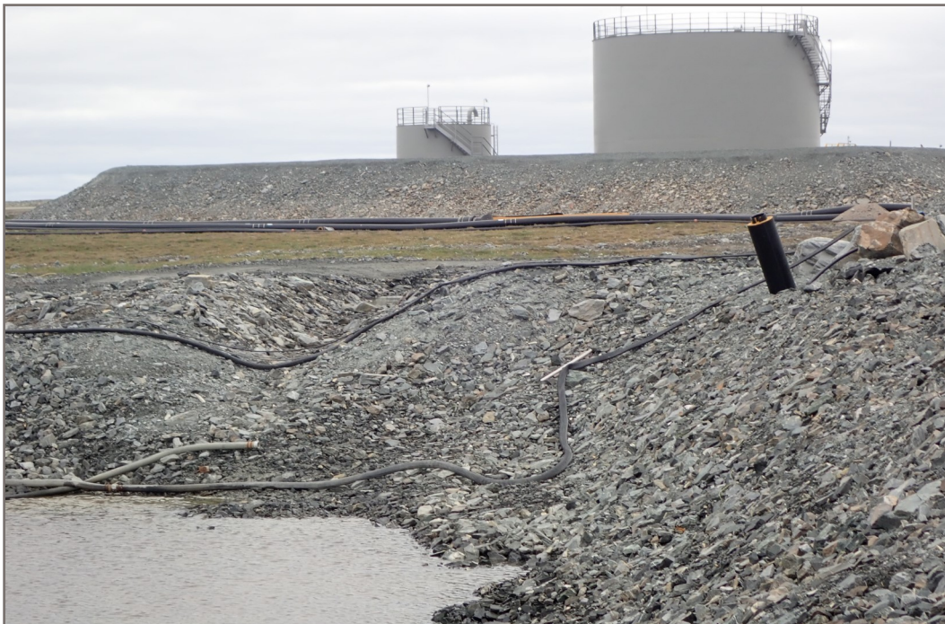
Photo 16: Dike D-CP1 - Subsidence at southeast corner of water collection pond downstream of the dike.
