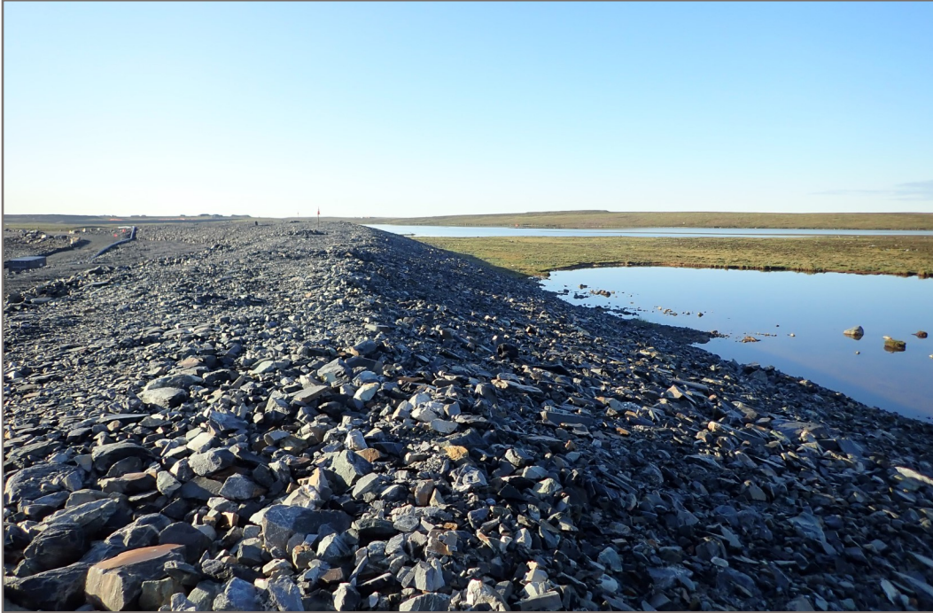
Photo 11: Berm CP3 - Downstream slope against lake B26.
