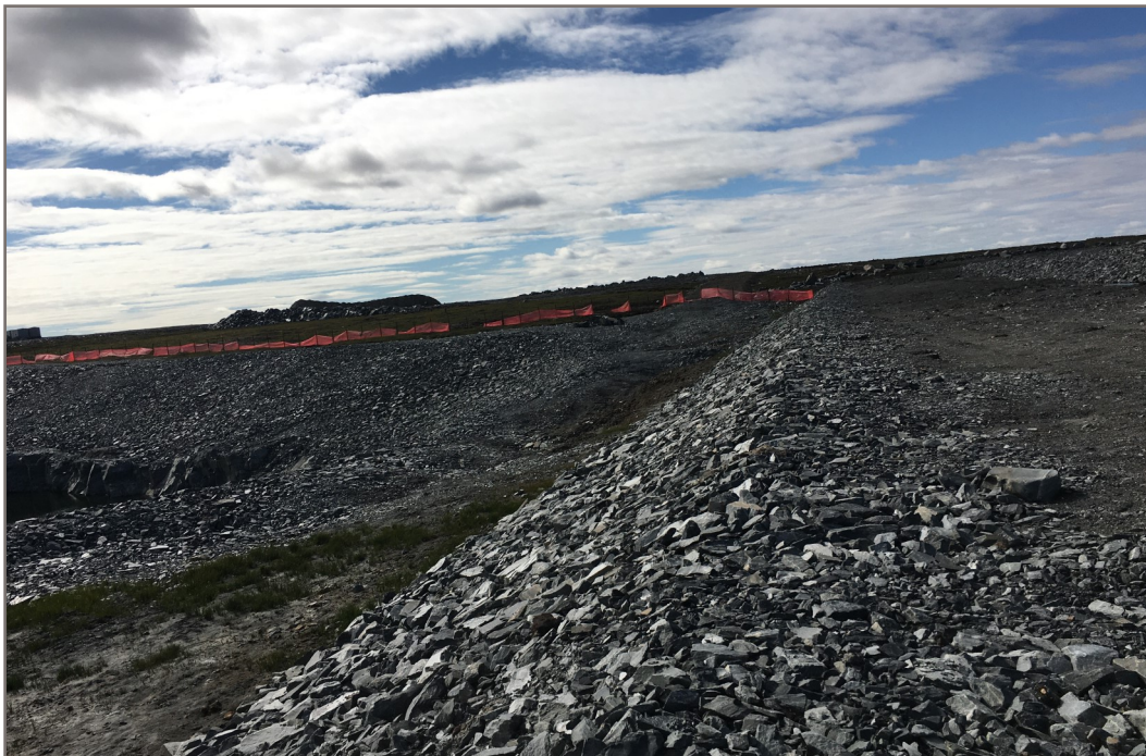
Photo 14: Berm CP4 - Upstream slope, thermal cover and original ground above Pond CP4
