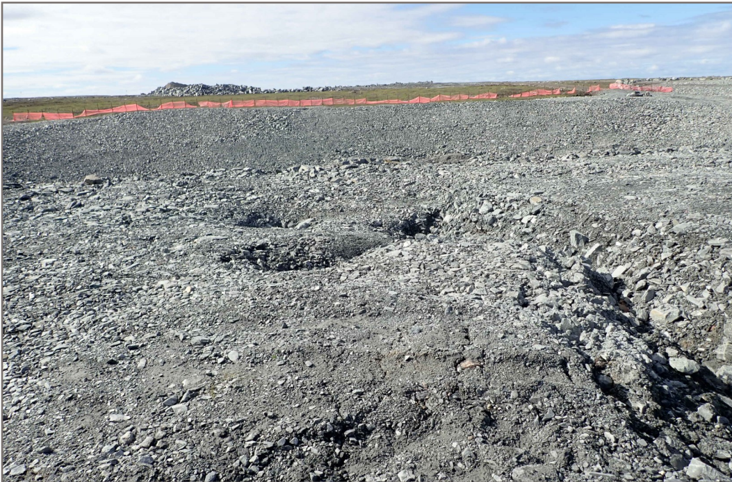
Photo 12: Pond CP4 - Settlement between original ground and north slope, looking south
