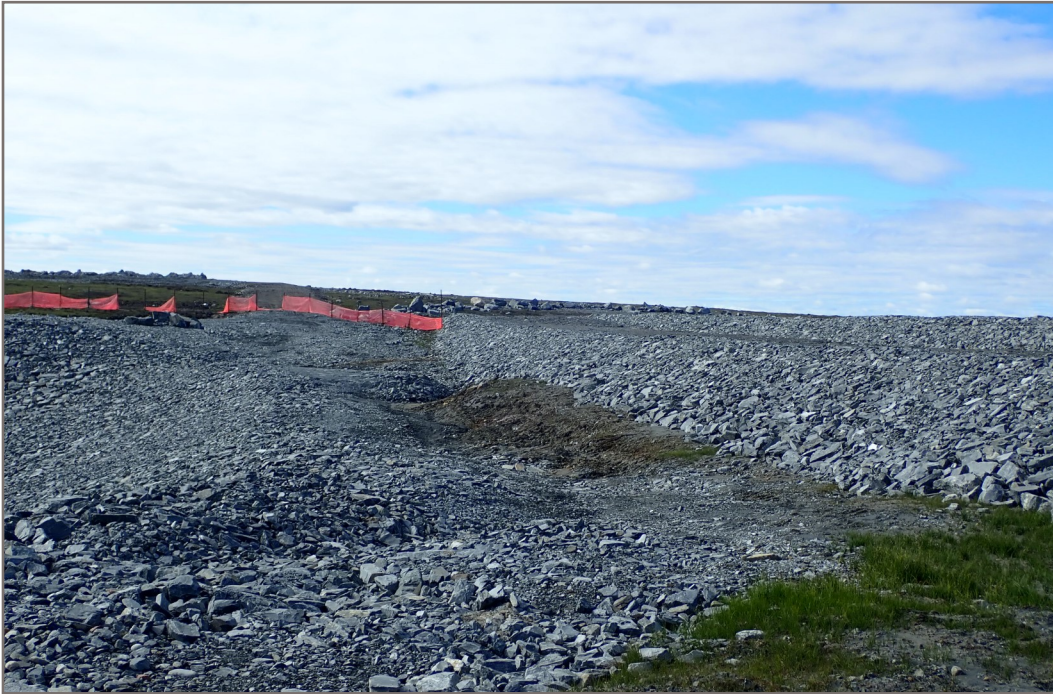
Photo 11: Pond CP4 - Settlement and between Berm CP4 and west pond slope.
