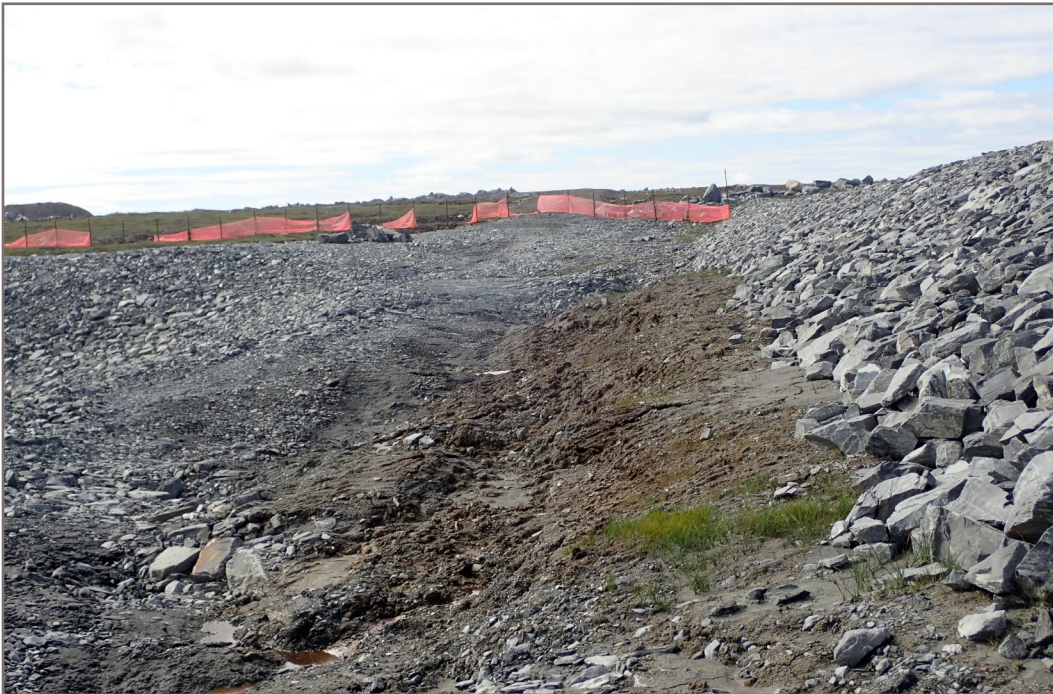
Photo 10: Pond CP4 - Settlement between Berm CP4 and west pond slope.
