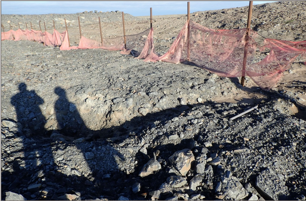
Photo 5: Pond CP3 - Runoff/erosion channel into pond from north end of TSF drainage, located on east side of pond.
