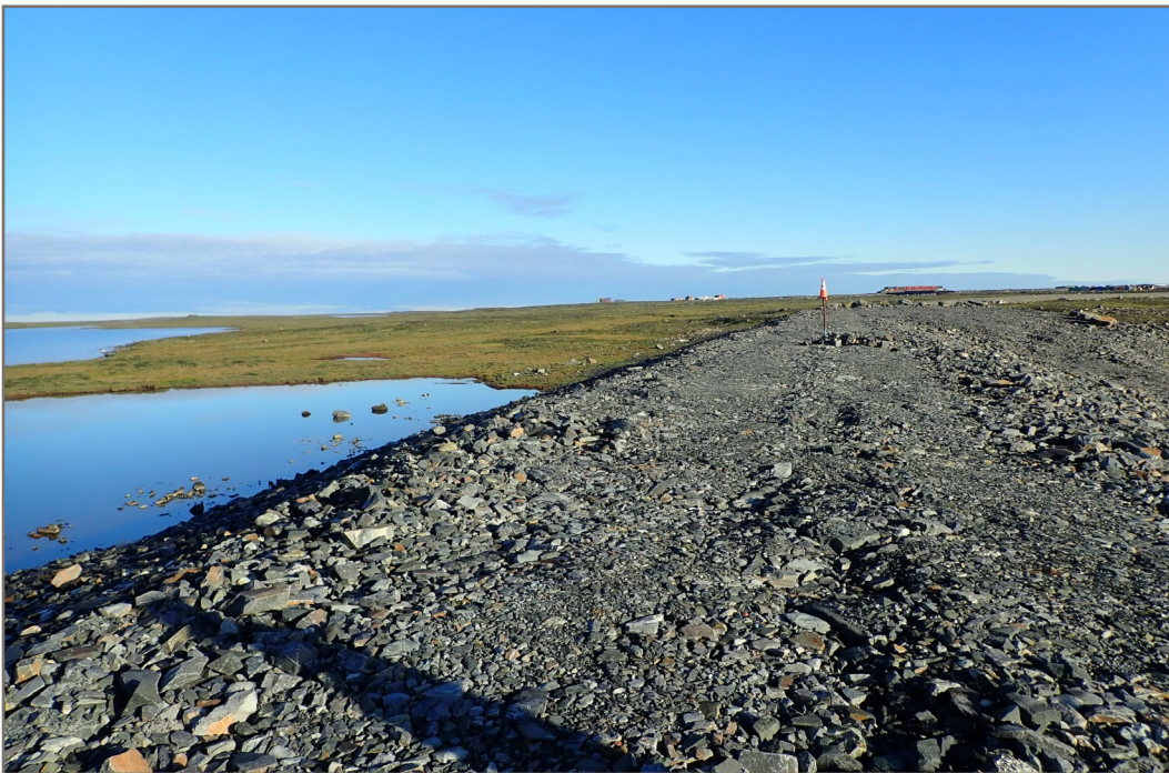
Photo 10: Berm CP3 - Berm crest, looking north. Undulations in crest 0.3 to 0.5 m.
