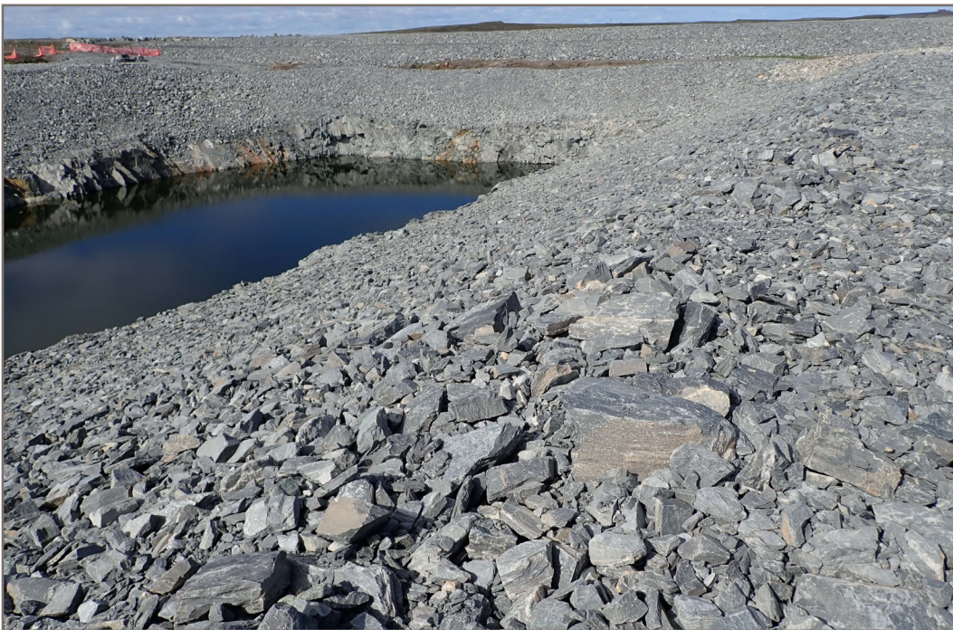
Photo 4: Pond CP4 - North slope—rockfill covered slope, no obvious signs of distress.
