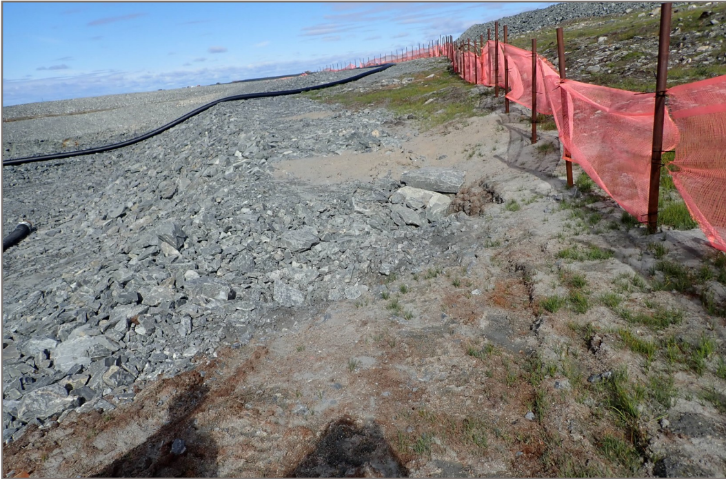
Photo 5: Pond CP4 - Settlement and cracking above north slope.
