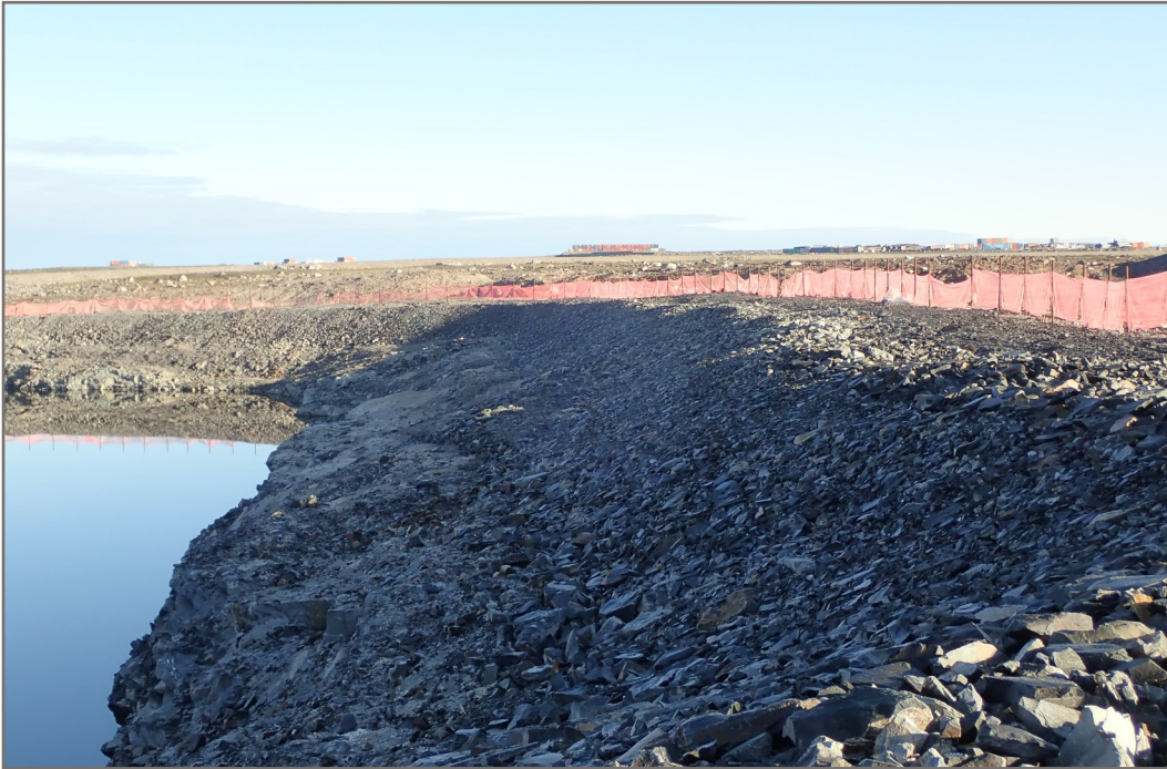
Photo 9: Pond CP3 - Rockfill covered overburden slope.
