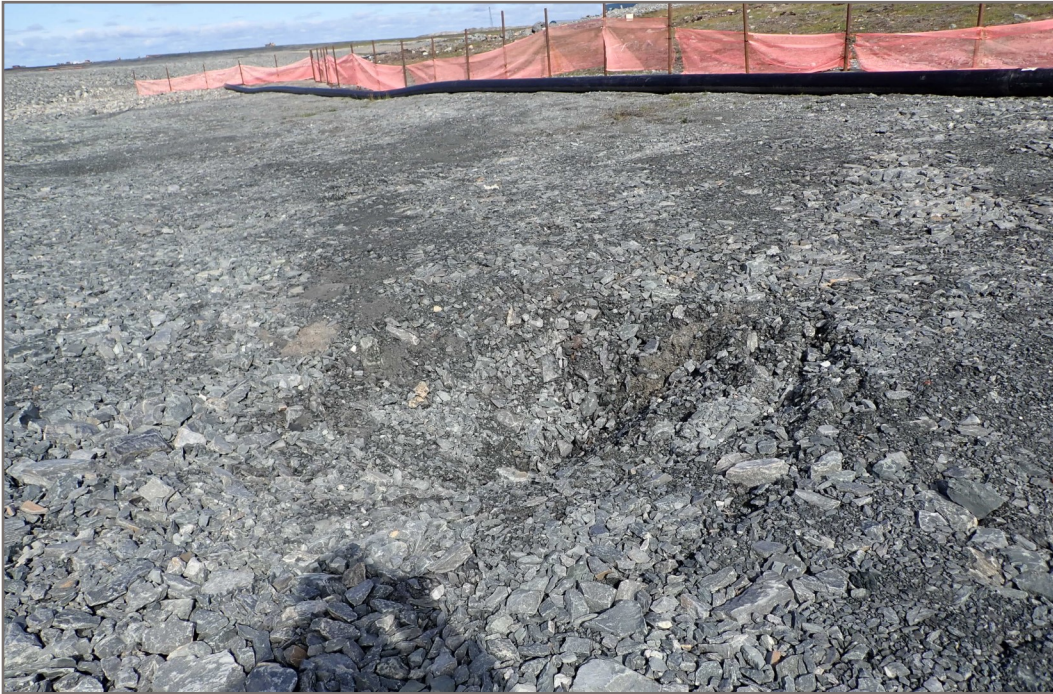
Photo 7: Pond CP4 - Ground above rockfill covered overburden slope. Settlement and subsidence in the area.
