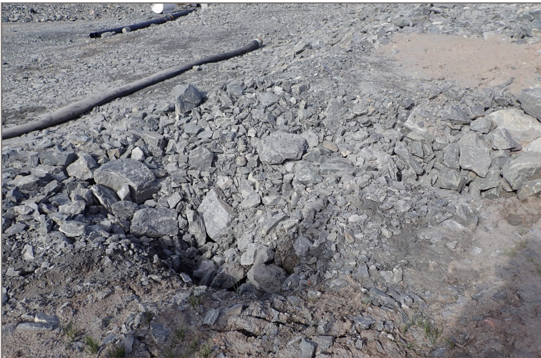
Photo 6: Pond CP4 - Small subsidence above north slope close to original ground contact.
