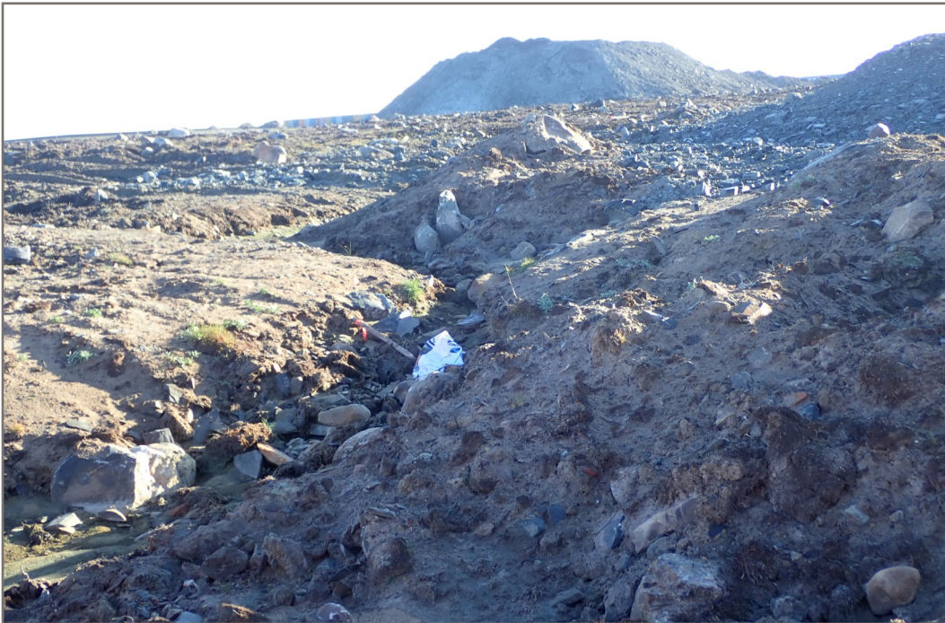
Photo 6: Pond CP3 - Runoff/erosion channel into pond from north end of TSF drainage, located on east side of pond.
