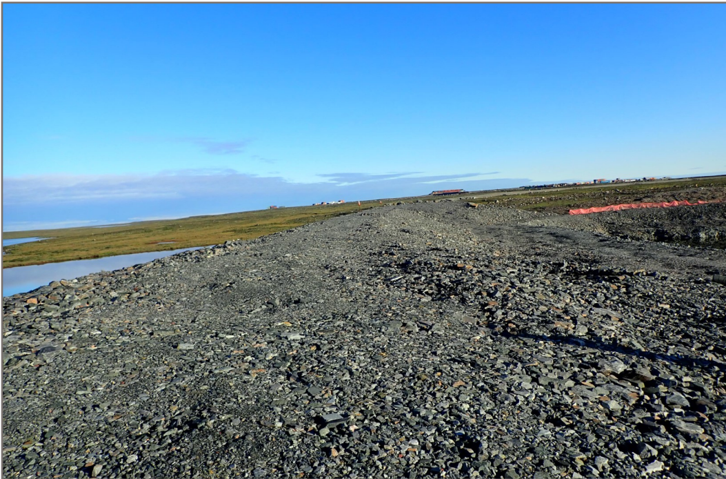
Photo 12: Berm CP3 - ground between the Dike toe and water collection channel, settlement and subsidence
