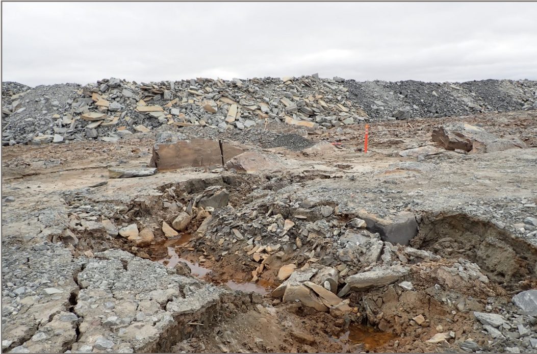
Photo 9: Pond CP6 - Former lakebed between Pond CP6 and WRSF3—erosion and subsidence channel.
