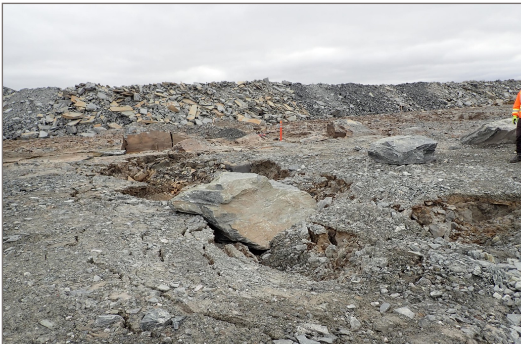
Photo 8: Pond CP6 - Former lakebed between Pond CP6 and WRSF3—erosion and subsidence channel.
