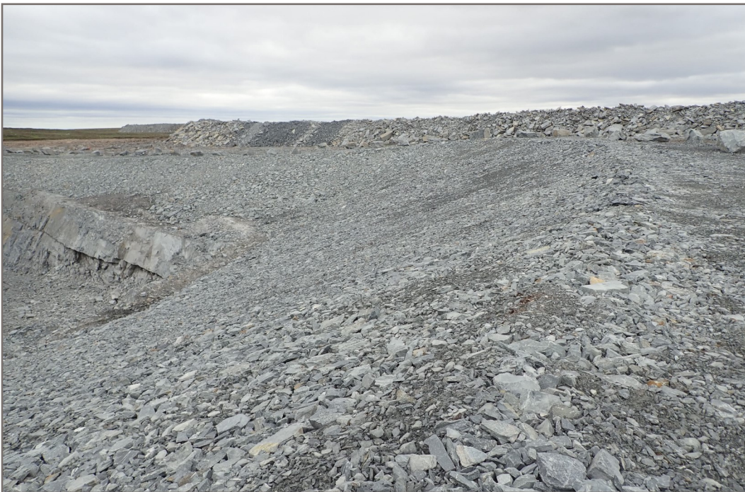
Photo 6: Pond CP6 - Southwest corner—Rockfill over the overburden slope.
