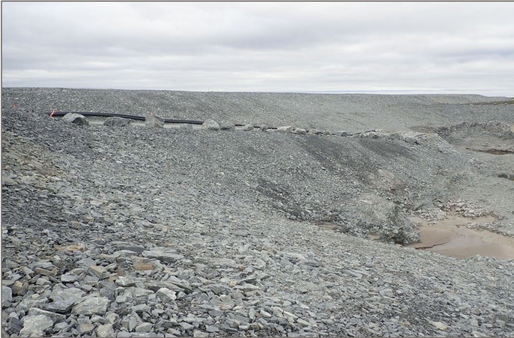
Photo 5: Pond CP6 - Upstream crest—some settlement is evident
