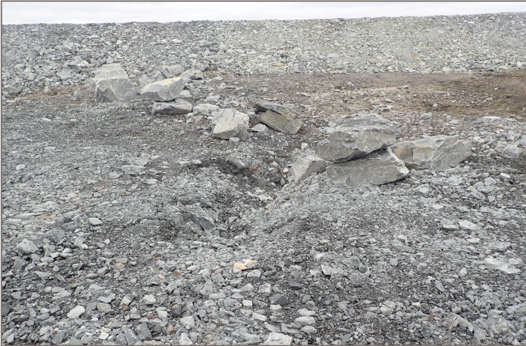
Photo 11: Pond CP6 - Subsidence and settlement in original ground adjacent to rockfill cover over overburden slope.
