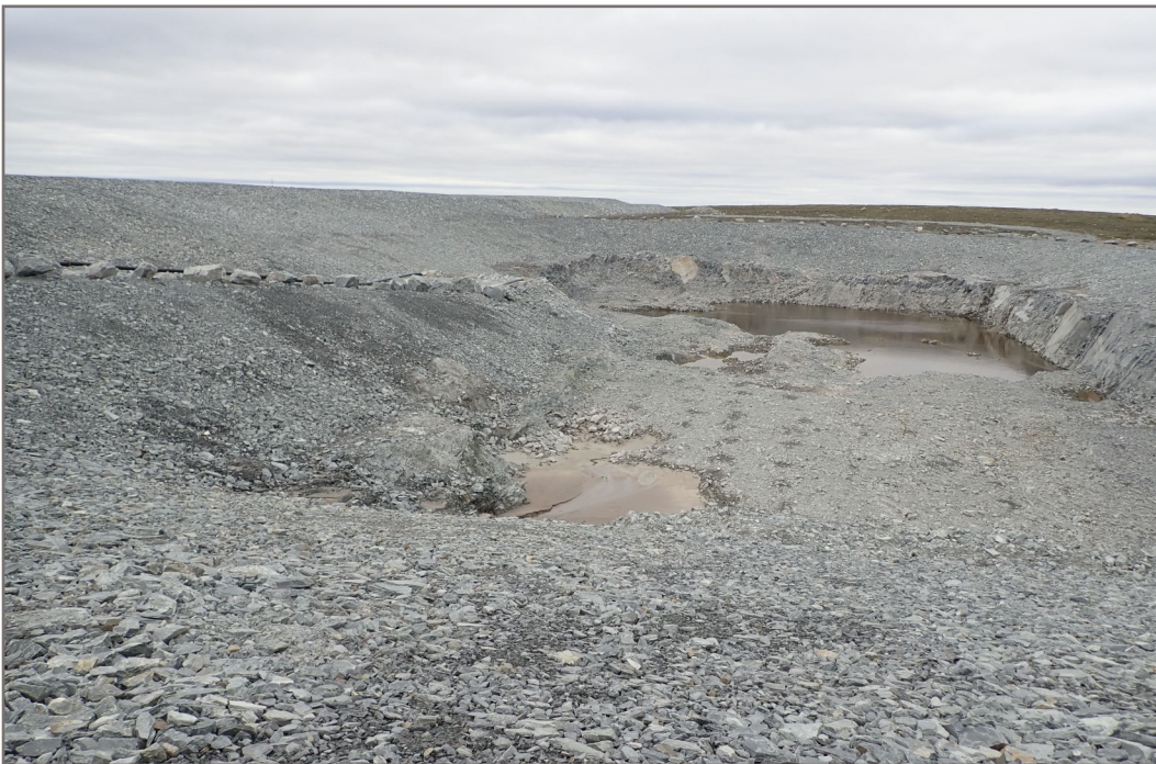
Photo 2: Pond CP6—Looking north, ramp into pond. Boulders along ramp. Some sediment washout in south west corner.
