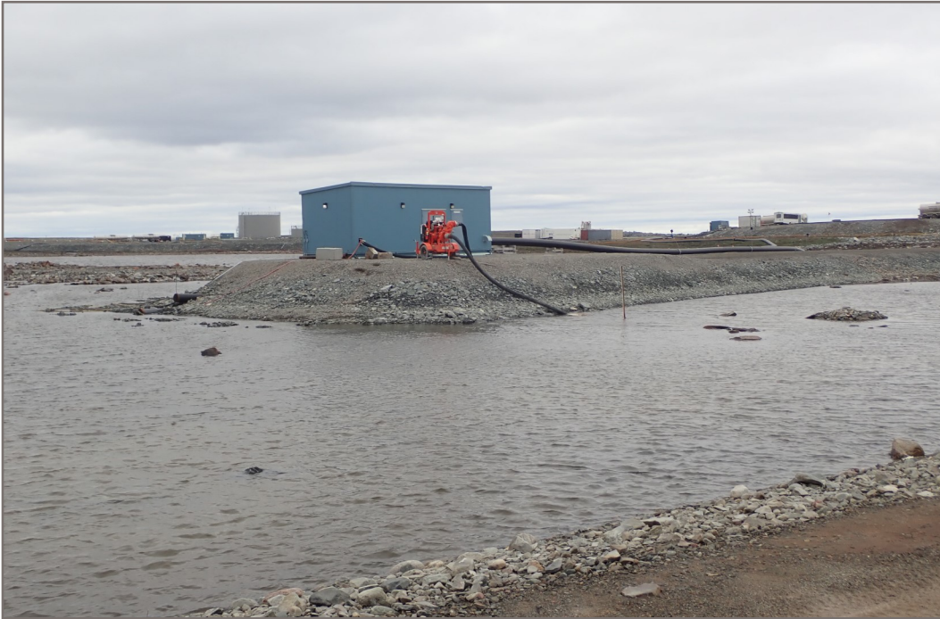
Photo 9: CP5 Jetty - looking towards the north east, erosion evident just above the water level.
