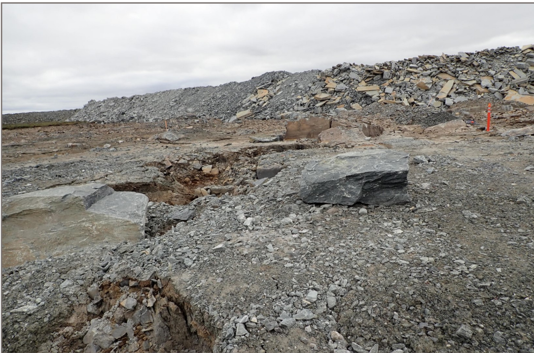
Photo 10: Pond CP6 - Former lakebed between Pond CP6 and WRSF3—erosion and subsidence channel.
