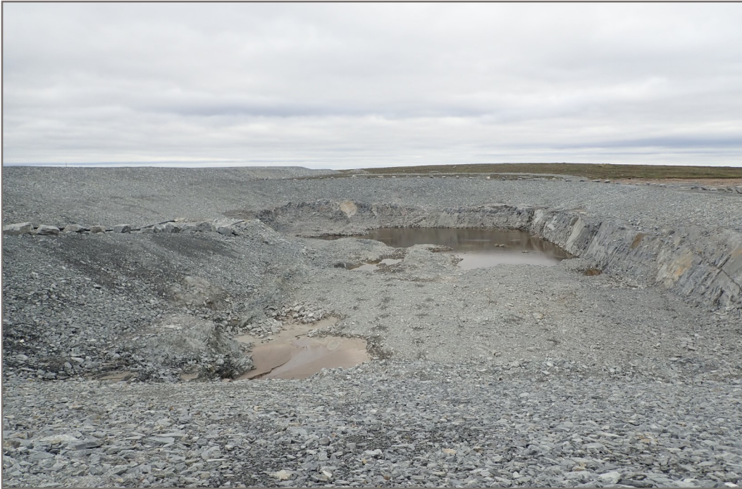
Photo 1: Pond CP6 - Looking north—contact between bedrock and overburden evident.
