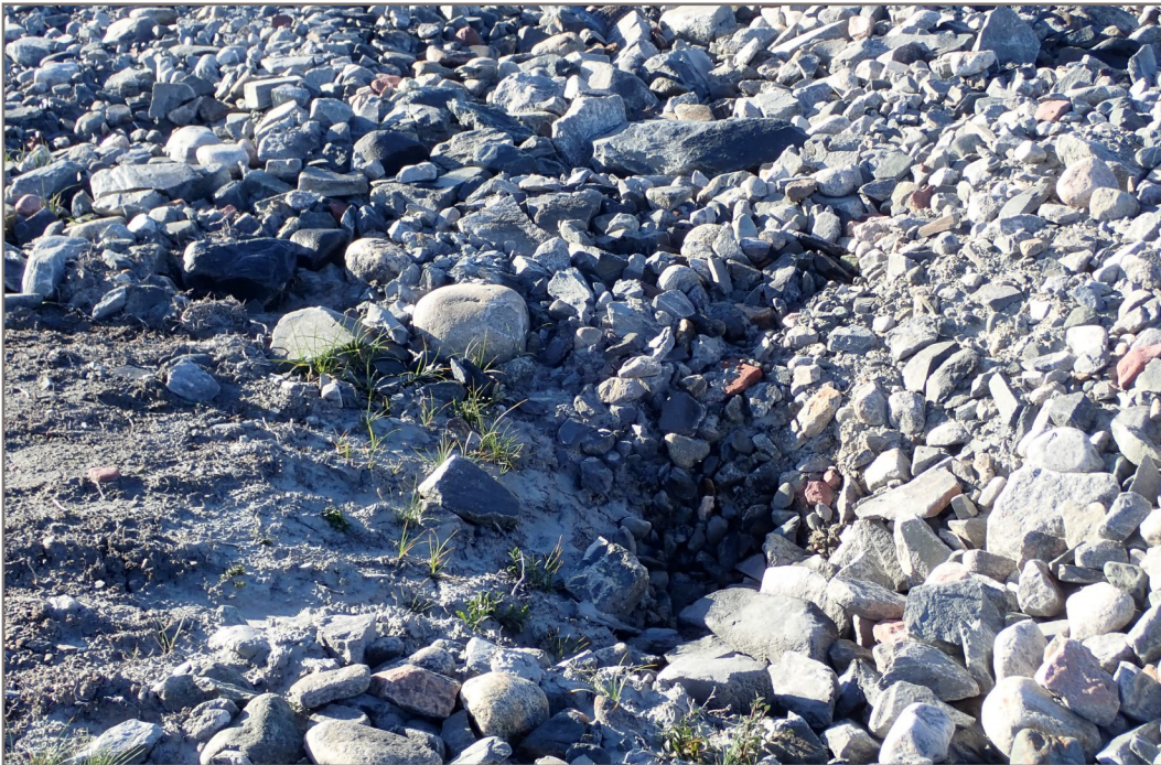
Photo 4: Channel 4 - Minor subsidence between original ground and channel rip rap.
