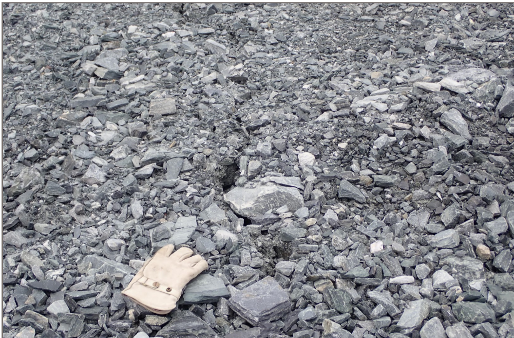
Photo 18: Berm CP6 - Cracking in rockfill berm cover.
