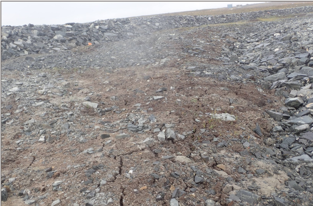
Photo 18: SP4 Saline Pond—Cracking in disturbed overburden above rockfill covered slope.
