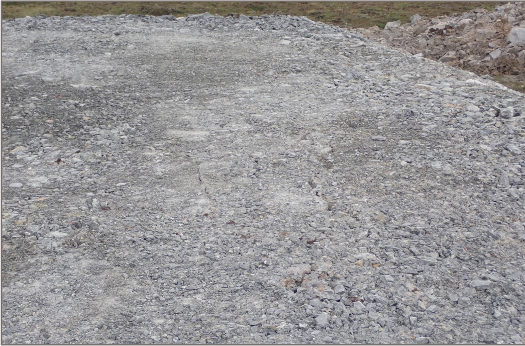
Photo 17: Berm CP6 - minor cracking in upstream/till cover.
