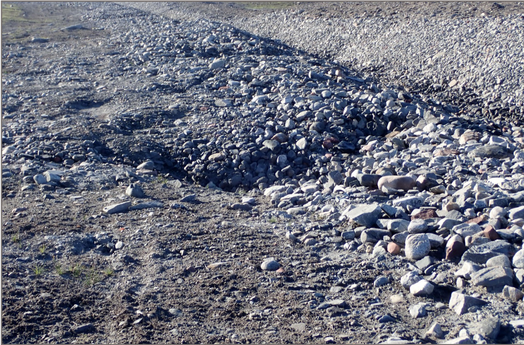
Photo 5: Channel 4 - Subsidence in rip rap—in upstream slope (east) slope of the channel.
