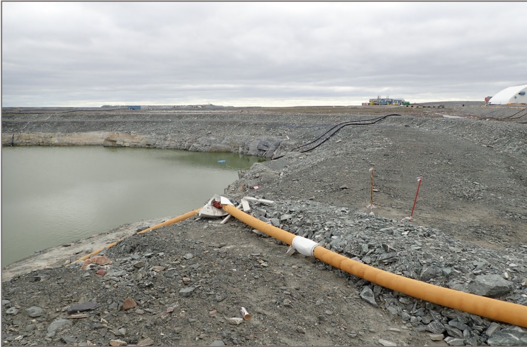
Photo 3: SP1 Saline Pond - discharge line into pond.
