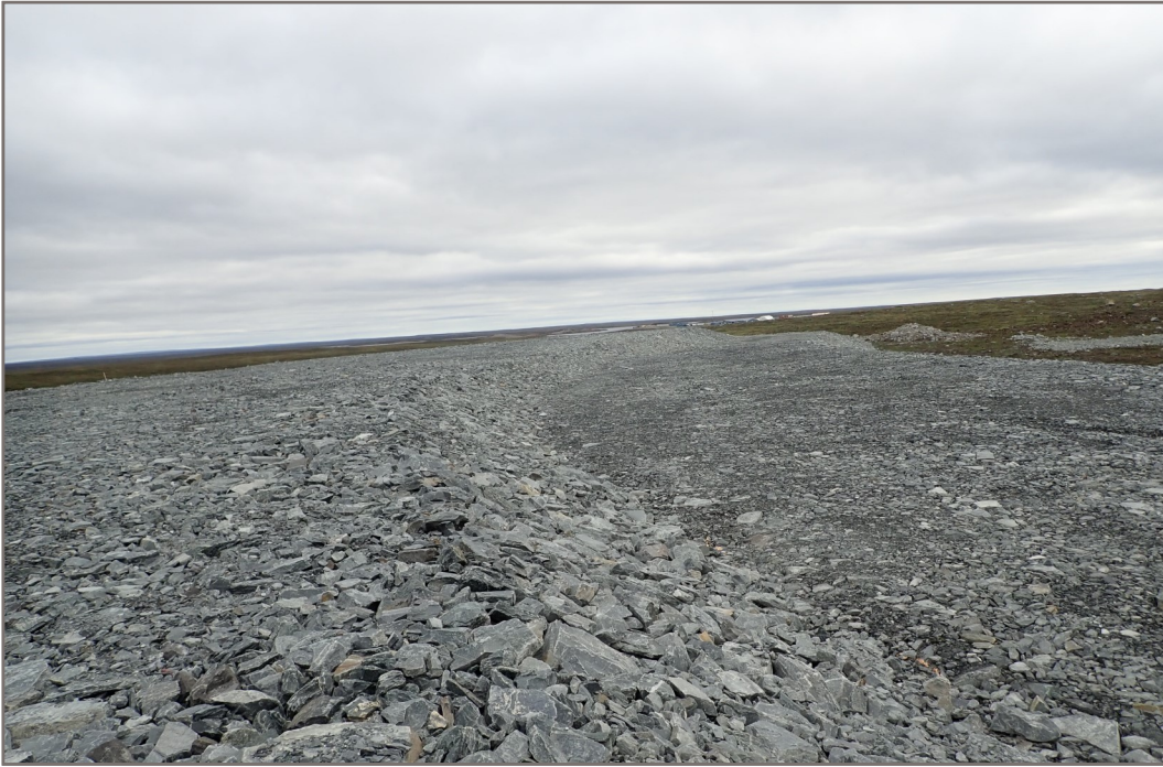
Photo 15: Berm CP6 - Crest and rockfill cover over upstream ground
