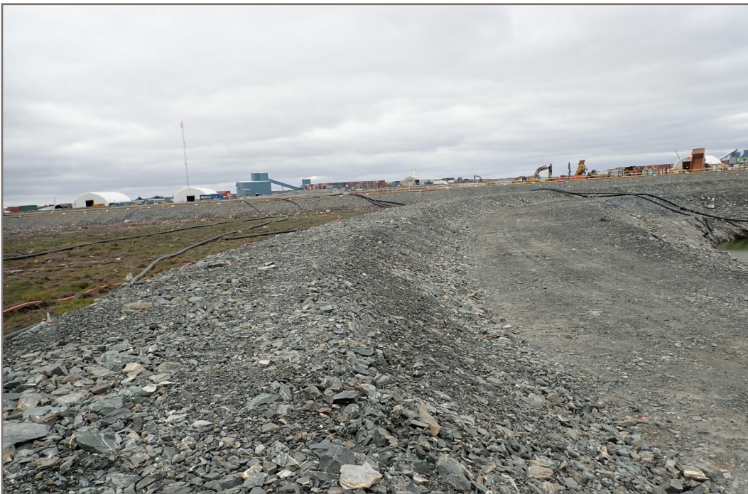
Photo 4: SP1 Saline Pond - thermal berm at crest.
