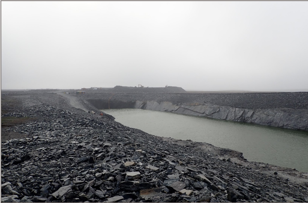
Photo 11: SP4 Saline Pond - looking east. Rockfill covered overburden slope over bedrock.
