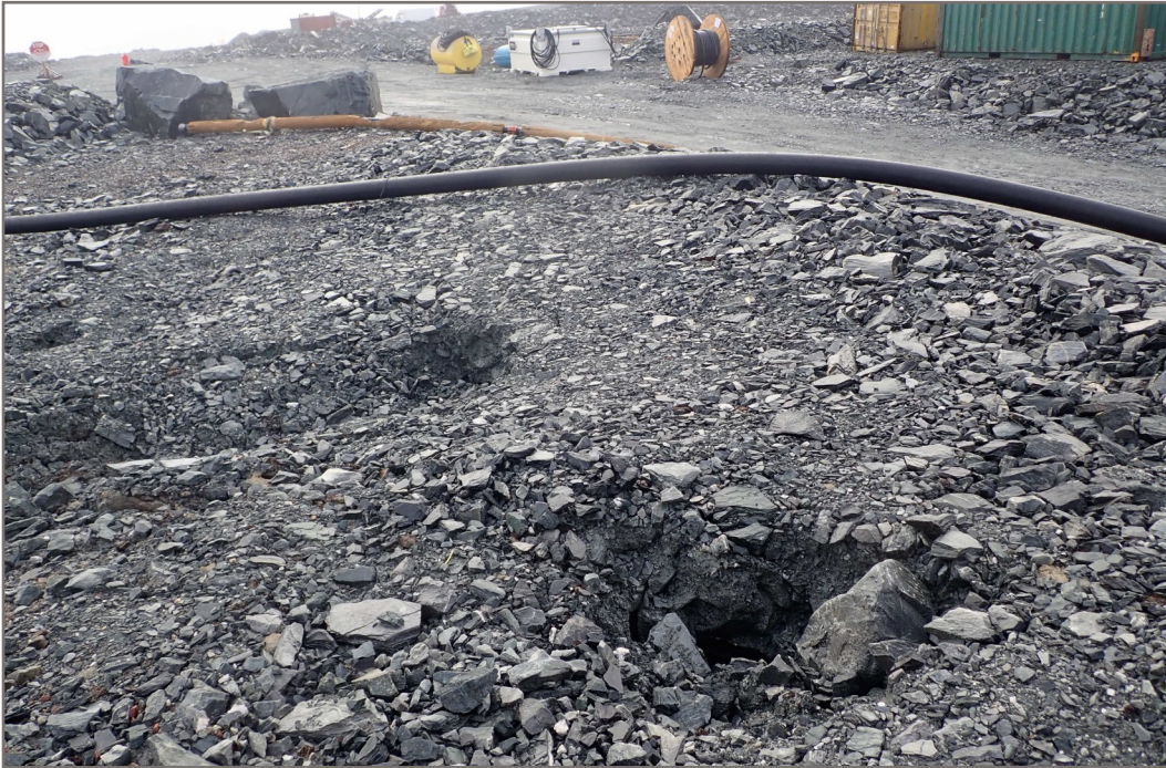
Photo 15: SP4 Saline Pond—Subsidence in rockfill at crest of slope.
