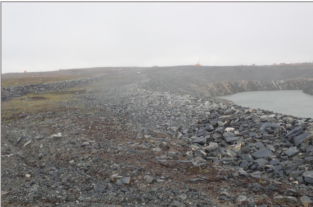
Photo 16: SP4 Saline Pond - Settlement of rockfill covering overburden slope.
