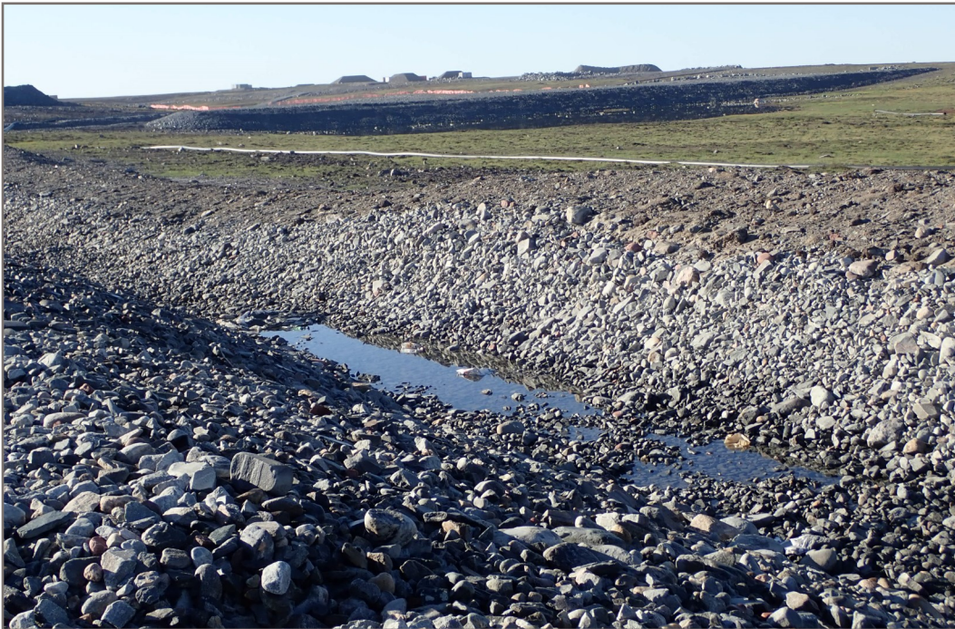
Photo 6: Channel 4 - Lower reach channel, minor ponding.
