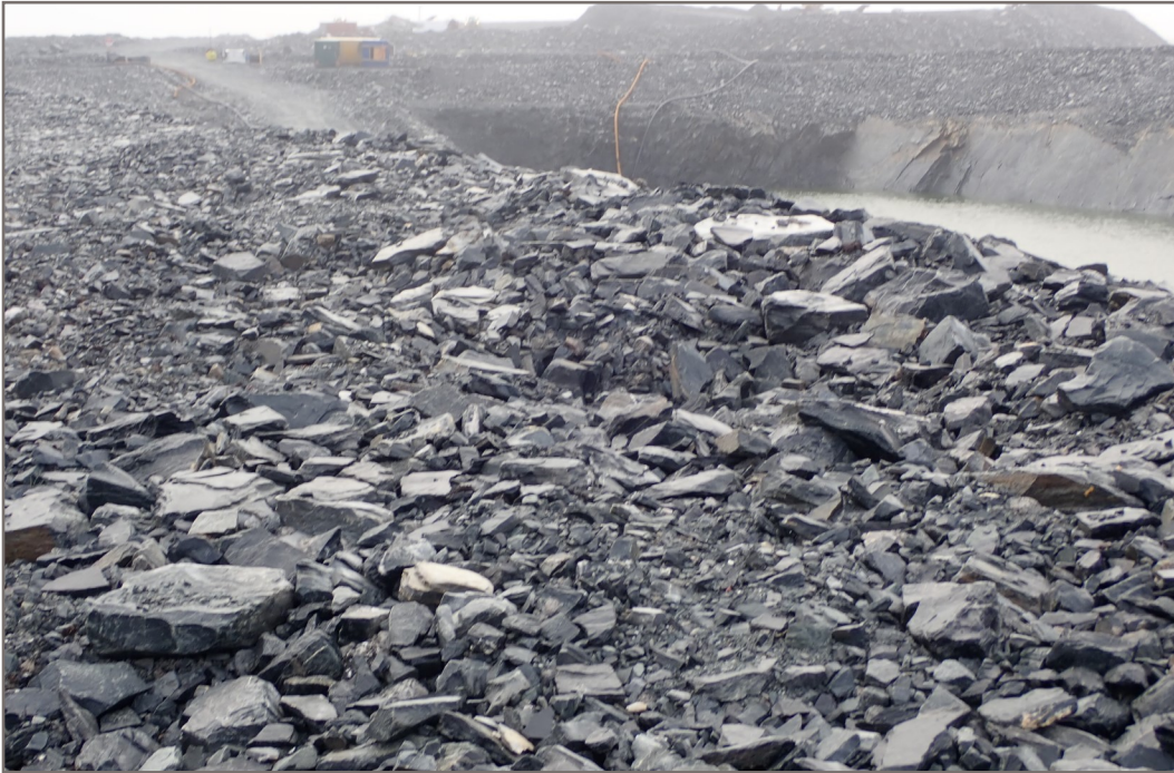
Photo 17: SP4 Saline Pond —Settlement in rockfill covering overburden slope.
