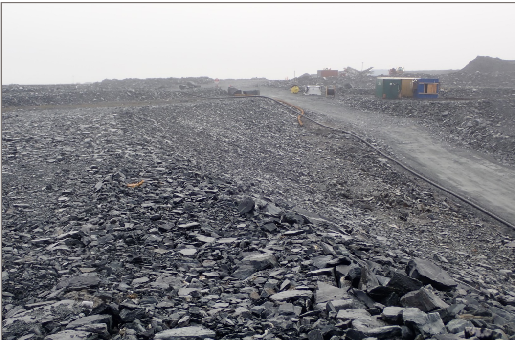
Photo 14: SP4—Rockfill covered overburden slope.
