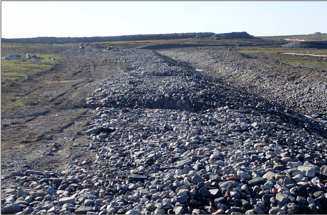
Photo 7: Channel 4 - Subsidence in rip rap—in upstream slope (east) slope of the channel.
