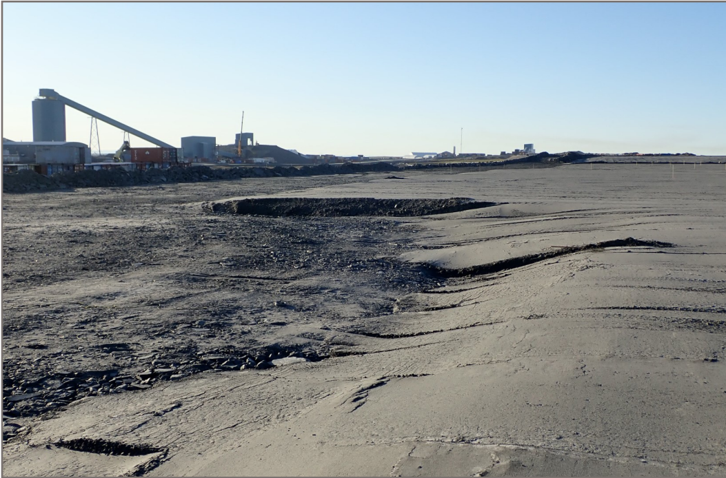
Photo 1: TSF - Tailing surface, northeast side, compacted, approximately 300 mm lift thickness
