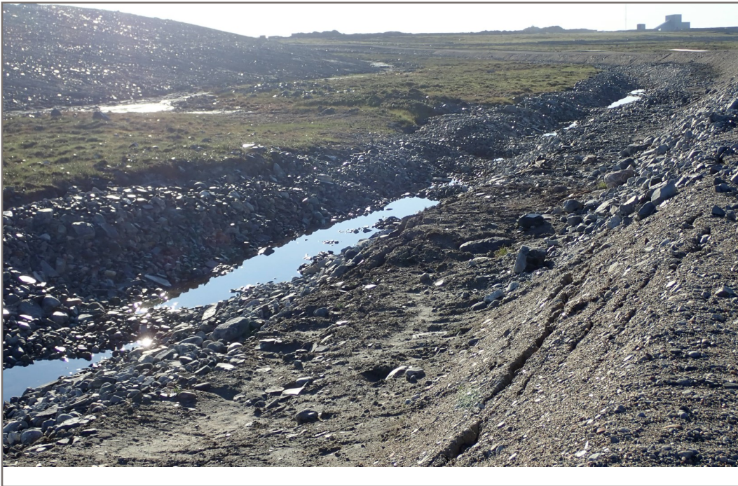
Photo 12: Channel 3 - Ponding in channel; appears to be some subsidence in base of channel resulting in rip settling and cracking in road side slope.
