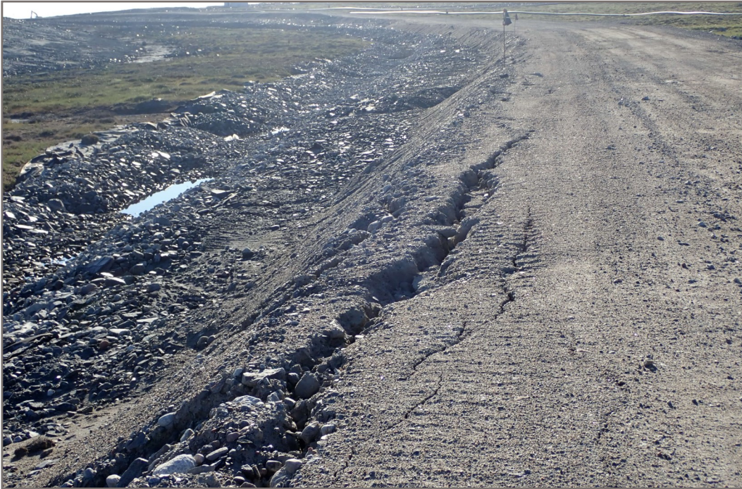
Photo 15: Channel 3 - Cracking in road side slopes.
