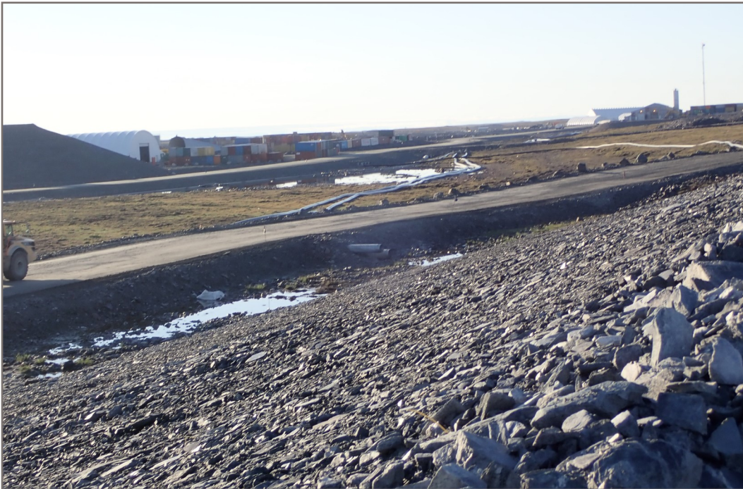
Photo 12: TSF - Rockfill covered TSF slope
