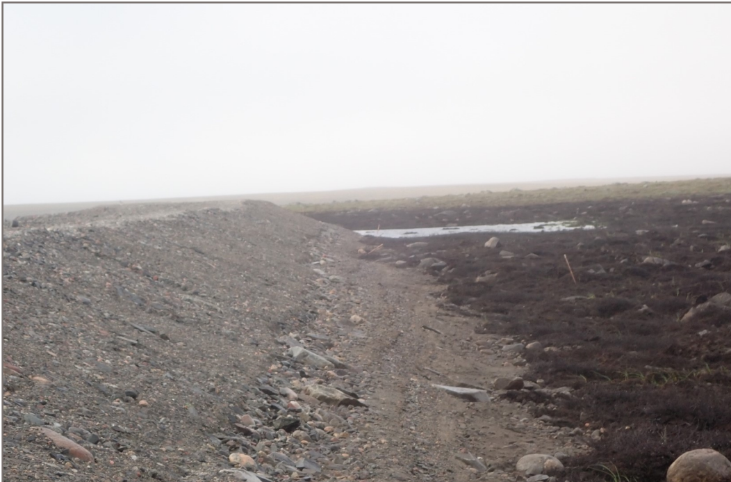
Photo 26: Channel 2—Minor surface erosion along berm from ponded water.
