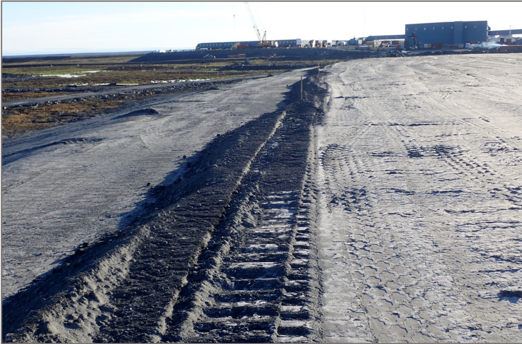
Photo 7: TSF - Slope between Cell 1 and future Cell 2. White precipitate on portions of the tailings surface.
