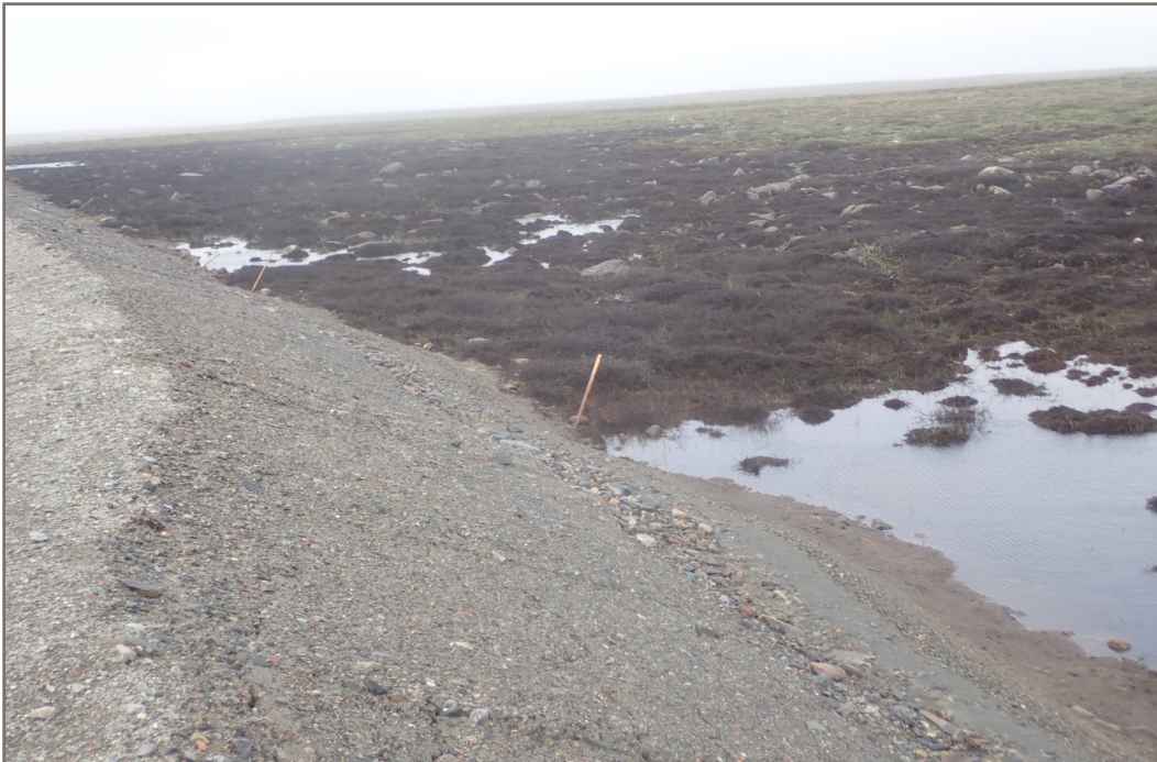
Photo 24: Berm 2—Ponded water upstream of Berm 2—Wave wash zone indication of higher water level.
