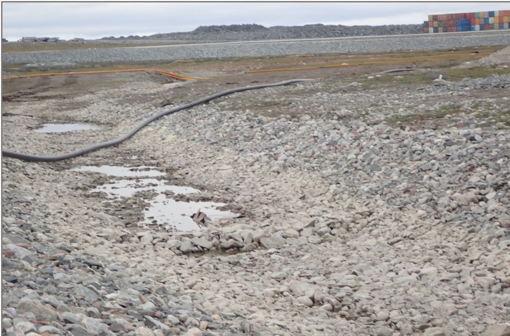
Photo 20: Channel 5—Settlement and ponding
