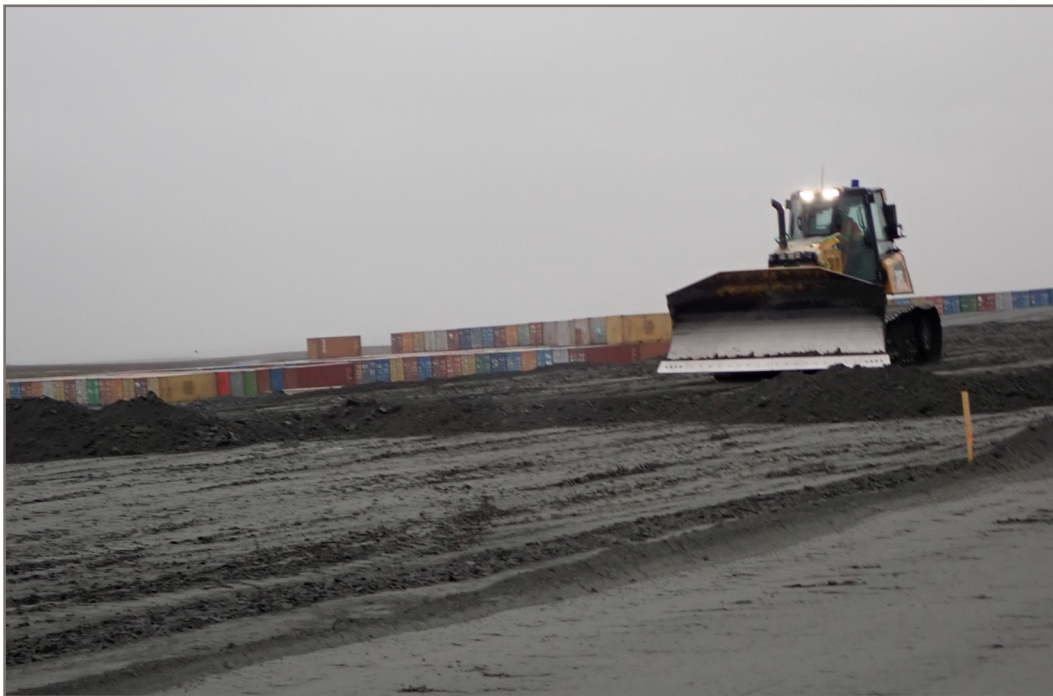
Photo 8: TSF - Spreading tailings, prior to compaction.
