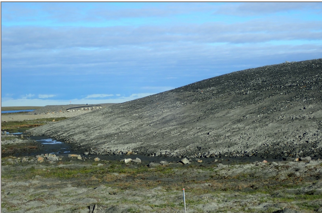
Photo 10: TSF - Rockfill covered slope of TSF. Some fine sediment at toe of slope, reported due to tailings contaminated snow placed in the area.
