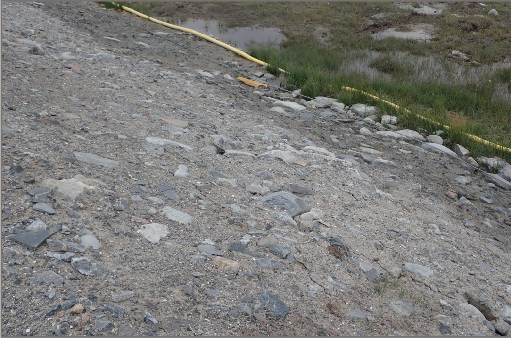
Photo 29: Berm 3—Minor cracking in berm.
