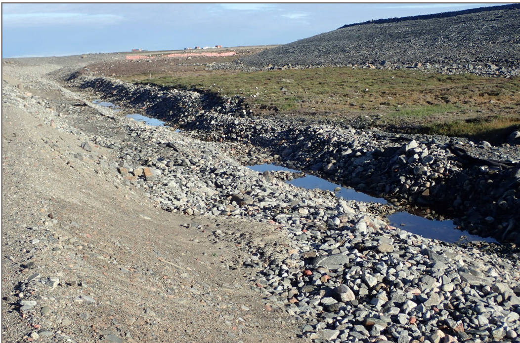
Photo 14: Channel 3 - Ponding in channel; appears to be some subsidence in base of channel resulting in rip settling and cracking in road side slope.. High points (less subsidence) resulting in ponding.
