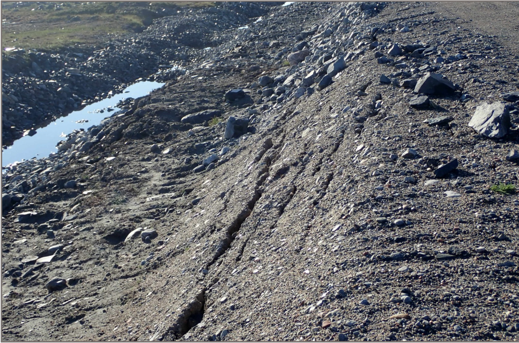
Photo 13: Channel 3 - Cracking in road side slope adjacent to channel.
