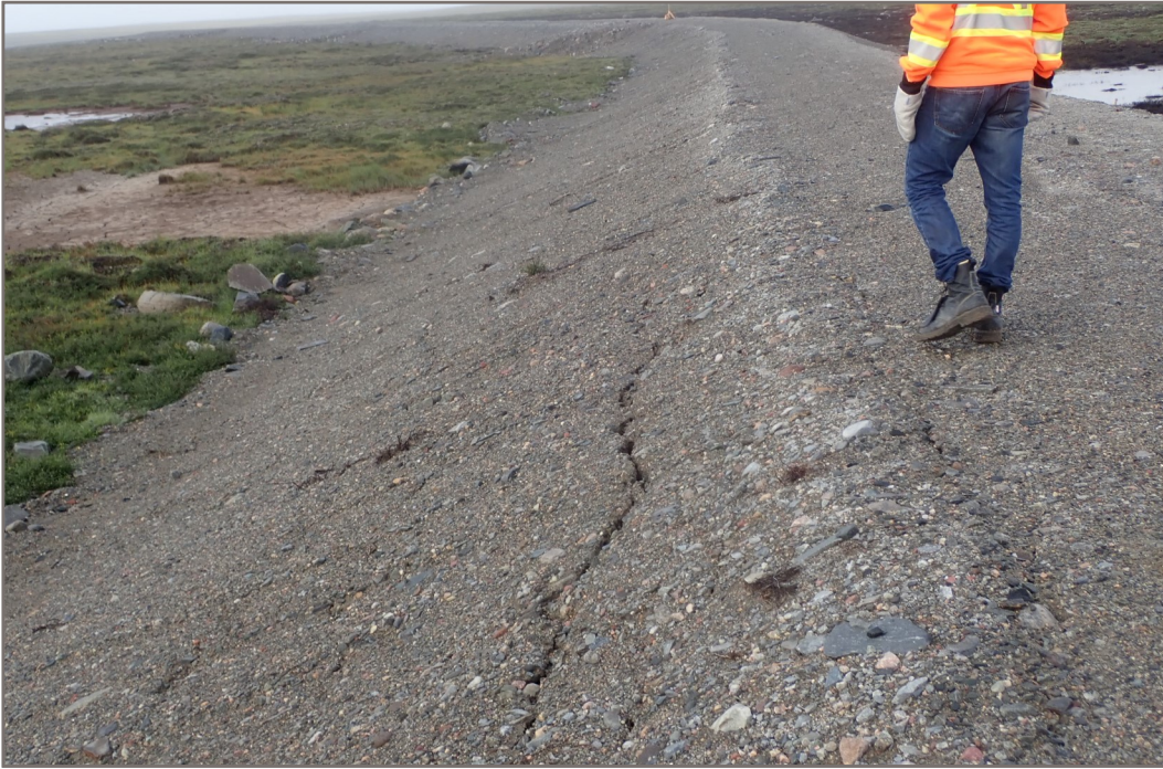
Photo 25: Berm 2—Cracking on side slope.
