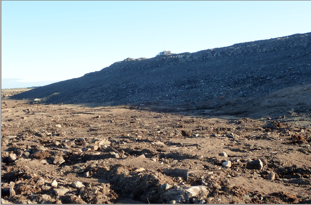
Photo 13: TSF - Rockfill covered TSF slope above CP3.
