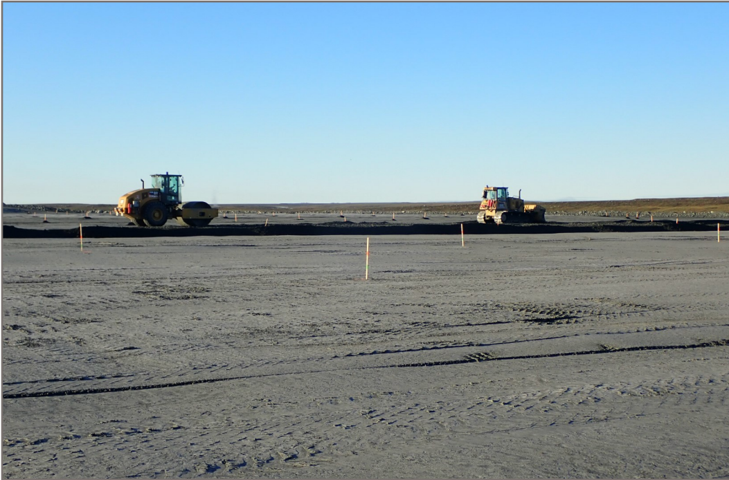
Photo 3: TSF - Placing and compacting tailings.
