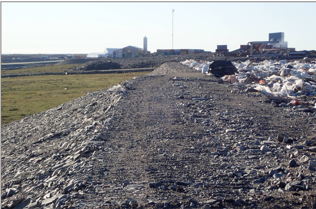
Photo 2: Landfill—East berm, waste close to crest.
