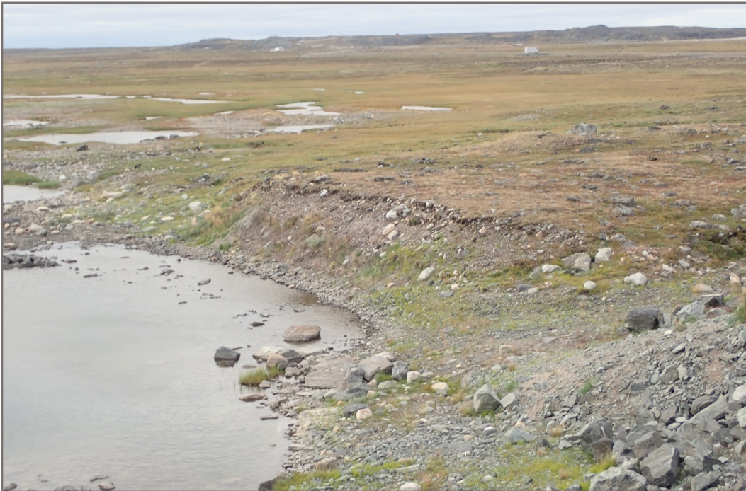
Photo 12: Meliadine River Bridge—Shoreline downstream of bridge—erodible sand and gravel deposit.
