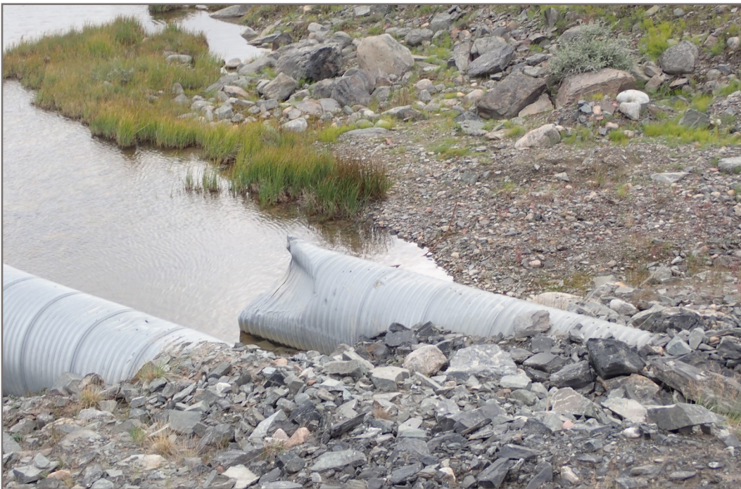
Photo 8: Culvert km 7.4—Damage to culvert inlet
