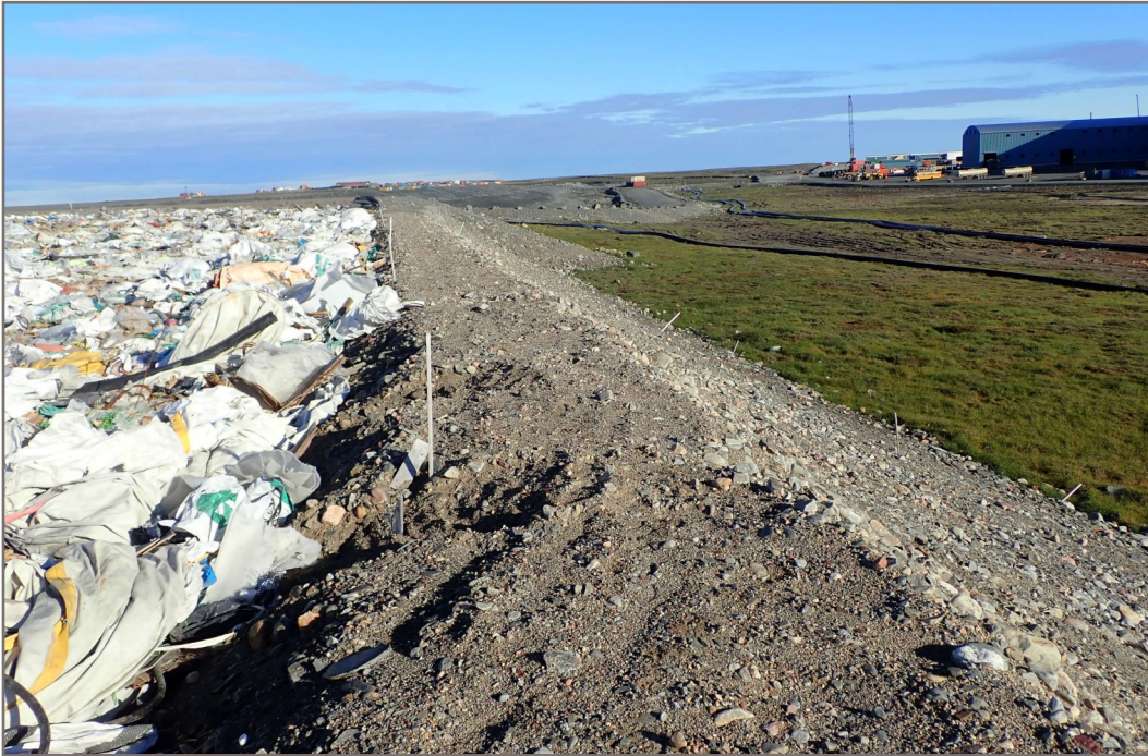
Photo 5: Landfill - West berm—esker fill.
