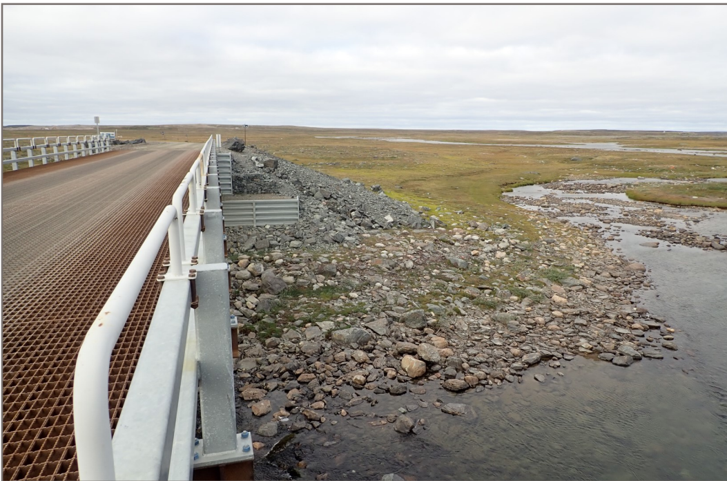
Photo 10: Meliadine River Bridge South Abutment
