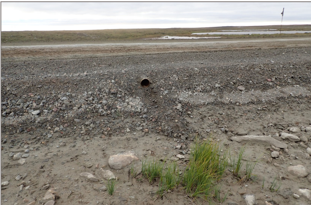
Photo 36: Culvert 26.8 - Lower culvert completely blocked with road fill.
