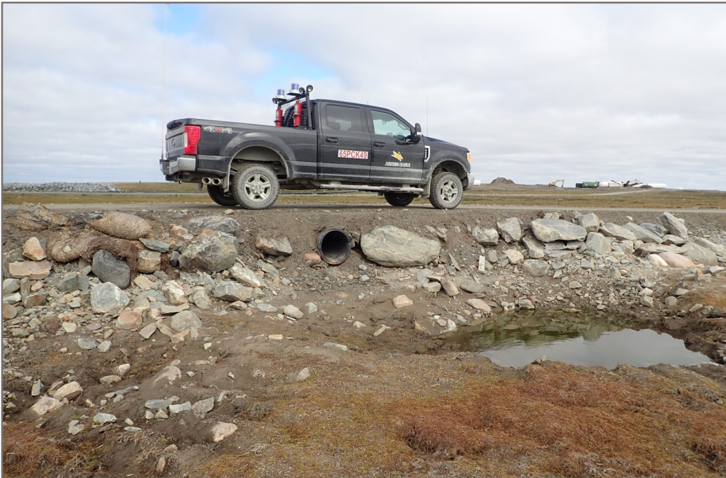
Photo 38: Culvert 29.6 - HDPE Culvert, inlet collapse approximately 25%.
