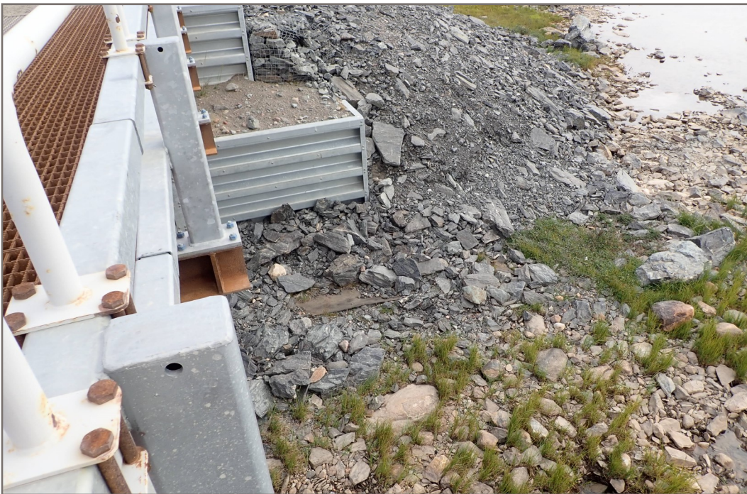
Photo 20: M-5 Bridge—Geotextile exposed at north abutment .
