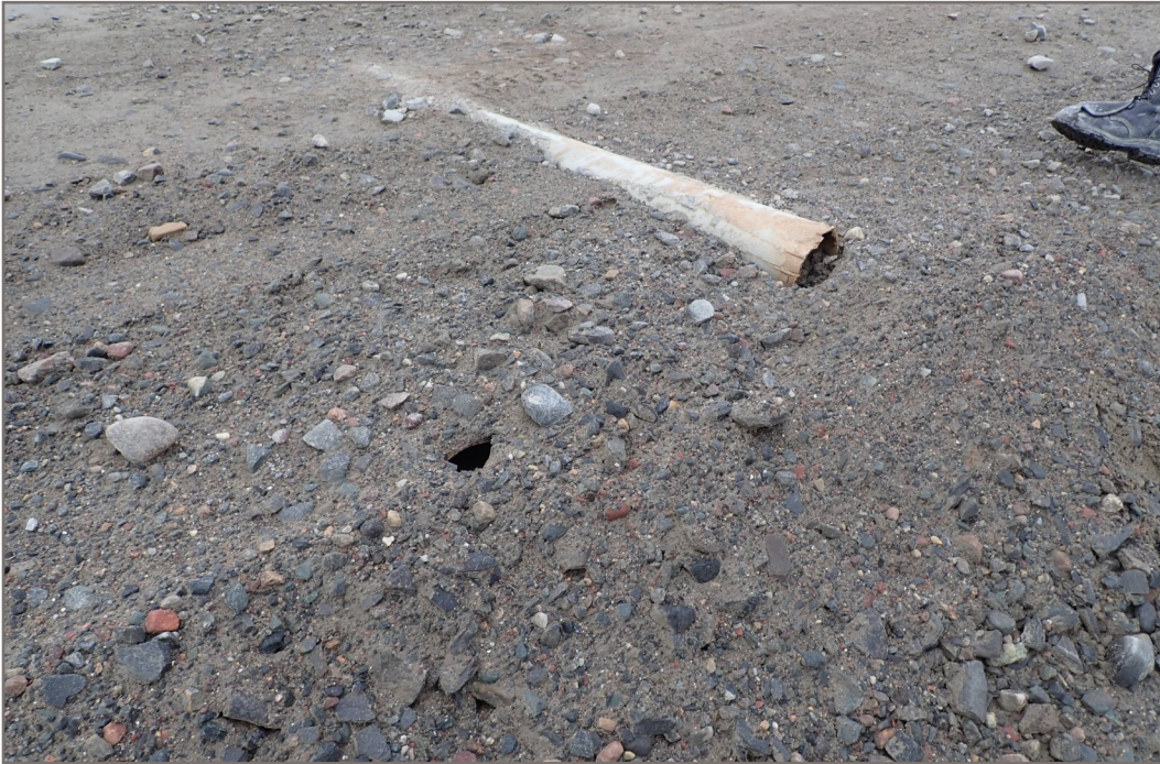
Photo 33: Culvert 26.2, Both inlets blocked with road fill.
