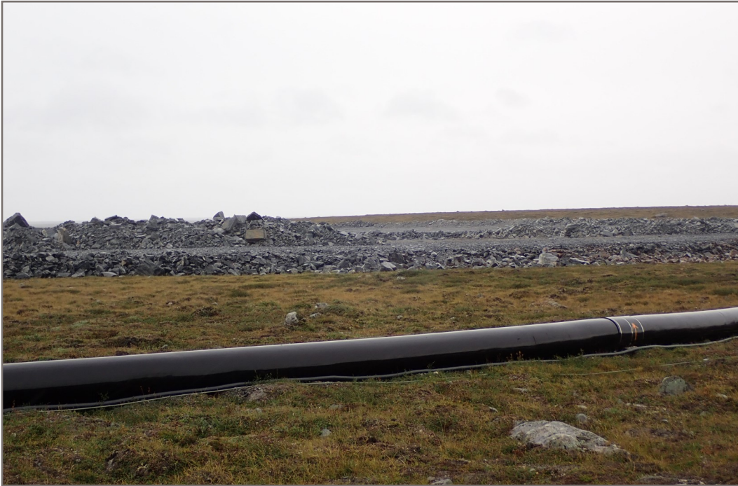
Photo 5: WRSF3—Initial lifts of waste rock in WRSF3
