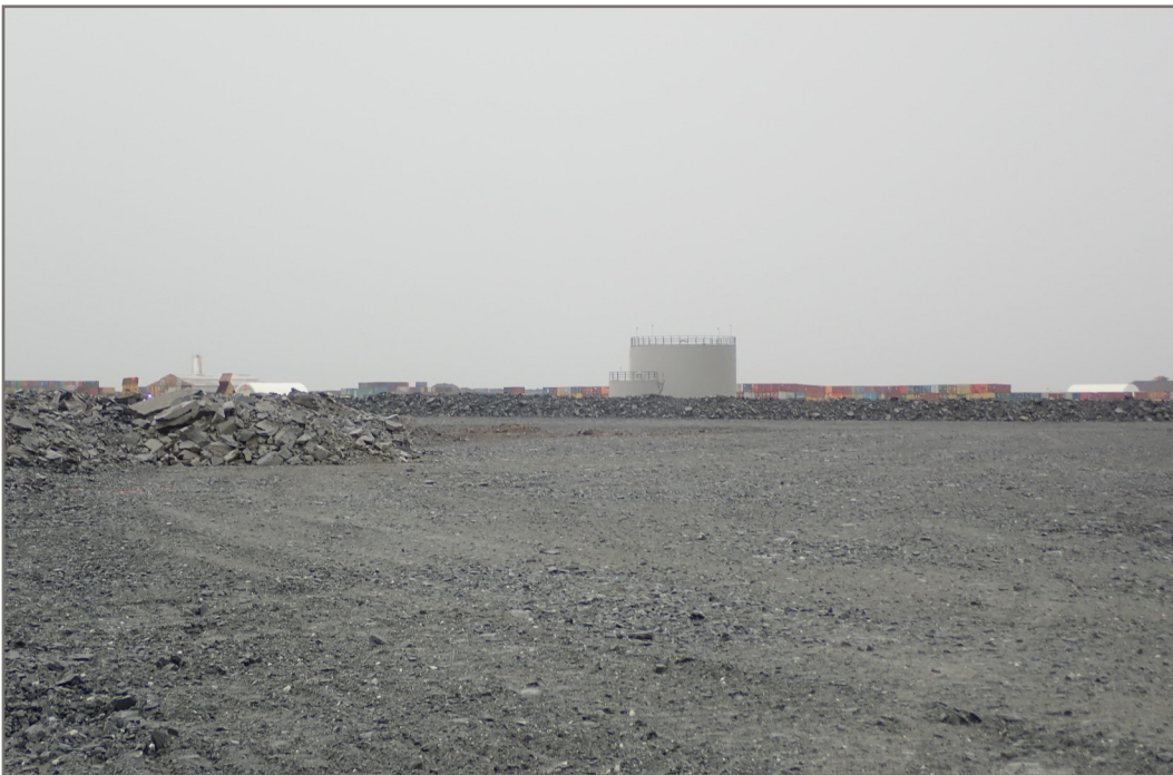
Photo 6: WRSF3—Initial lifts of waste rock in WRSF3—well spread, relatively tight structure
