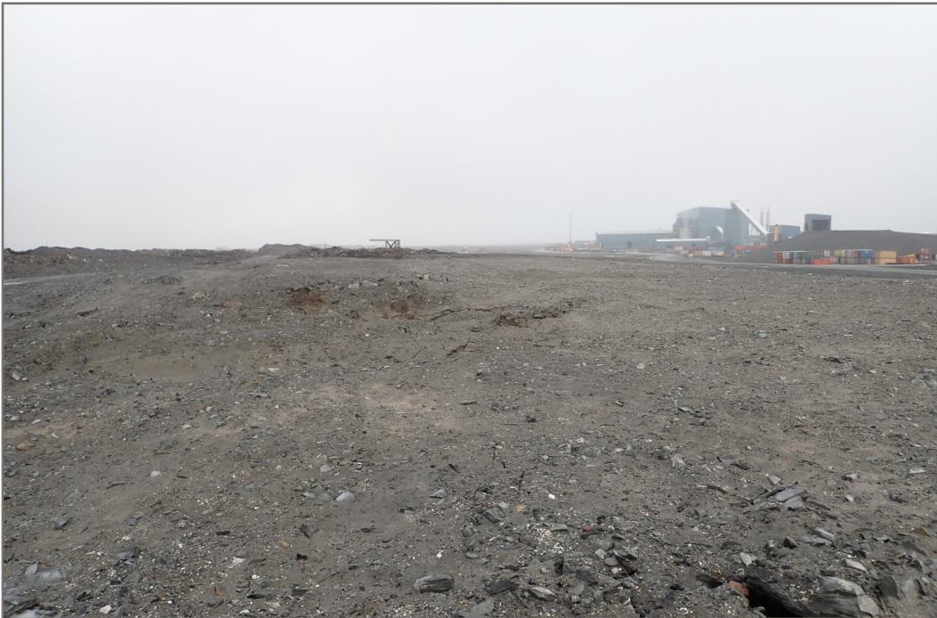
Photo 2: WRSF1 - Winter placed till—relatively wet, and settling.
