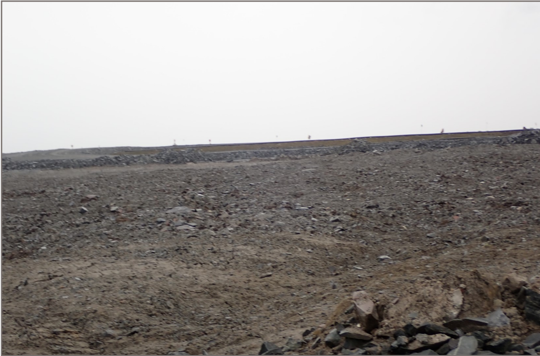
Photo 7: WRSF3—Initial lifts of till in WRSF3
