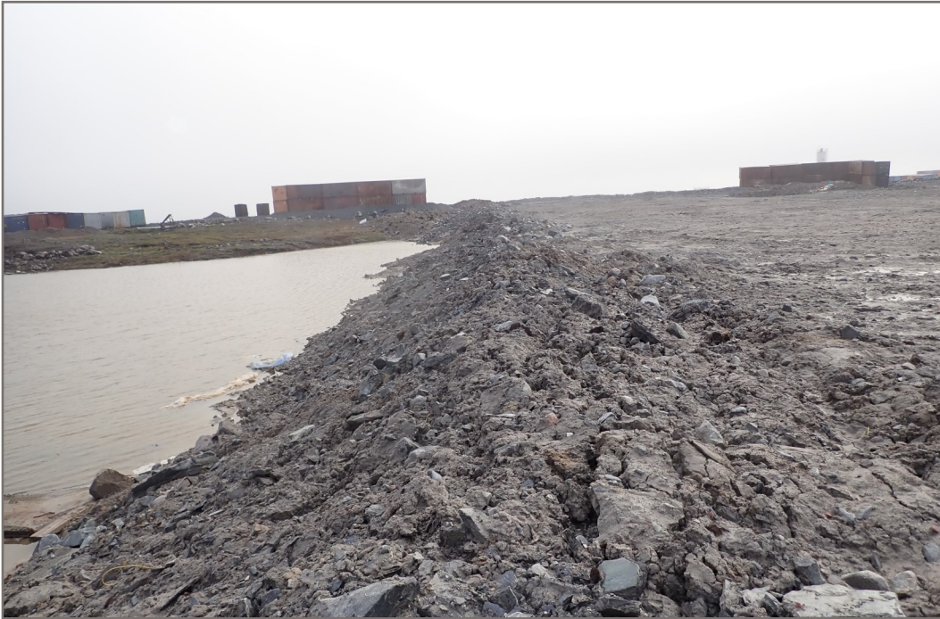
Photo 3: WRSF1—Winter placed till—wet and settling. Adjacent to small pond.
