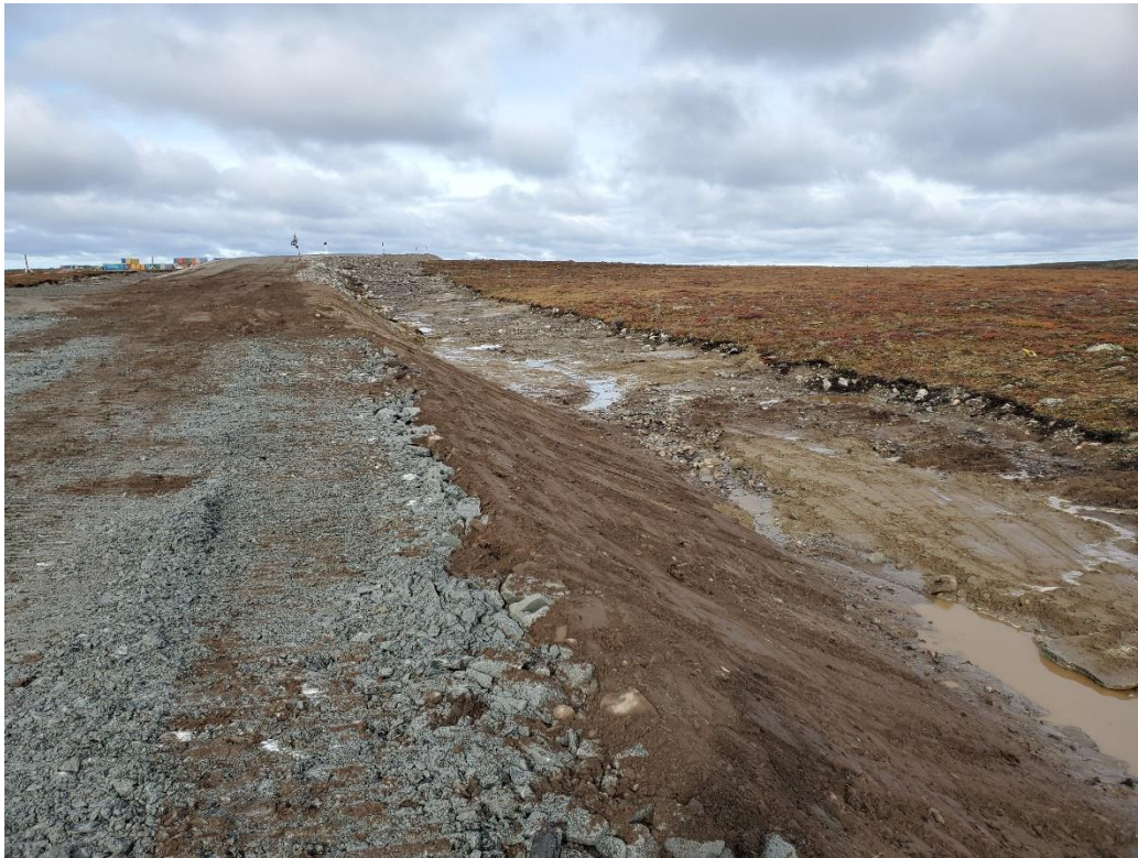
Figure 5: Road widened, and drainage channel restored.
