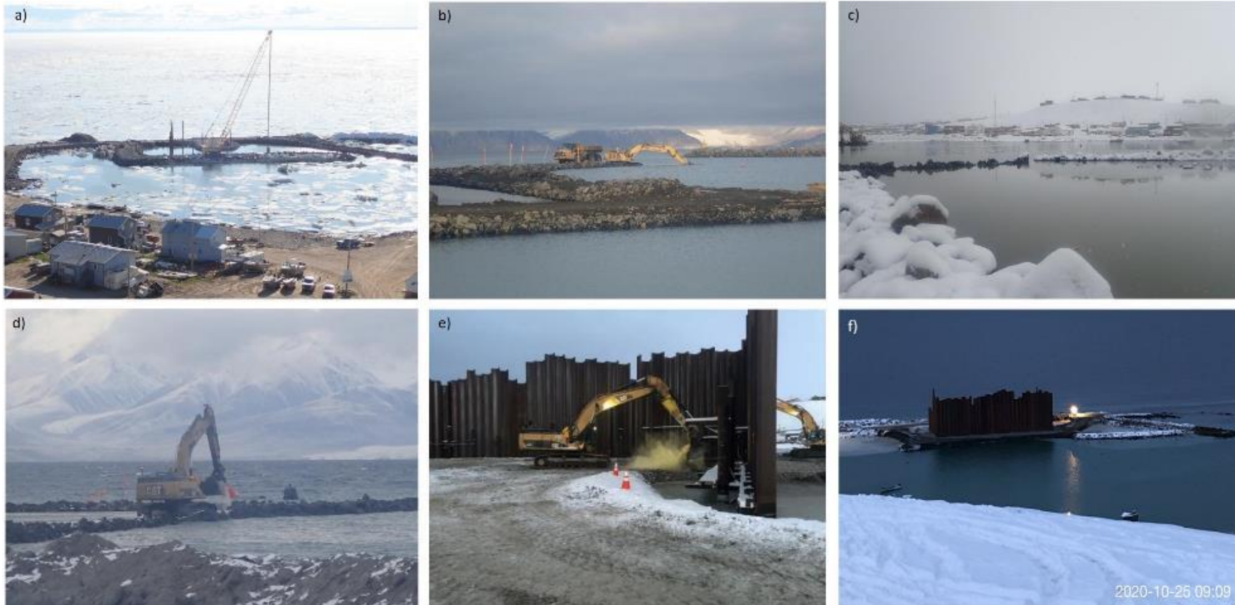
Photo 2-2 Development of Temporary Components – 2020 Construction Season: a) start of 2020 construction season, July 9 (Week 5); b) dredging causeway, September 30 (Week 17); c) water breaching the fixed wharf enclosure, October 3 (Week 17); d) subsequent elevation raise of enclosure, October 10 (Week 18); e) infill around fixed wharf, October 24 (Week 20); f) end of 2020 construction season, October 25 (Week 20)
