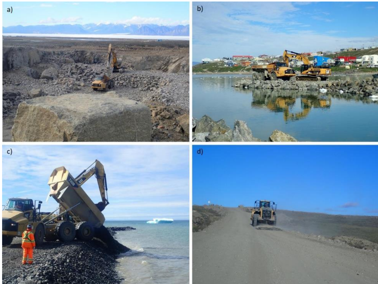
Photo 3-5 Representative Rock Truck Activity: a) rock truck loading in quarry, July 14 (Week 6); b) Unloading rock truck, July 18 (Week 6); c) unloading rock truck, July 31 (Week 8); d) front end loader maintaining haul road, August 3 (Week 9)
