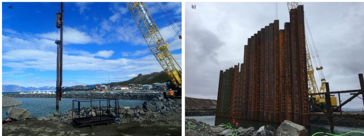
Photo 2-3 SCH - Representative Pile Driving Construction - 2020 Construction Season: a) Falsework Piles, July 8 (Week 5); b) Fixed Wharf, September 10 (Week 14)
