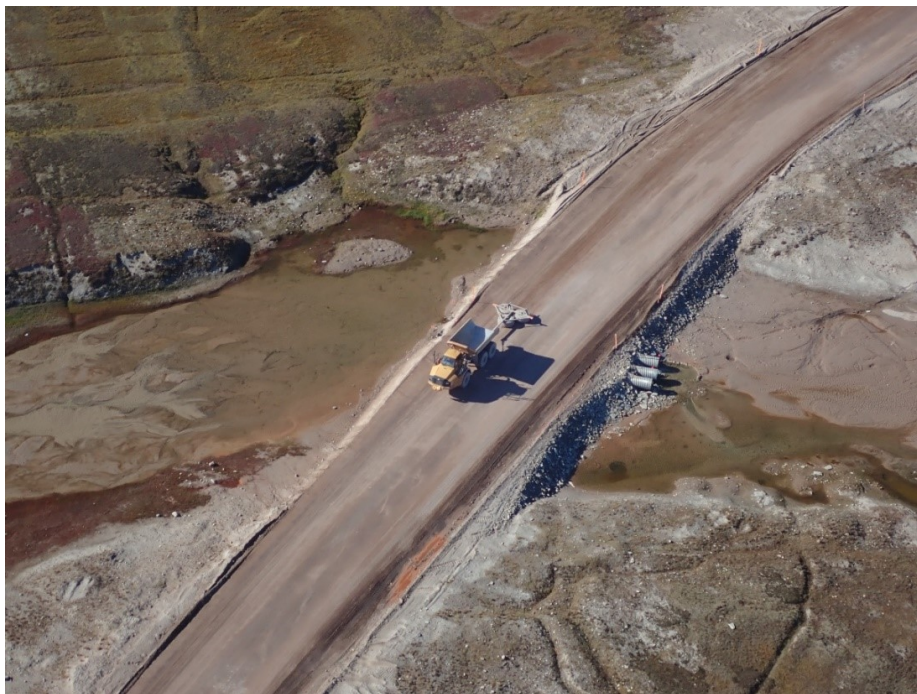
Photo 11 : Tire Drag for Dust Suppression – September 2020
