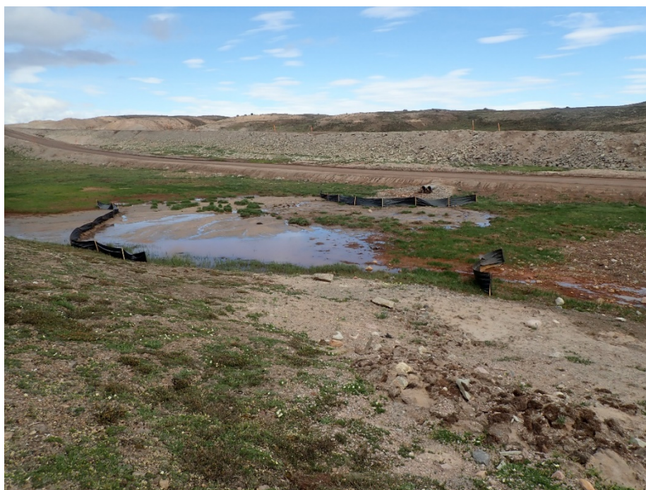
Photo 15 : Tote Road Sediment Control- July 2020
