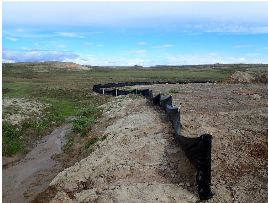
Photo 14: Silt Fence Installation around a Snow Stockpile – July 2020
