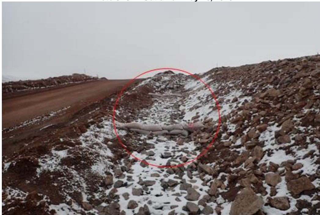
Photo 4: BG-01 Downstream Ditch with Sand Bags (May 18, 2020)
