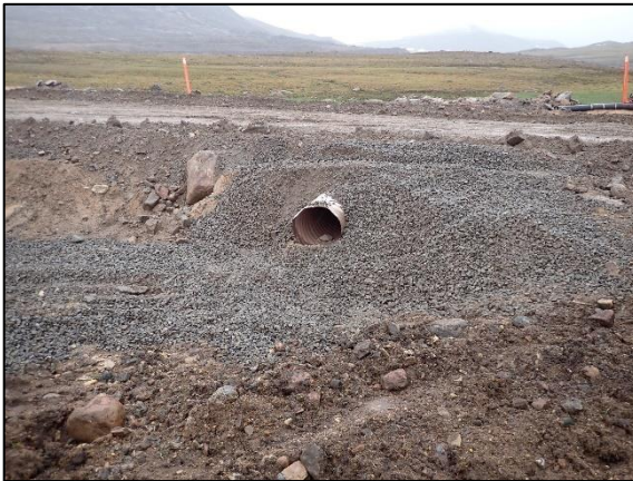
Photo 84: New Culvert by Effluent Discharge
