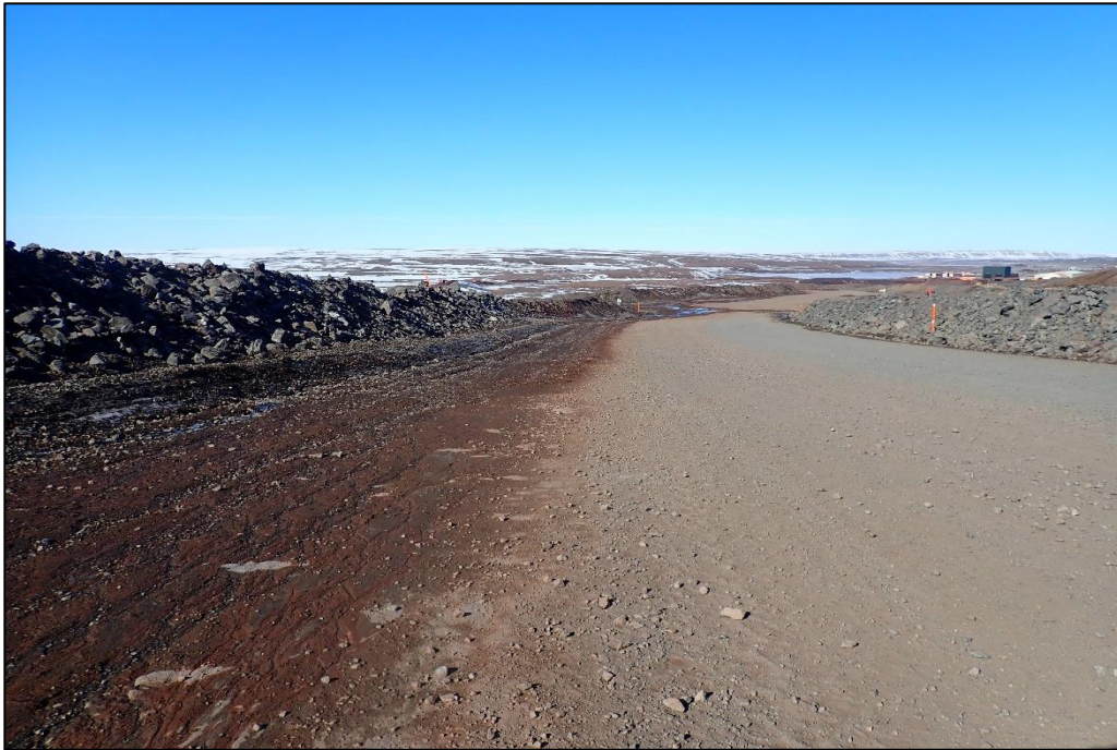
Photo 79: Mine Haul Road KM-106 to KM-107 following Lift Construction
