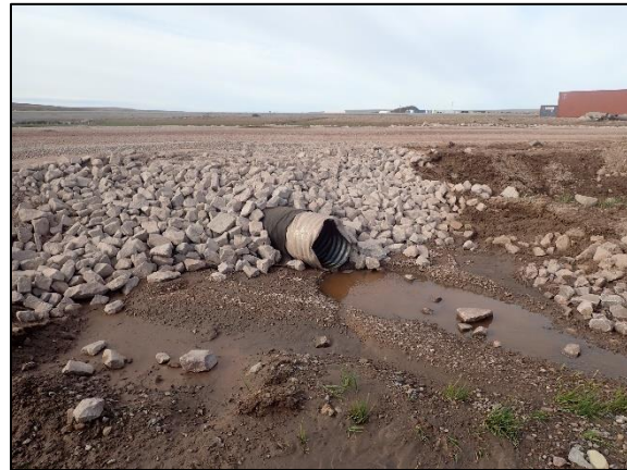
Photo 85: New culvert near Site Services Shop
