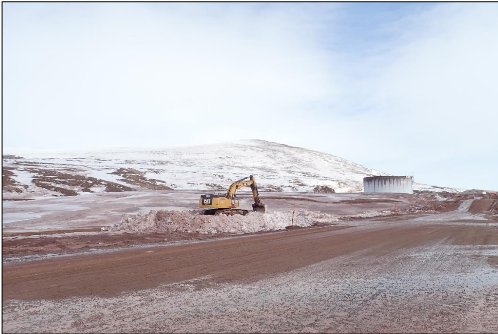
Photo 19: Snow Removal from a Culvert Across from Sailiivik Camp
