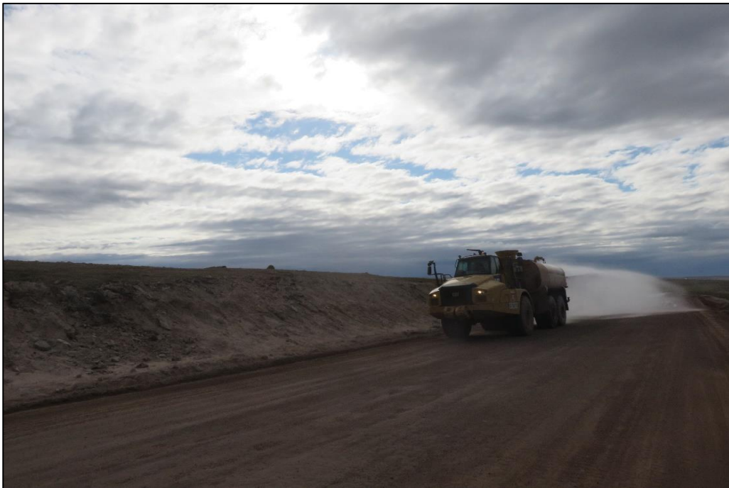
Photo 42: Truck Wetting the Tote Road for Dust Suppression
