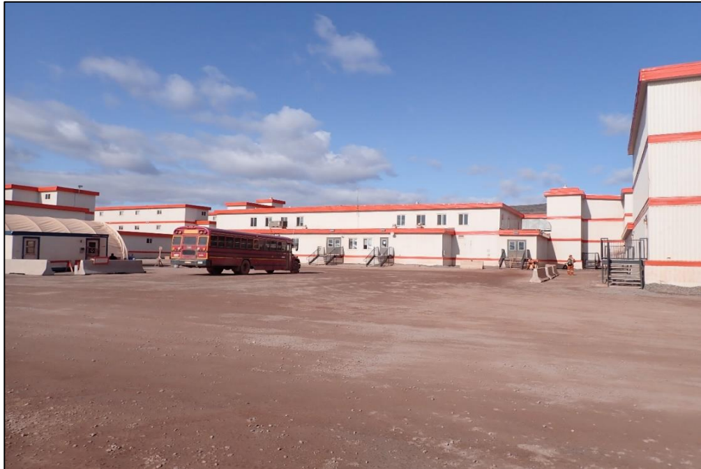
Photo 3: Sailiivik Accommodation Complex with Metal Skirting Around the Base
