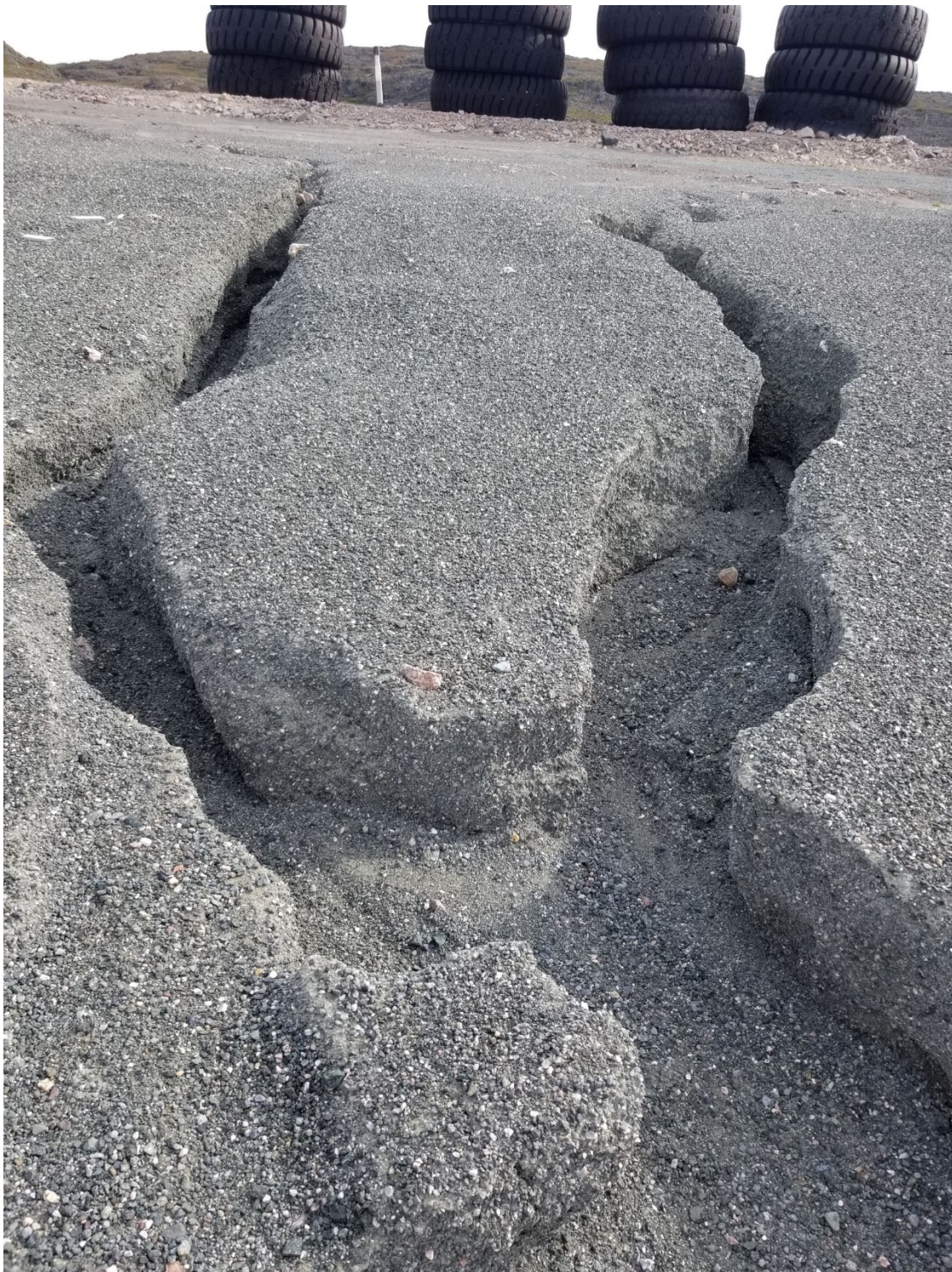
Photo 2: Erosion Channel in PKCA
