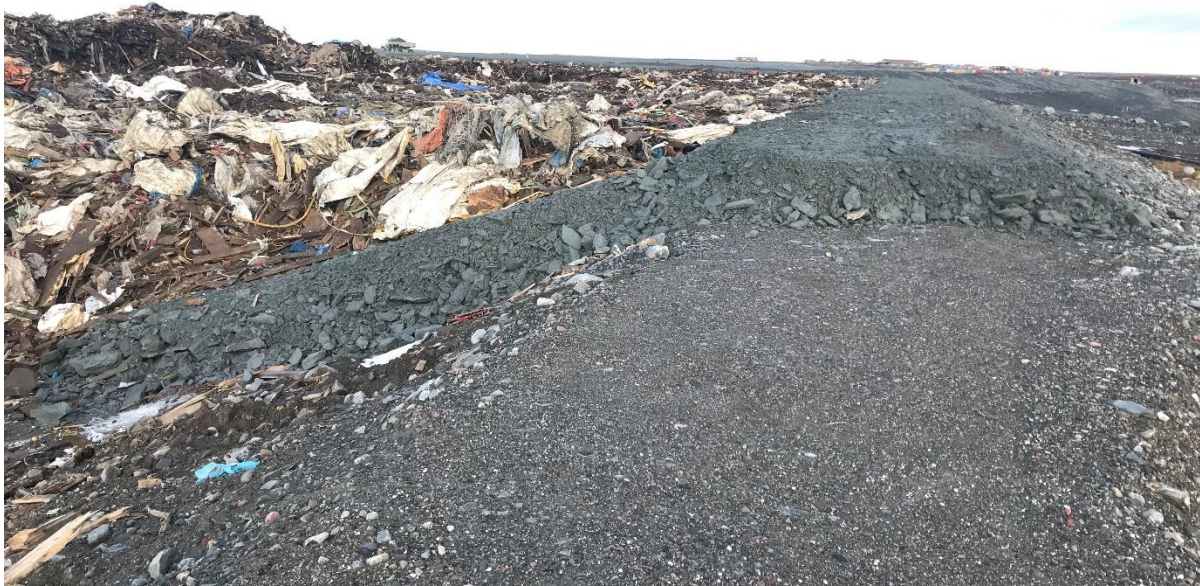
Photograph 3: Completed placement of fill with landfill waste placed back against the interior slope of the Stage 3 raise (Landfill Stage 3), September 19, 2020.
