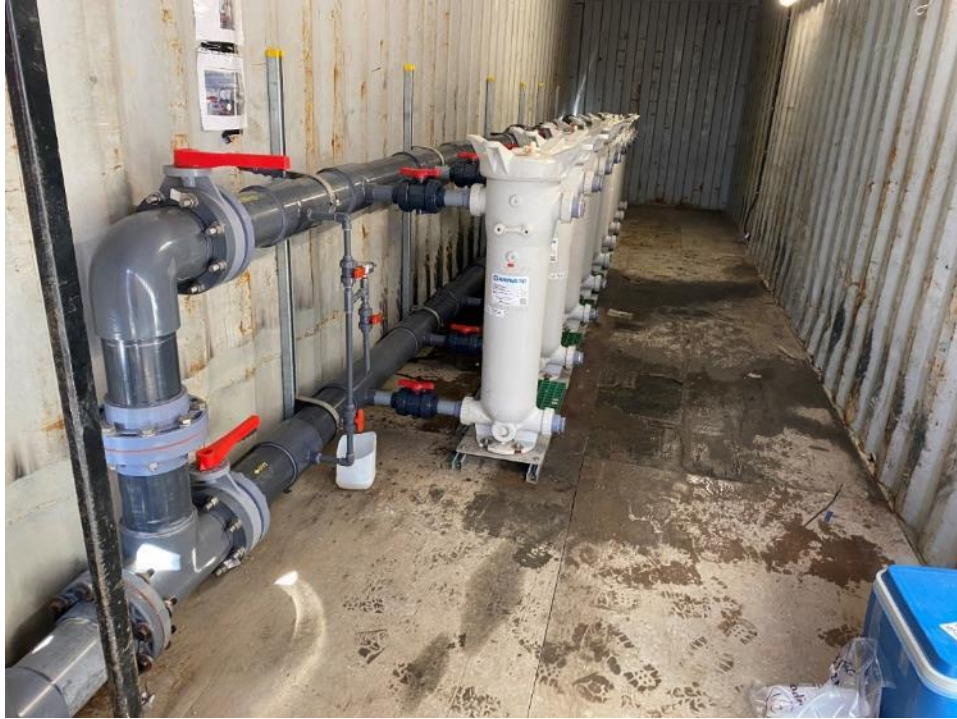
Photo 4: Saline Effluent Filtration Station Installed in 2021
