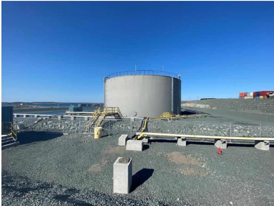
Photo 2: Fuel Farm 2 and Secondary Containment
