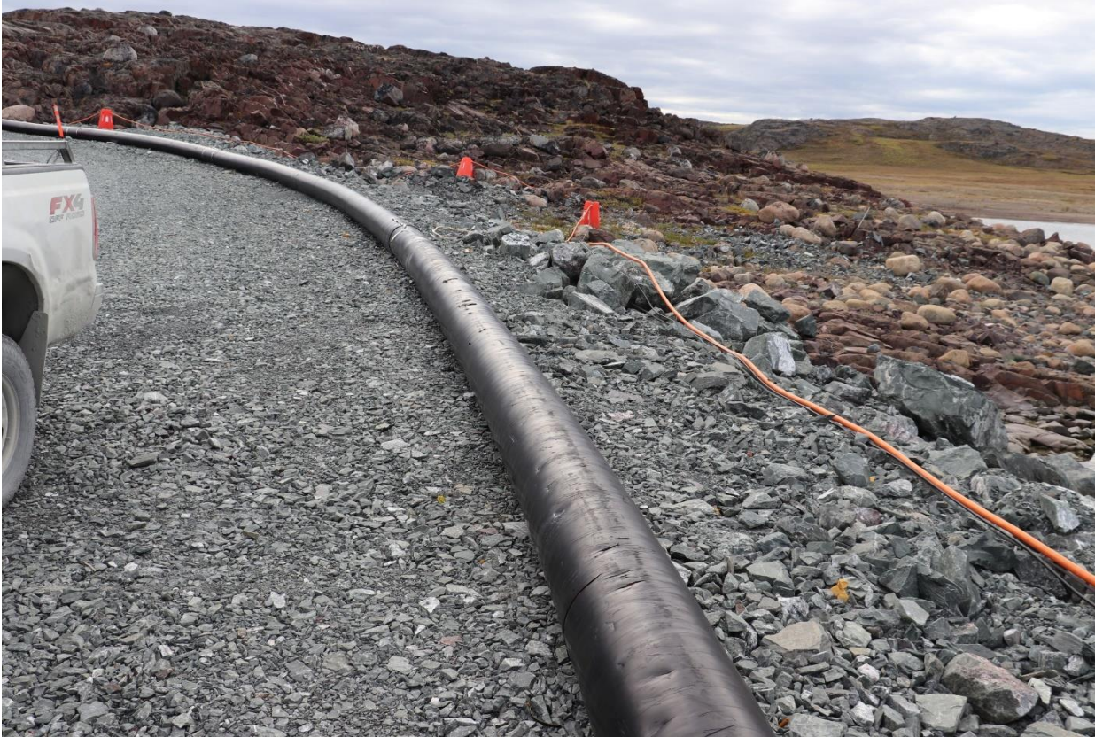
Photo 10: Damage to Saline Line from Vehicles
