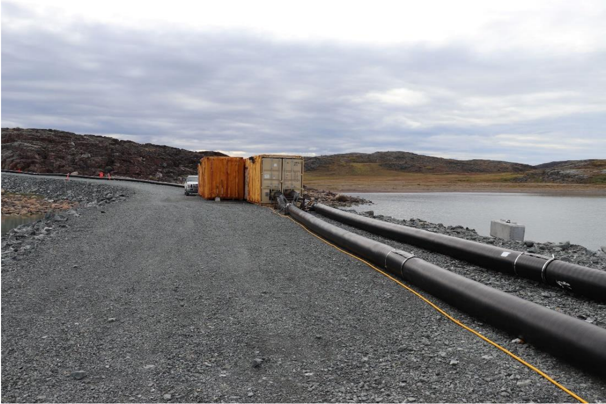
Photo 8: Saline Discharge Line and Water Recirculation Line
