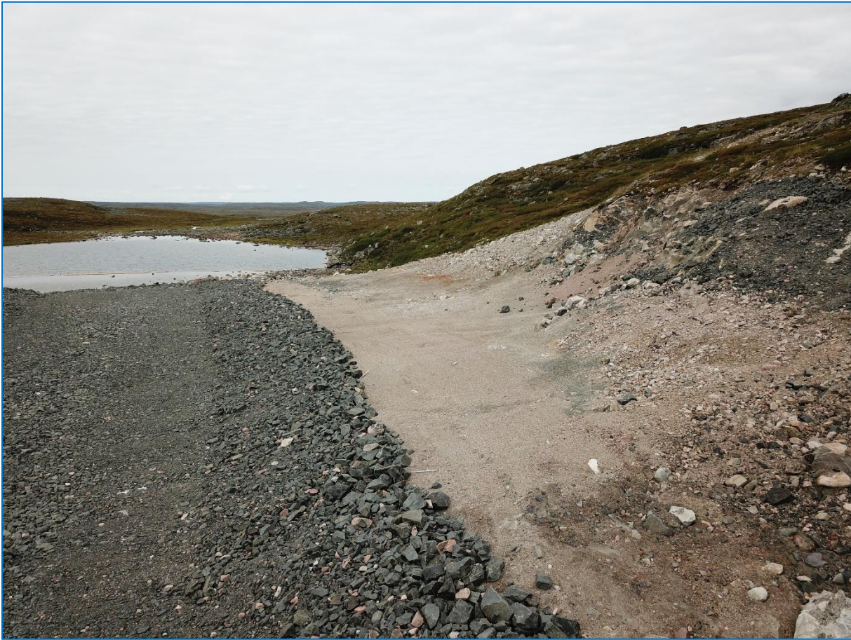
Photo 3: Aug. 17, 2021 West Dam Breach, Looking E – Erosion gully from North slope no longer observed.
