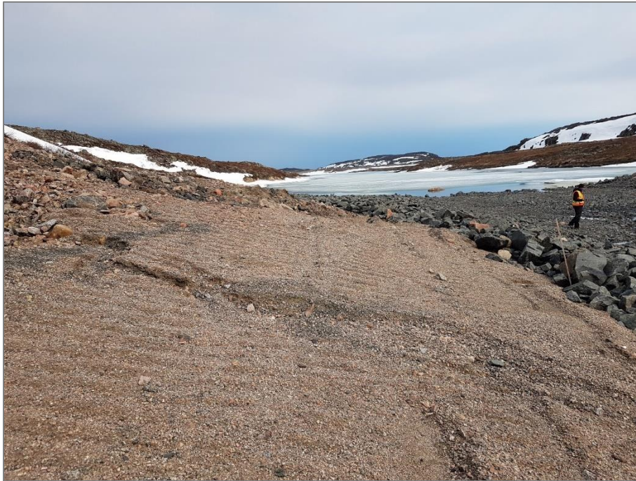
Photo 4: June 17, 2019 West Dam Breach – 2019 photo of erosion gully on North Bank.
