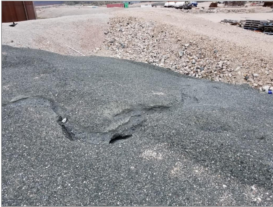
Photo 8: Sept 1, 2020 PHC Containment Cell Cover – 2020 photo of some minor drainage erosion in north corner of East Bank.
