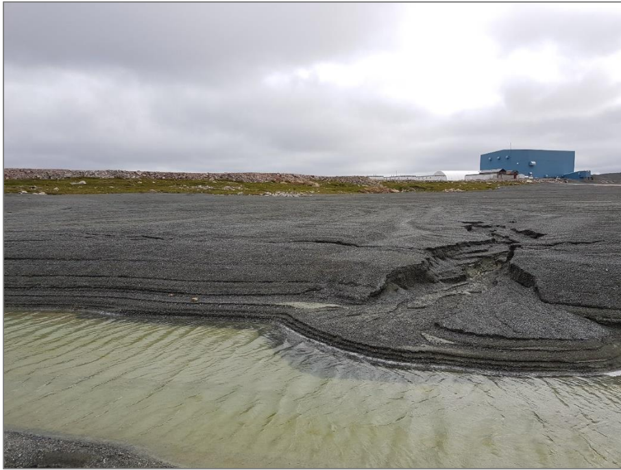
Photo 20: Aug. 3, 2018 PKCA Cover, North PKCA – 2018 photo of Outlet of Erosion Channel near ponded water adjacent Divider Dike A.
