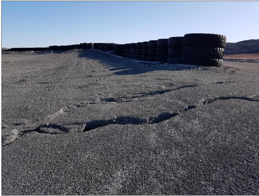
Photo 25: Sept. 11, 2019 PKCA Cover, East PKCA – 2019 photo of erosion from drainage into PKCA.
