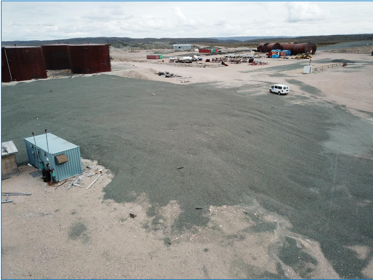
Photo 7: Aug. 17, 2021 PHC Containment Cell Cover, Looking NE – Erosion channels from previous years not observed.
