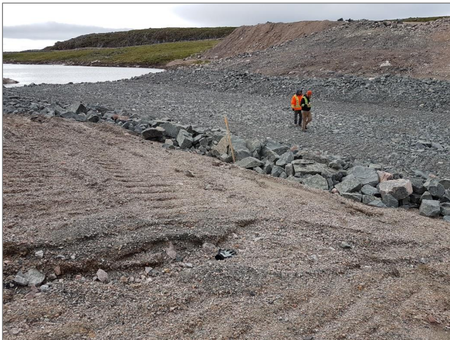
Photo 5: Aug. 3, 2018 West Dam Breach – 2018 photo of North Bank Erosion Gully.
