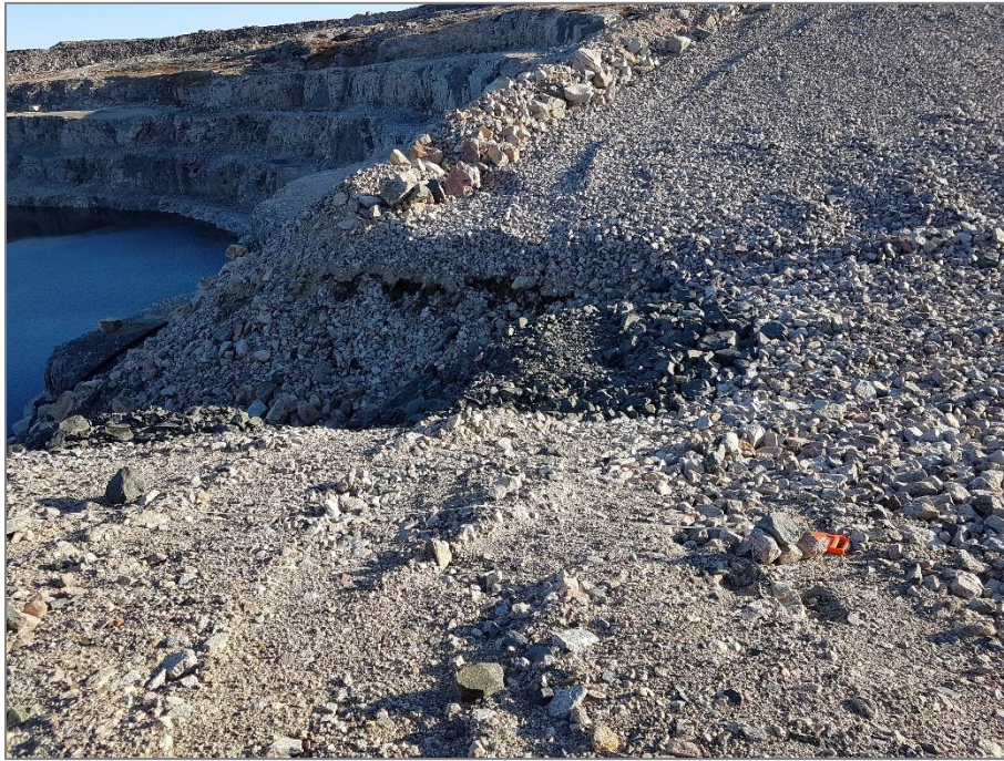
Photo 29: Sept. 10, 2019 C1 Channel, Looking E – 2019 photo of eroded section into Open Water @ 6.3 m in Fall.
