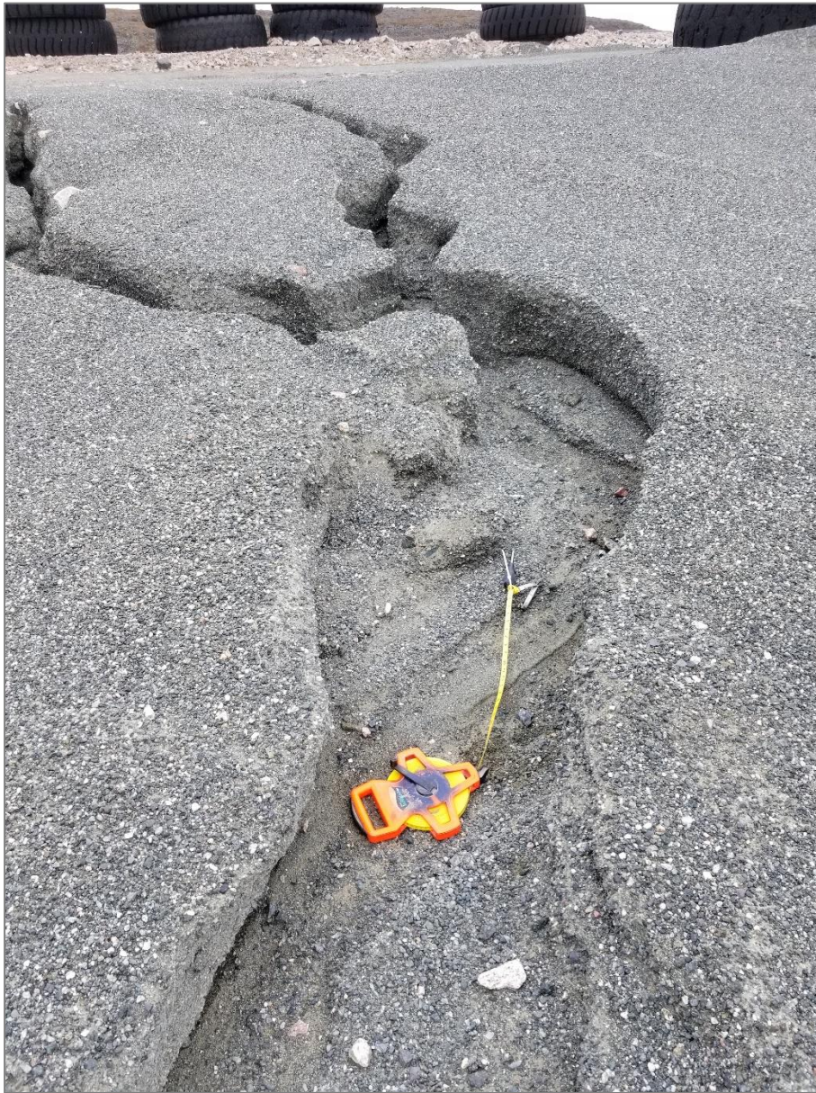
Photo 24: Sept. 1, 2020 PKCA Cover, East PKCA – 2020 photo of erosion from drainage into PKCA (some expansion from 2019).
