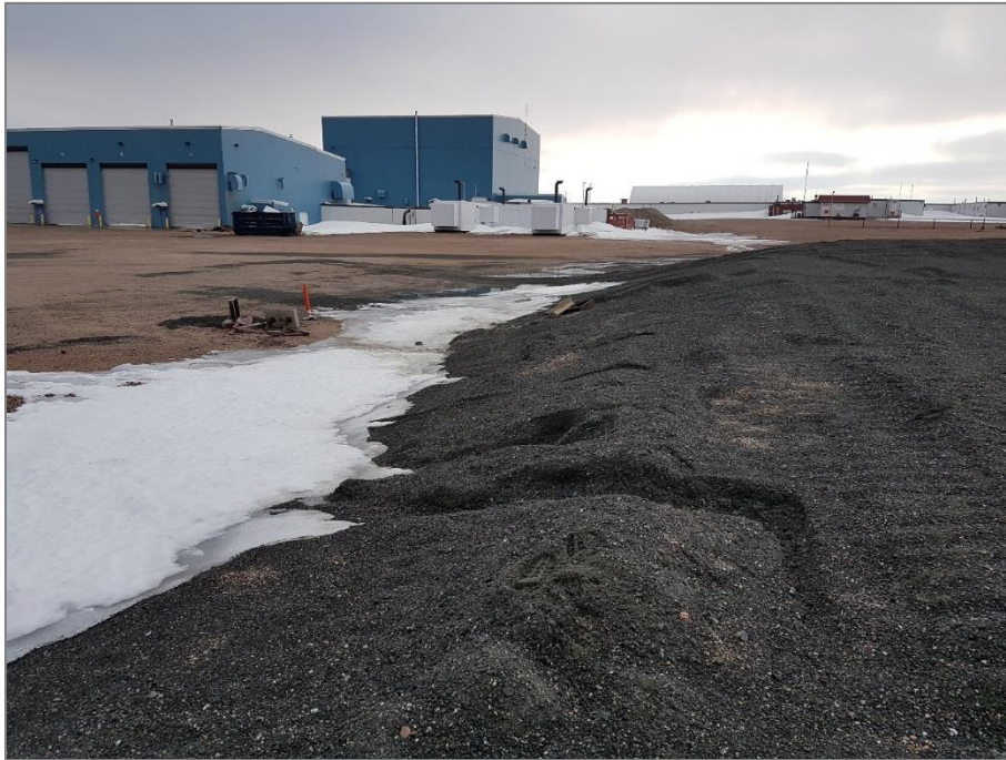
Photo 10: June 17, 2019 PHC Containment Cell Cover – 2019 photo looking S, drainage erosion on East Bank.
