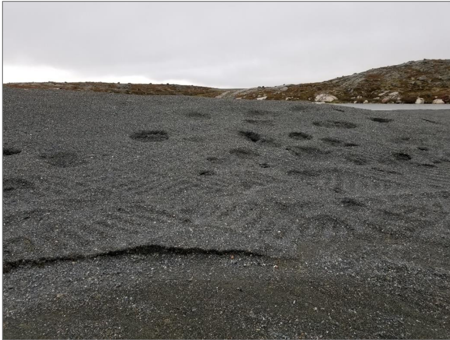
Photo 22: Sept. 1, 2020 PKCA Cover – 2020 photo of potholes (seasonally collapsed).
