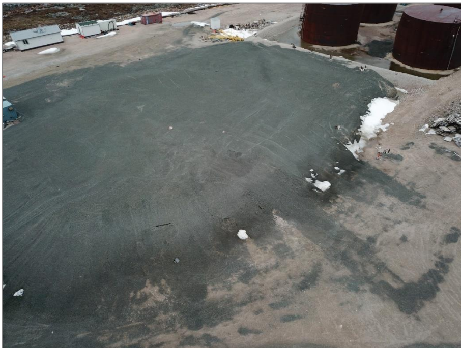
Photo 9: June 18, 2019 PHC Containment Cell Cover – 2019 photo looking N, some settlement and drainage erosion along East Bank.
