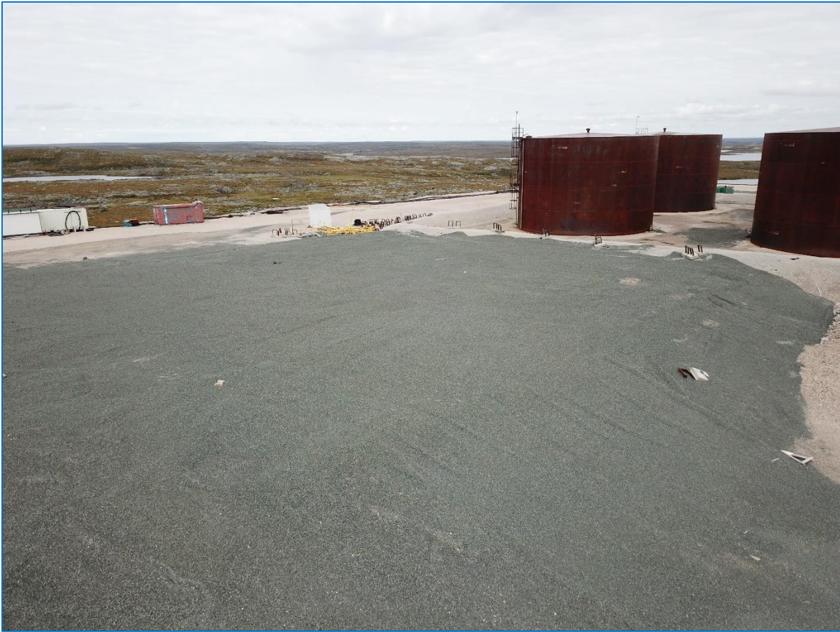
Photo 6: Aug. 17, 2021 PHC Containment Cell Cover, Looking N (to airstrip) – Protection soil cover in good condition.
