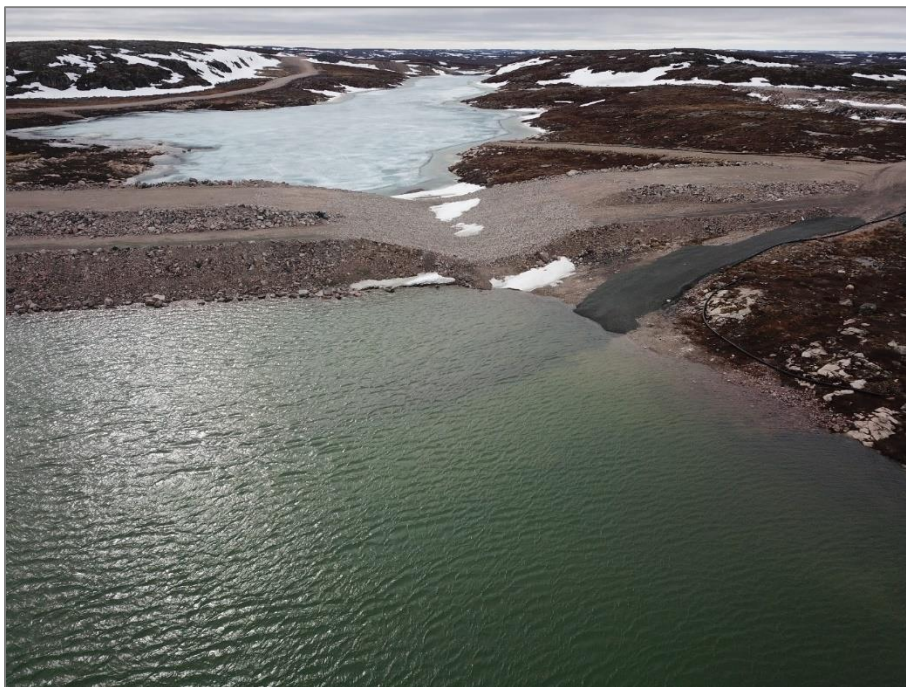
Photo 19: June 18, 2019 PKCA Cover – 2019 photo looking W, ponded water covering access road.
