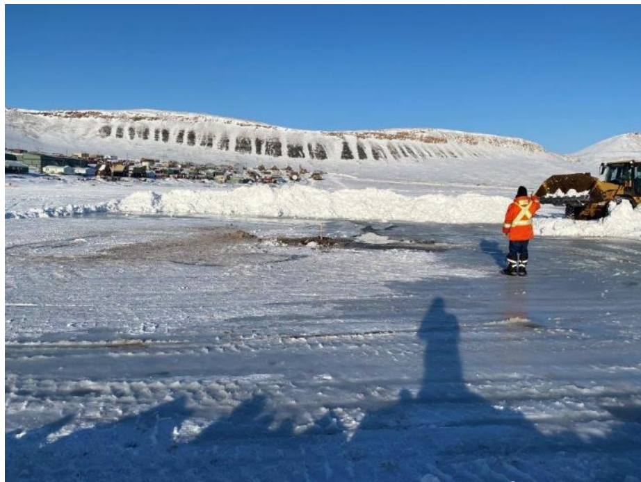
Photo 9 Loader placing snow back on ice after completion of BH21-0, March 29, 2021
