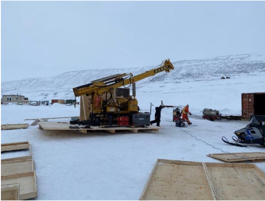
Photo 3 Floor of drill shack constructed. March 26, 2021
