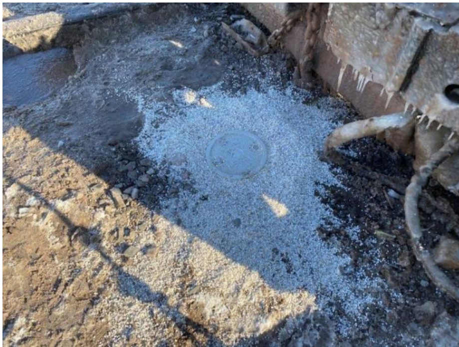
Photo 16 Monitoring well installation complete at BH/MW21-10, April 8, 2021
