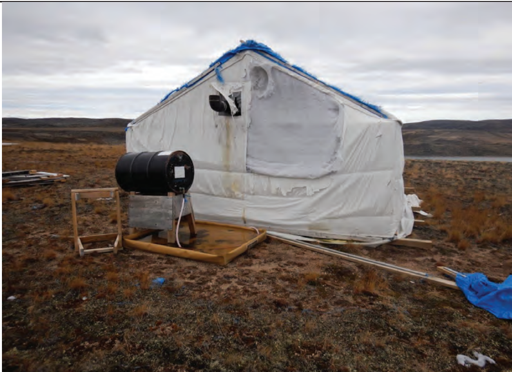
Description: heating stove tank without required covering.
