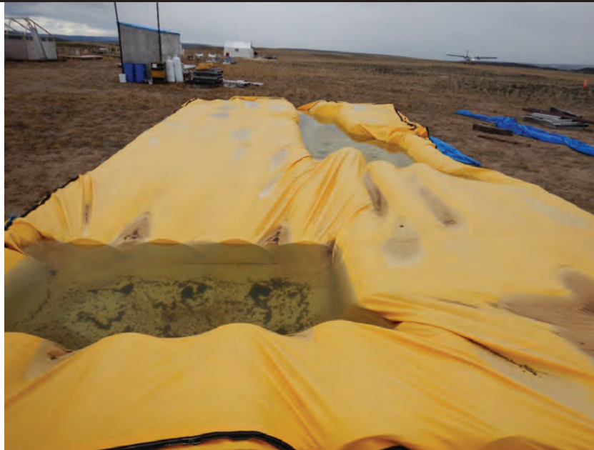
Description: pooling water on top of containment.
