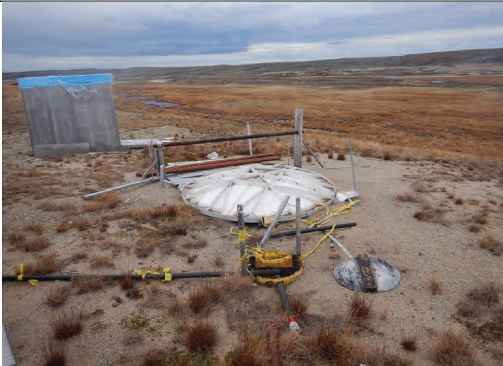
Description: sump without berms to prevent flooding.
