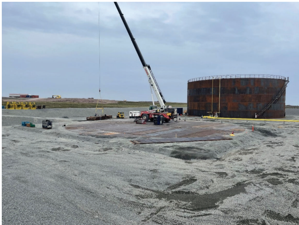
Tank floor construction
