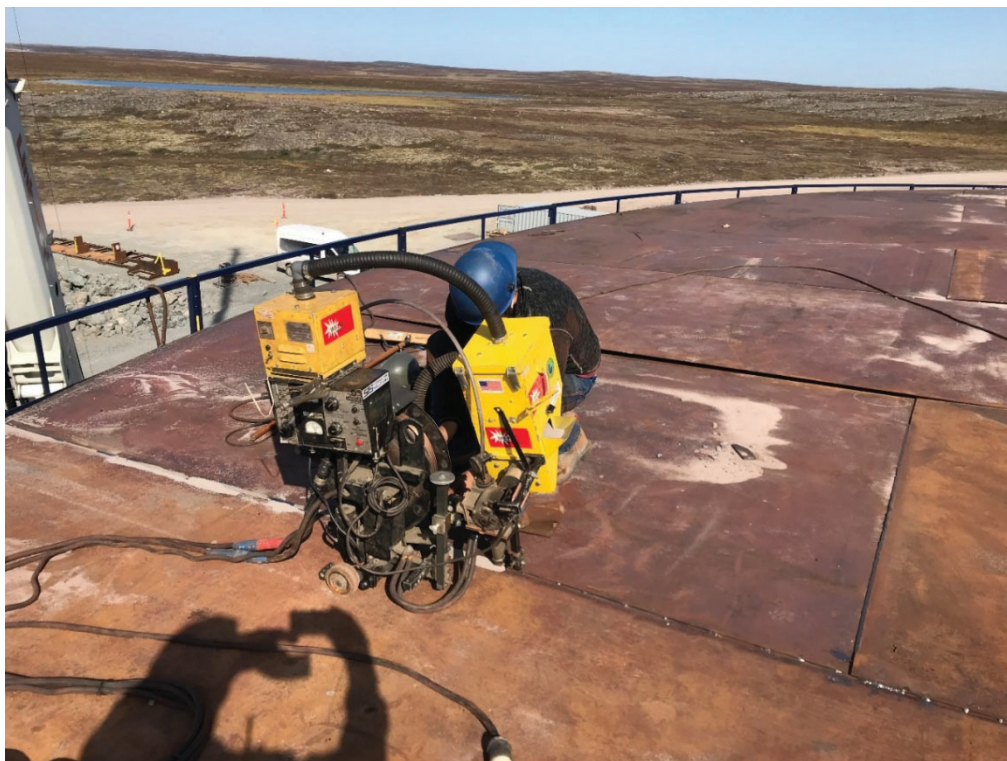
Tank roof plate welding
