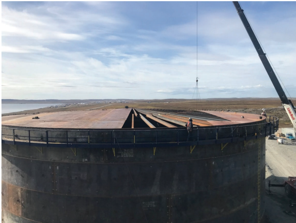
Tank roof structure
