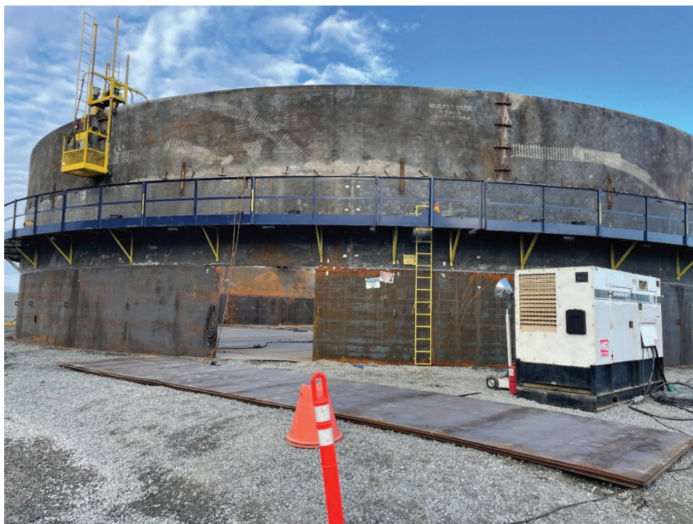
Tank wall third ring installation
